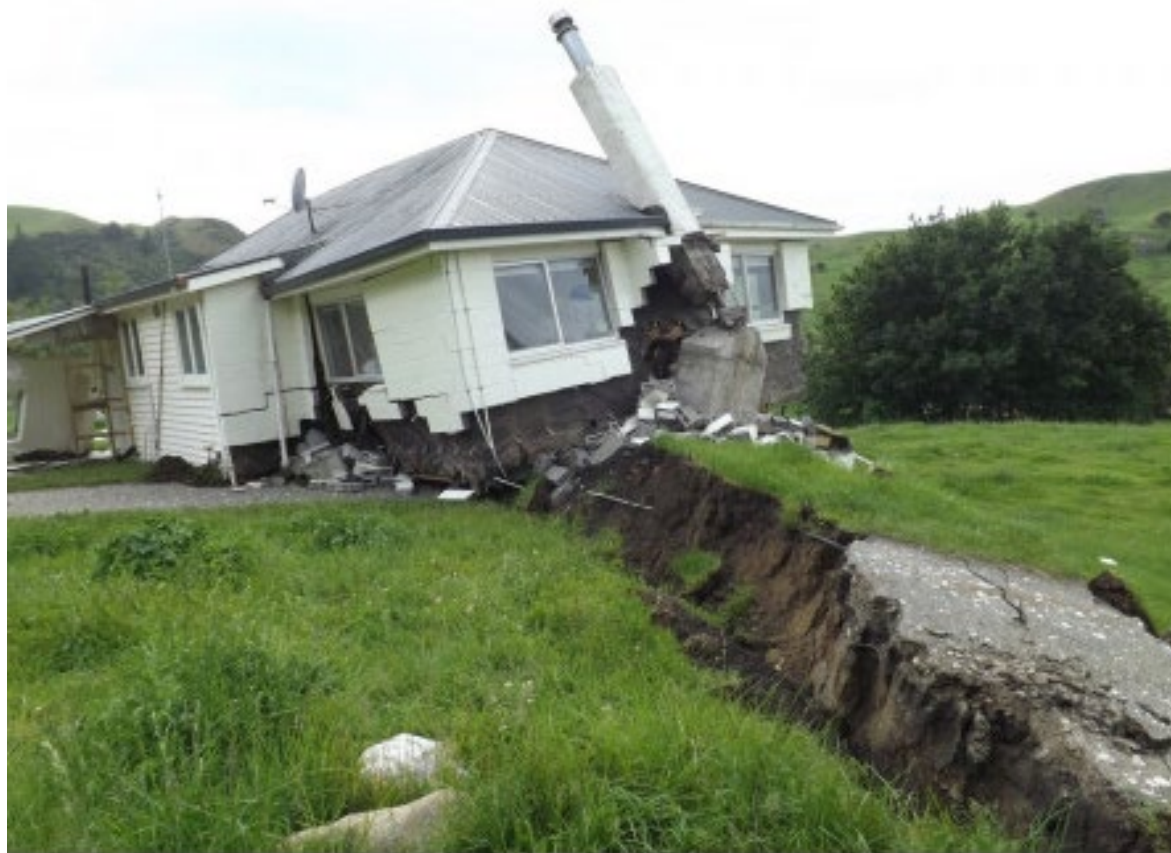
Figure 7 Consequence of a fault rupturing under a house, Kēkerengū Valley, Kaikōura earthquake 2016.
