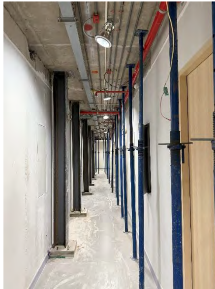
(k) Support system along the hallway, Level 8
