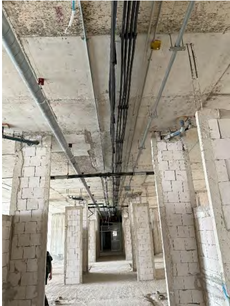
(a) A view of infill walls and services pipes
