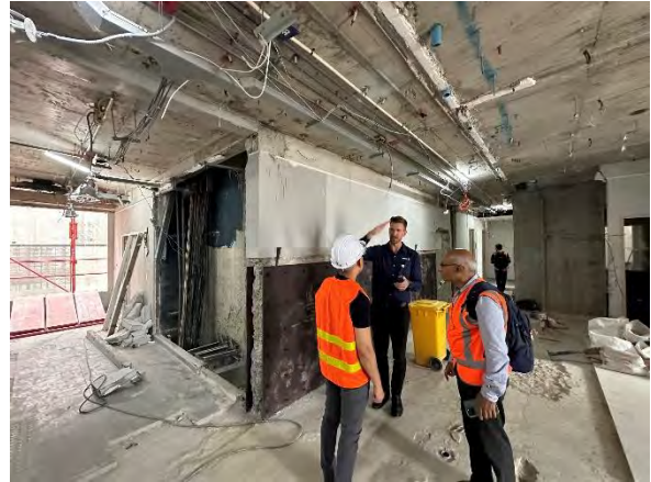
(b) Steel plates attached on walls of 10 th floor
