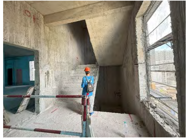
(b) Staircase with structural RC walls (typical thickness 250 mm thick)
