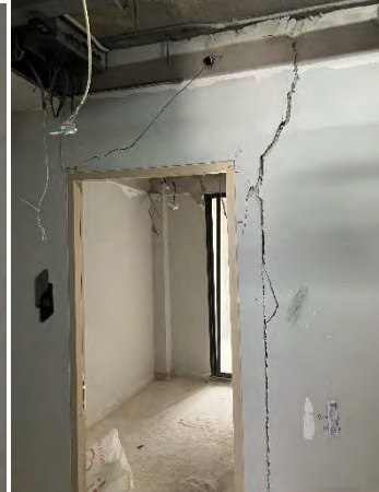
Figure 34: Potential damage to the adjacent building to Building R1
