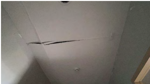
(b) Damage to plasterboard ceilings on 8 th and 9 th stories (typical)
