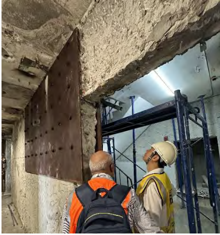
(a) Steel plates attached on walls of the 8 th floor
