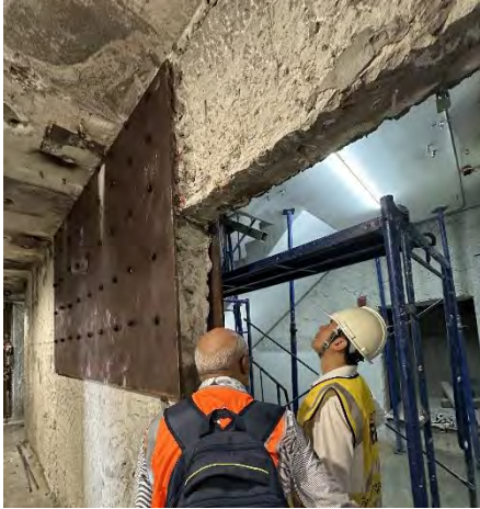
(a) Steel plates attached on walls of 8 th floor
