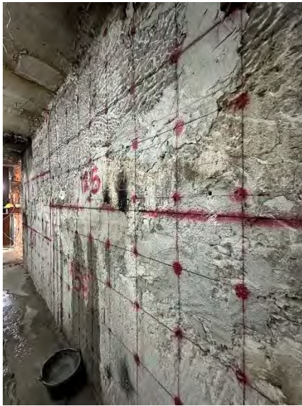
(c) Holes drilled into the wall to have bolts pass through the wall, 9 th floor
