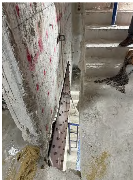
(h) Stair slab cut through to insert steel plate
