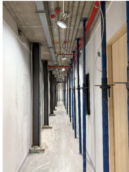
(l) Support system along hallway, 8 th floor
