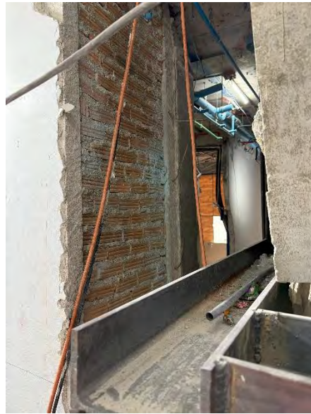
(f) Infill walls in toilet areas
