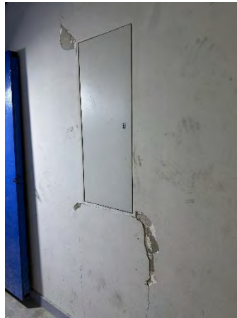
(a) Damage to infill walls on 8 th and 9 th stories (typical)
