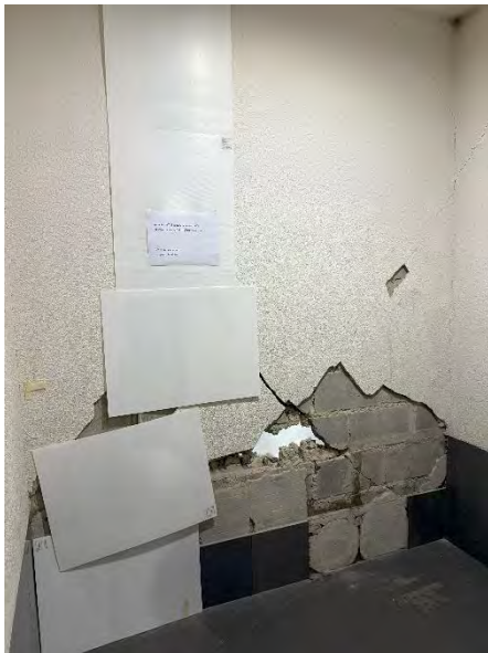
(g) Concrete block walls, thickness 70 mm.
