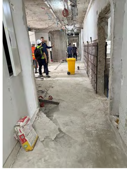
(j) Repair and strengthening, Level 9
