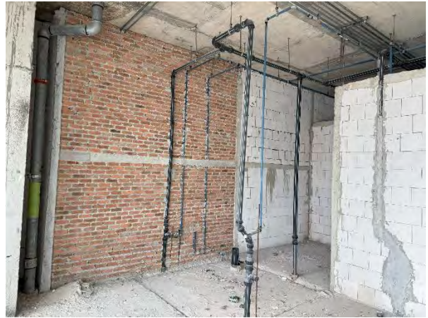
(b) Hollow brick (75 mm thick) infill wall
