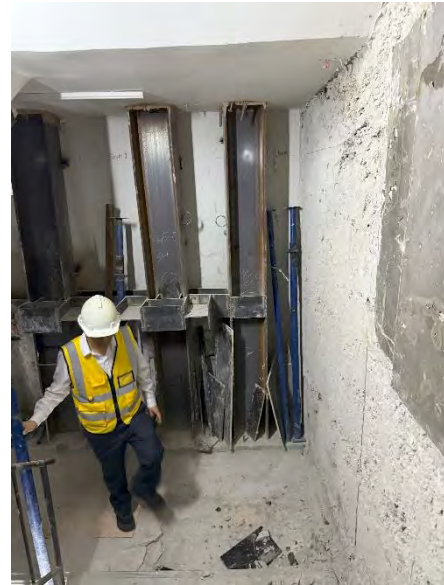
(h) New steel columns supported by corbels
