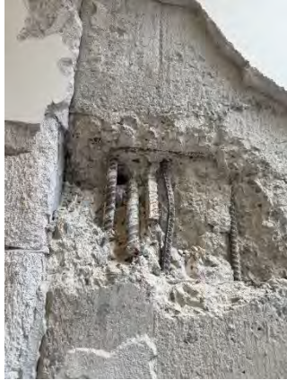
(e) Rebar splicing in the short RC wall along X-Dir
