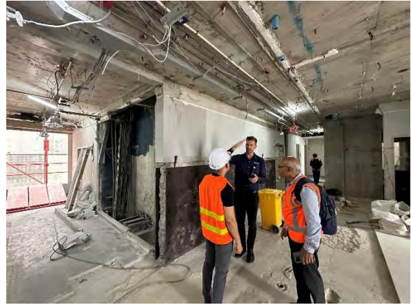
(b) Steel plates attached on walls of the 10 th floor
