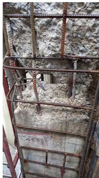
(c) Jacketing repair of wall
