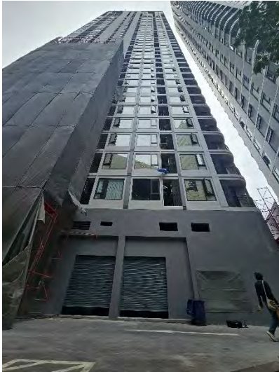
(a) Photo of Station 01 placed on the ground outside of building R1, near rolling doors to the loading bay
