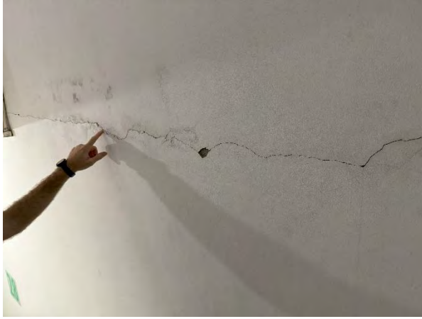
Figure 40: Damage at the interface of floor slab and non-structural walls (Level 28) in Building R3
