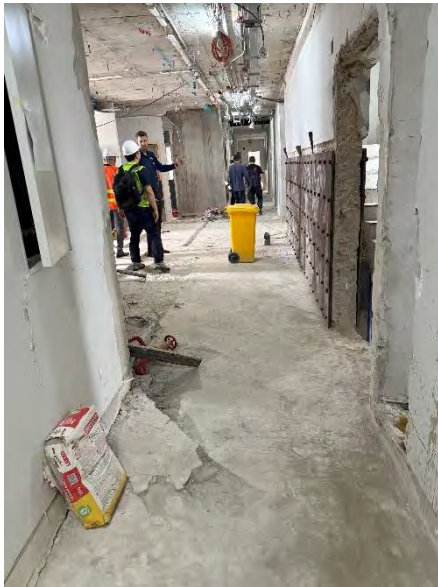
(k) Repair and strengthening, 9 th floor
