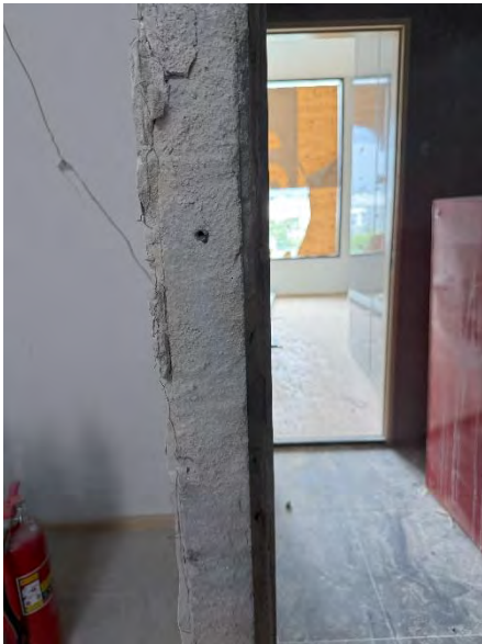
(e) A typical infill wall constructed of AC blocks with chicken mesh plastering
