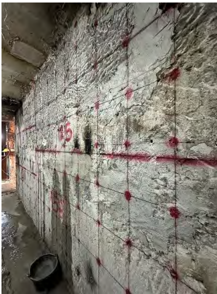
(c) Holes being drilled into the wall for bolts pass through the wall, 9 th floor
