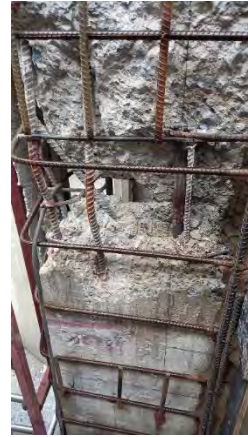
(f) Jacketing repair of wall
