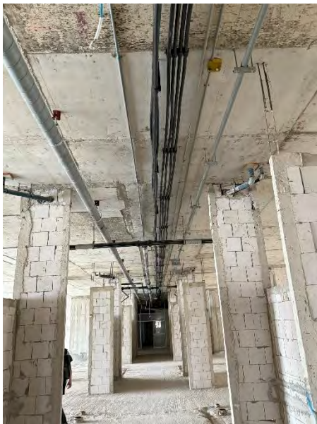
(c) A view of infill walls and services pipes
