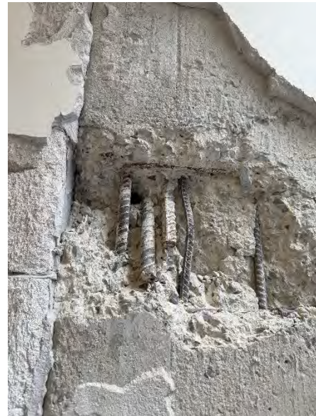
(d) Rebar splicing in the short reinforced concrete wall along the X-direction
