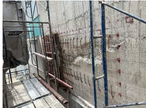
(b) Repair to exterior Y-direction wall with epoxied dowel bars
