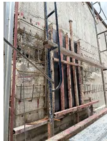
(h) Repair to exterior Y-direction wall with epoxied dowel bars
