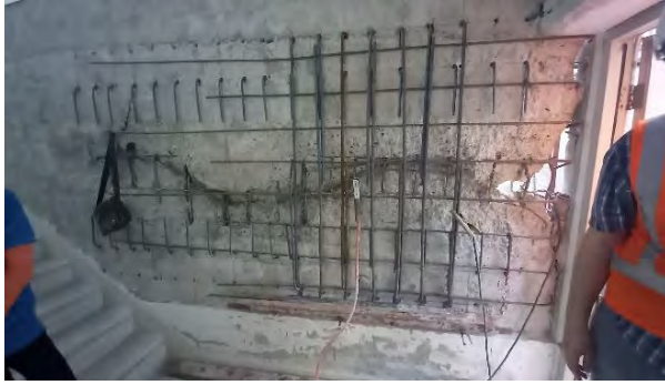
(a) Repair to Y-direction wall
