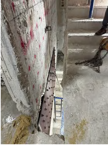
(i) Stair slab cut through to insert a steel plate
