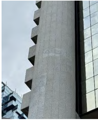
(e) Damage to the exterior concrete block wall (plaster spalling, relatively lighter white colour) has already been repaired.
