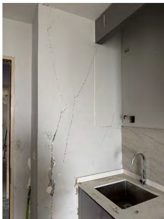
(a) Damage to infill walls on 8 th and 9 th stories (typical)
