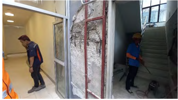
(b) Repair to through-thickness failure of wall in x-direction
