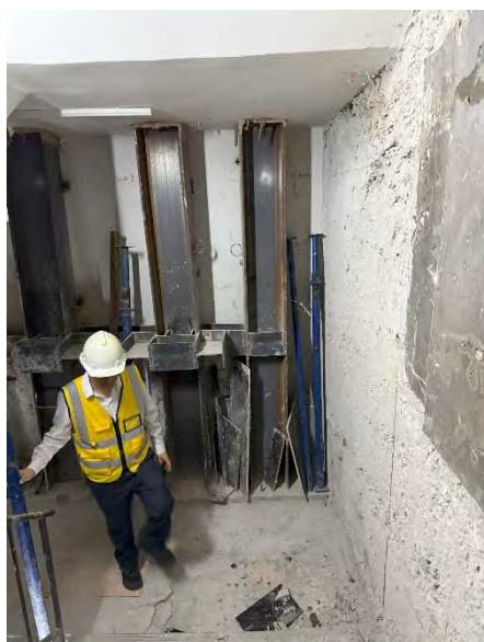
(g) New steel columns supported by corbels
