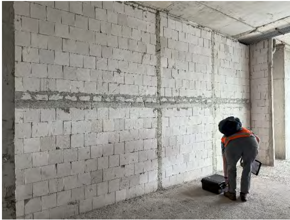
(a) AC infill wall (75 mm thick), note mostly dry joints
