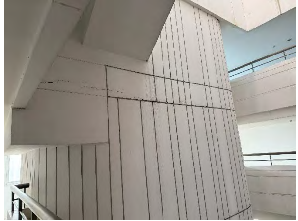
Figure 40: Damage at the interface of floor slab and non-structural walls (Level 28) in Building R3
