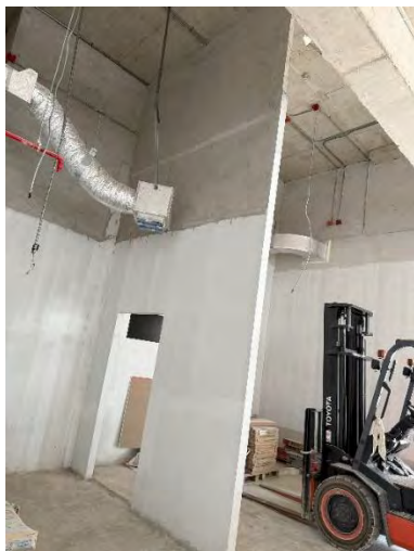
(a) Non-structural infill wall (wall height approximately 6 m) (ground floor)
