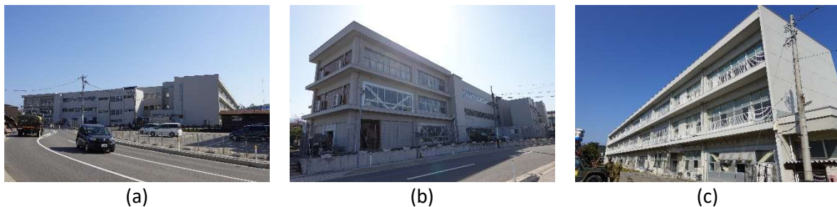
Figure 24: Building W2: (a) Overview of School W2, (b) Overview of South Building, (c) Overview of North Building
