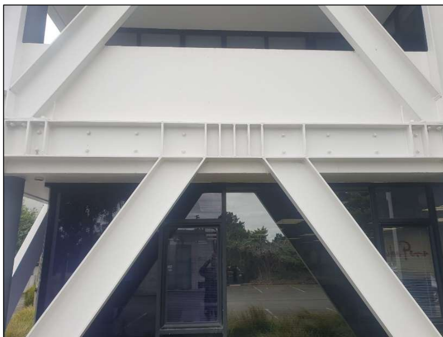
Figure 2. Connection between EBF and Concrete Frame not allowing for differences between deformed shapes.
