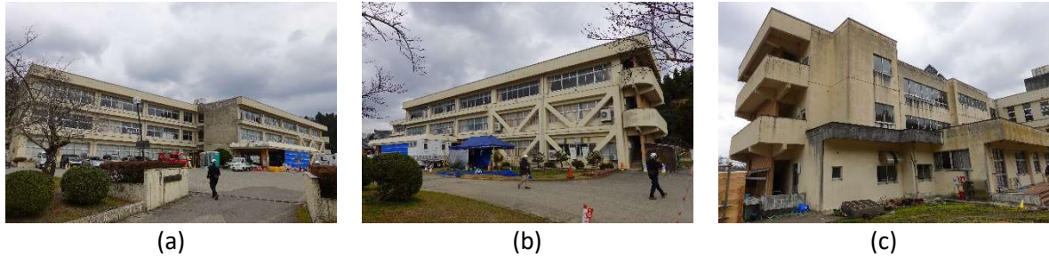
Figure 26: Building S4: (a) Overview of School W2, (b) Overview of South exterior frame of South Building, (c) Overview of North exterior frame of North Building
