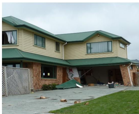
Photograph C.2. Very severe land damage (lateral spreading)
