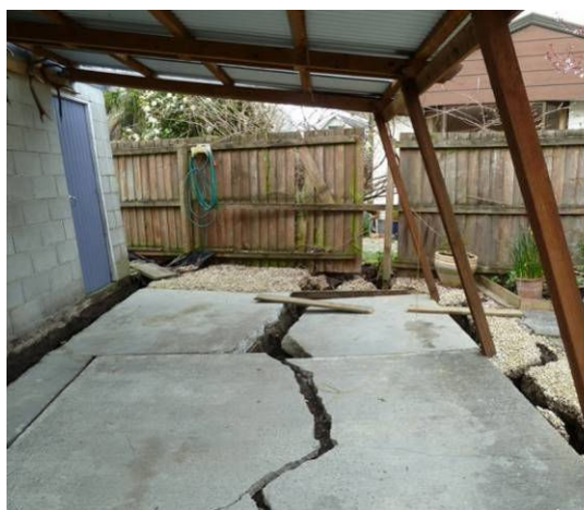
Photograph C.1. Very severe land damage (lateral spreading)
