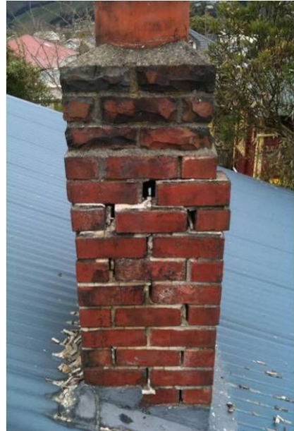
Photograph C.10. Chimney damage
