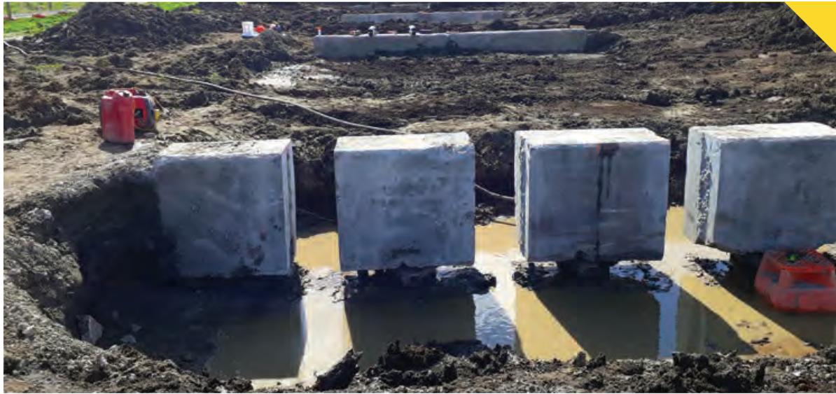
► Bridge piles ready to test
