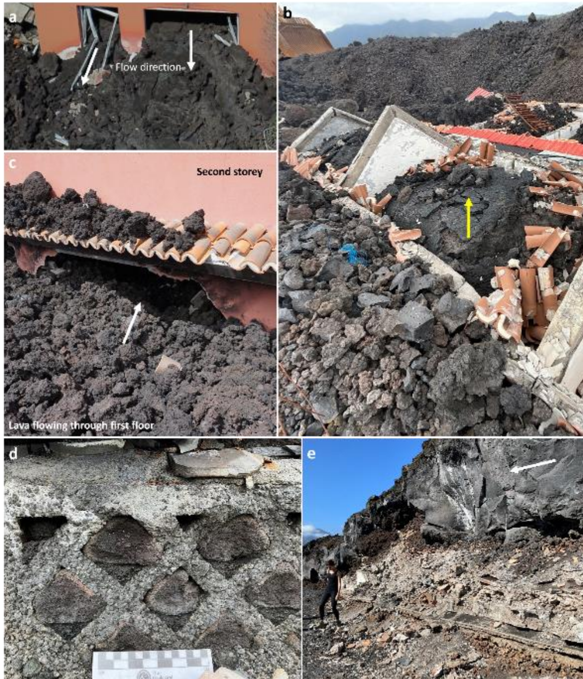
Figure 8. Variable lava flow inundation across structures: a) lava flowing through a building and out of the window and door with the structure still standing; b) lava flowed through the back wall then rose up into the structure (yellow arrow); c) lava flowing into the lower floor of a two storey building while the structure remains standing; d) lava flowing through gaps in a boundary wall, the upper marks on the scale are 1 cm; e) complete inundation and burial. The white arrows show lava flow direction.
