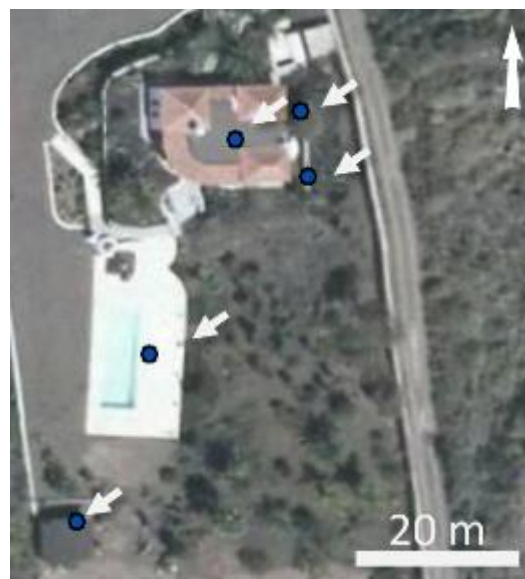
Figure 4. An example of one property with five damage grades. Here, we assigned a damage state of 4 for this building. White arrows indicate flow direction.
