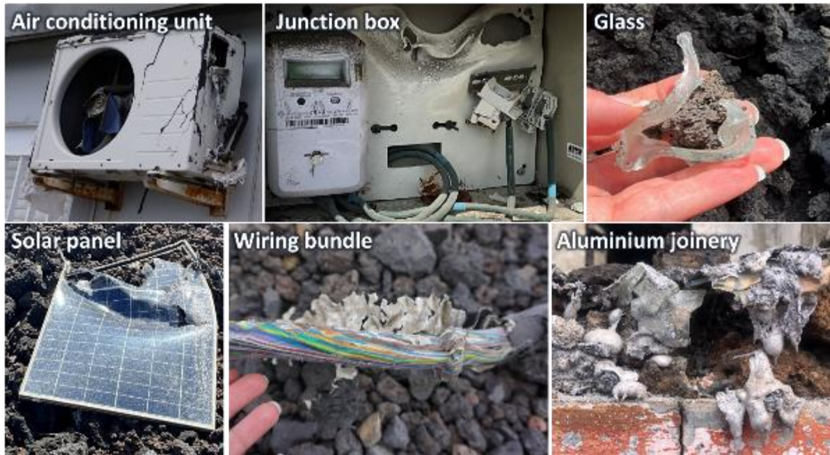
Figure 9. Thermal damage to different materials around the lava flow field boundary.
