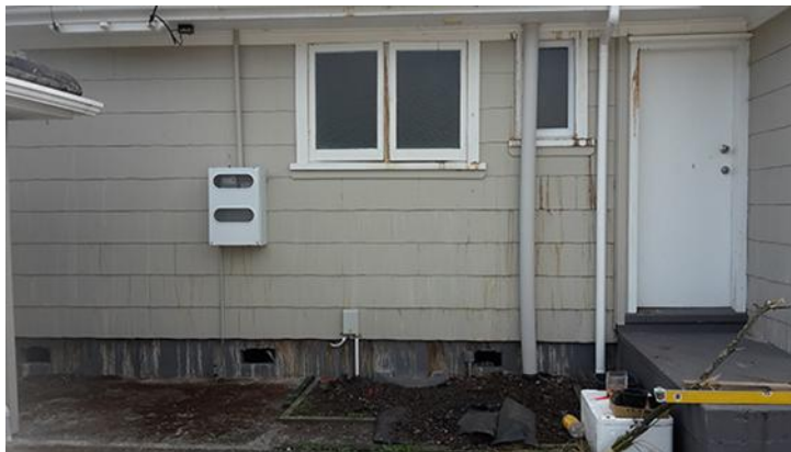
Figure 4 Heat damage to cladding from hydrothermal activity
