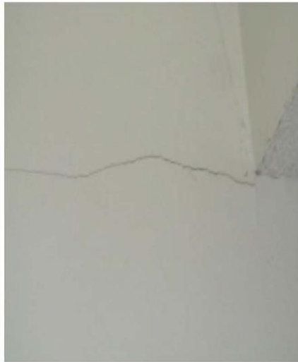
Bedroom 2 – 1.2 LM crack to painted plastered wall. Discoloured & aged. Not EQ-related.
