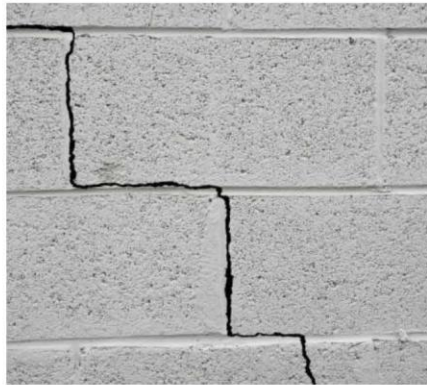
Intertenancy wall between Unit 1 & 2 – 1.0 LM structural crack through concrete block mortar. EQ-related.
