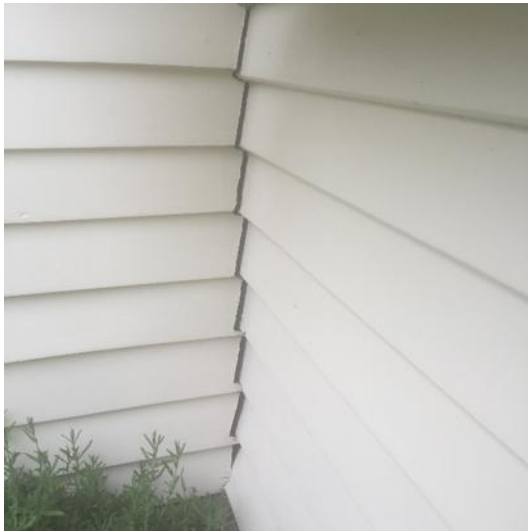
Figure 7 Weatherboard movement and cracking
