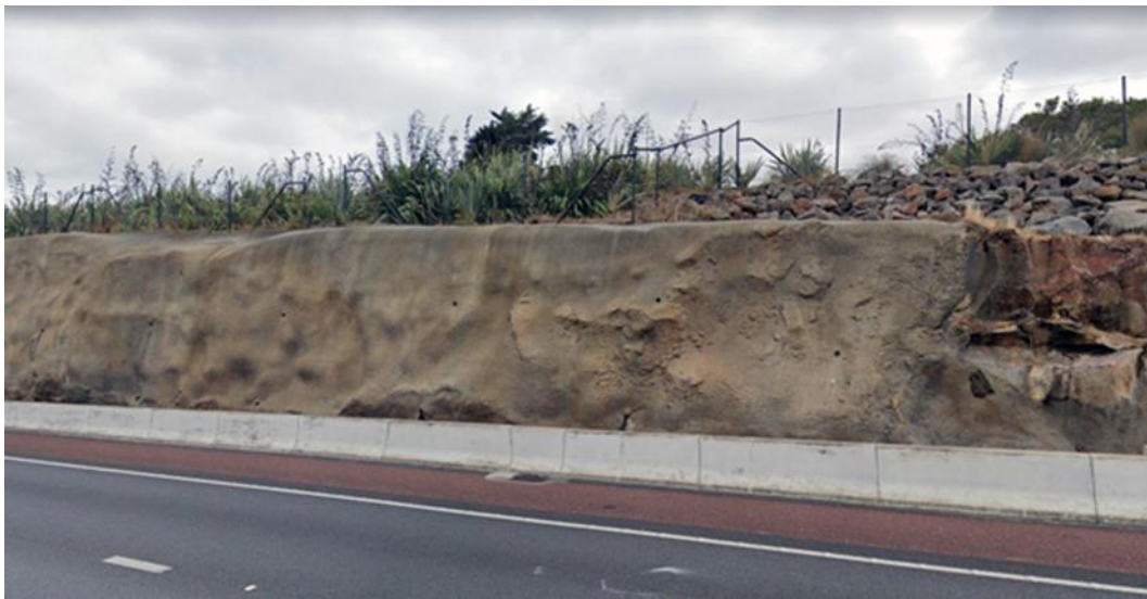
Figure 57 Sprayed concrete retaining wall
