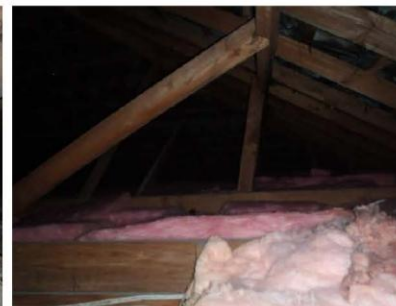
Figure 2: Timber rafters and struts
