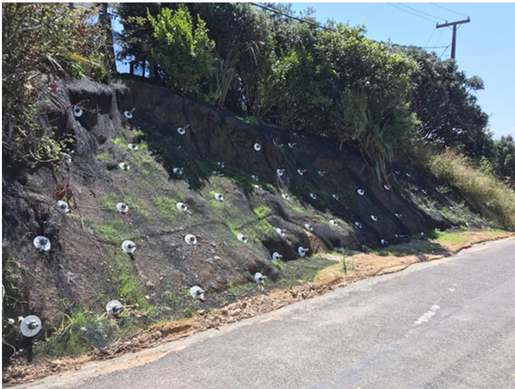
Figure 55 Soil nail retaining wall
