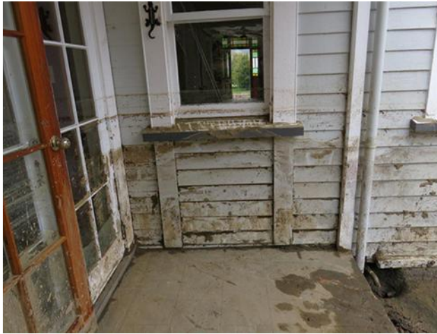
Figure 8 Moisture damage to weatherboards
