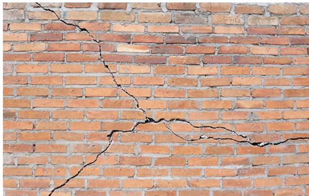
Figure 14 Severely cracked brick wall
