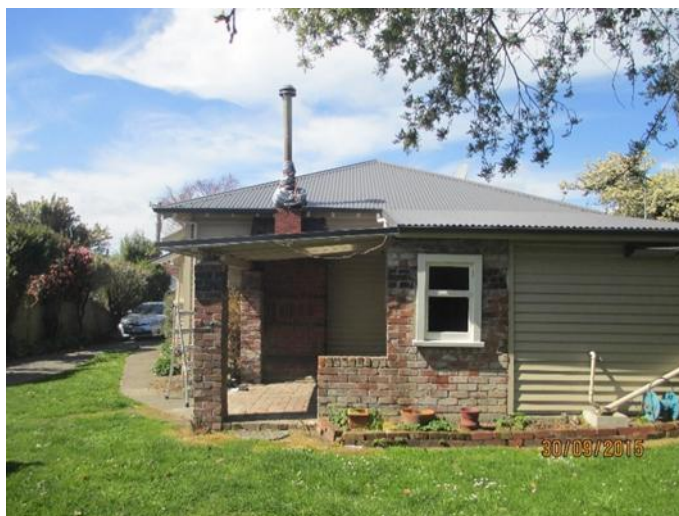
Figure 27 Disconnected flue with temporary waterproofing measures
