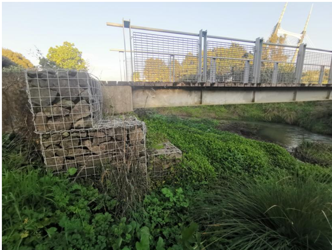
Figure 50 Gabion basket scour protection
