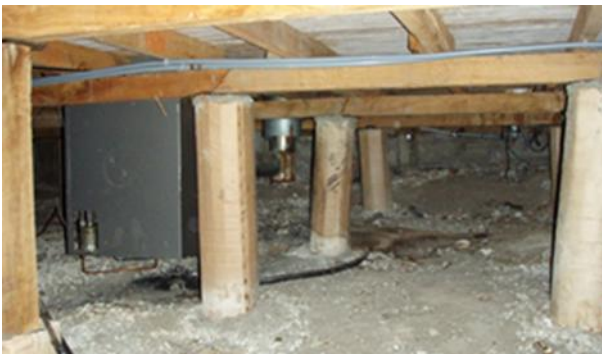
Figure 21 Pile detachment and rotation
