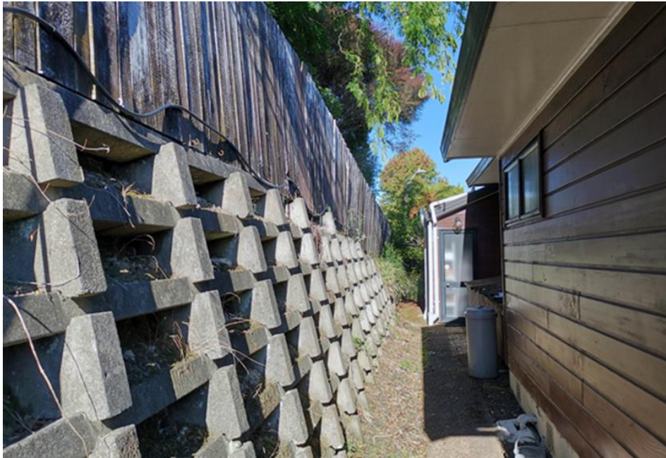
Figure 48 Concrete crib retaining wall
