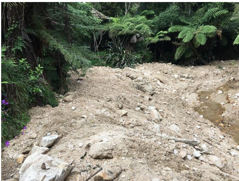
Figure 42 Stacked stone retaining wall washed away by flood waters
