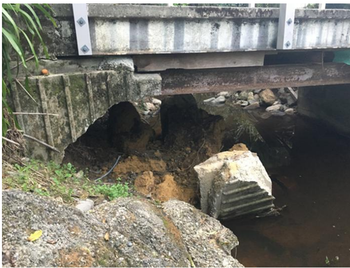
Figure 38 Impact damage to a bridge abutment from flood debris
