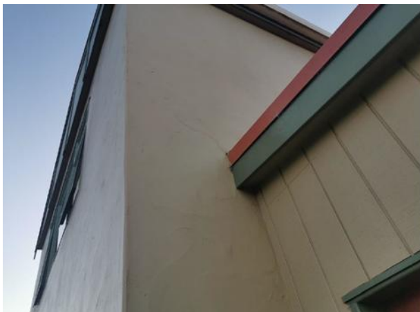
Figure 11 Cracked stucco panel
