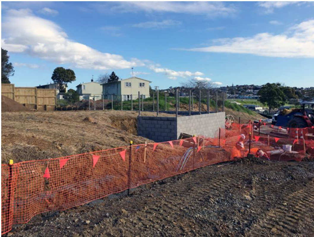
Figure 52 Concrete block retaining wall
