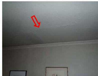
Figure 9: Ceiling crack in living area
