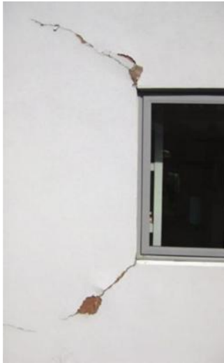
Figure 10 Cracked EIFS panel (BRANZ)
