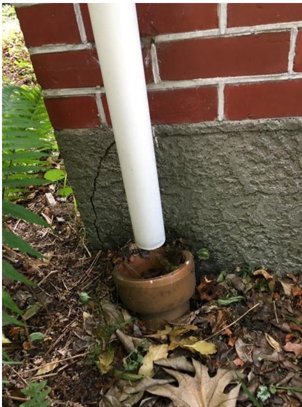
Figure 23 Cracked render finish
