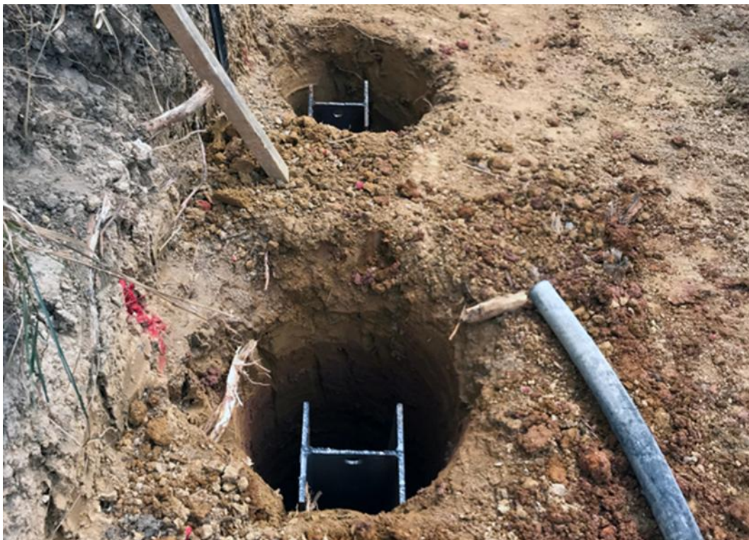
Figure 53 Reinforced concrete palisade wall holes
