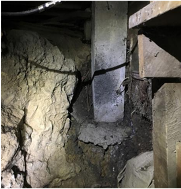
Figure 1 Pile settlement due to loss of support
