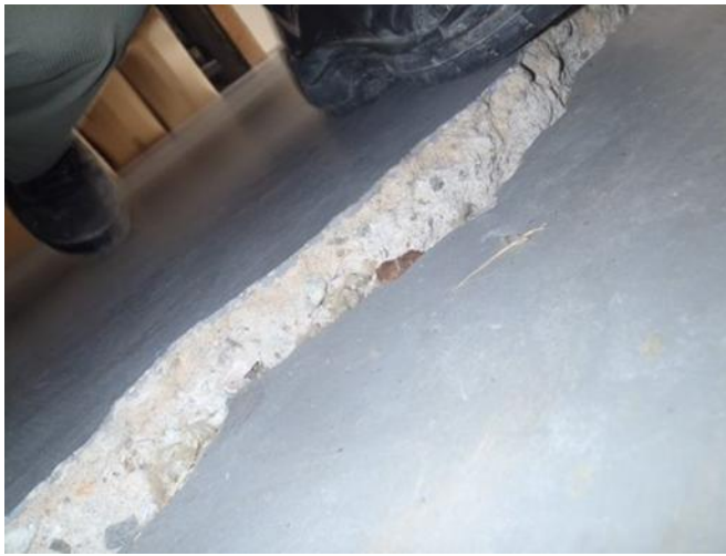
Figure 24 Cracking with vertical displacement
