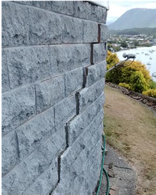
Figure 13 Step cracking to brick cladding with detachment
