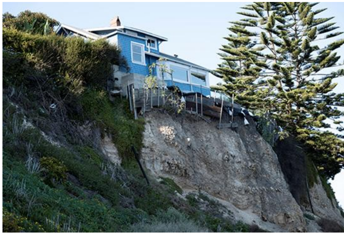
Figure 2 Landslide resulting in undermining of dwelling foundation
