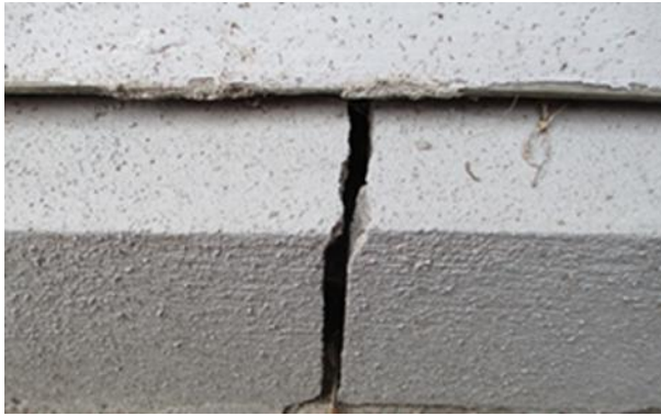
Figure 22 Cracked foundation
