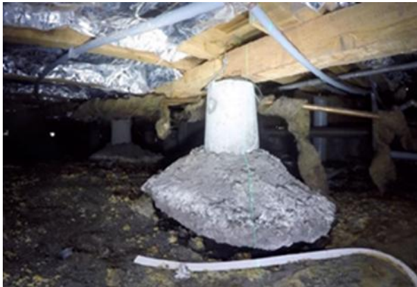
Figure 20 Loss of support resulting in settlement
