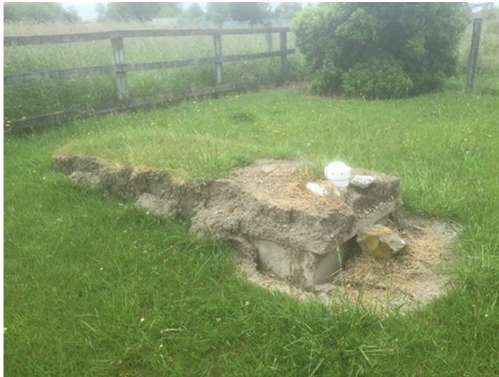
Figure 29 Displacement of septic tank
