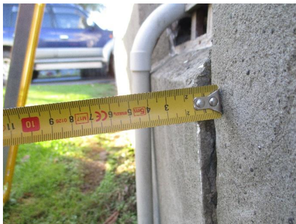
Figure 43 Out-of-plane displacement
