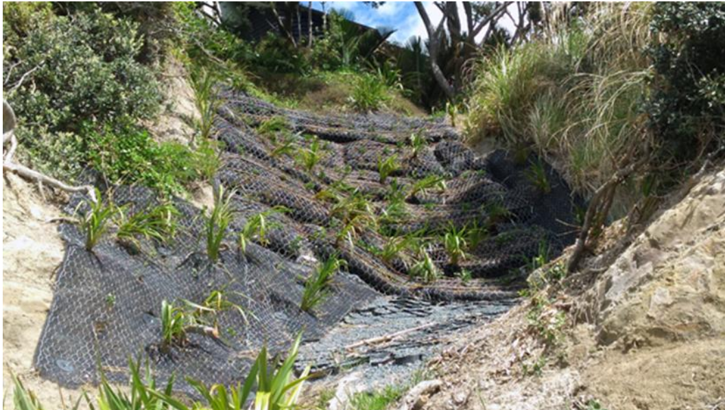
Figure 56 Pinned mesh retaining wall
