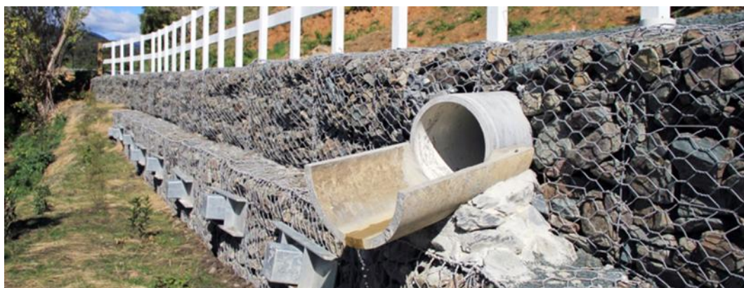
Figure 51 Gabion basket retaining wall
