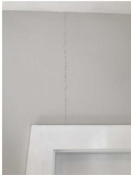
Bedroom 1 – 1.0 LM crack to painted plastered wall. EQ-related.
