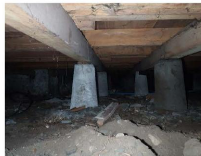
Figure 1: Precast concrete piles
