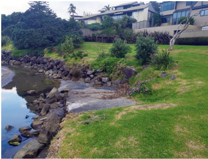
Figure 69 Riprap scour protection
