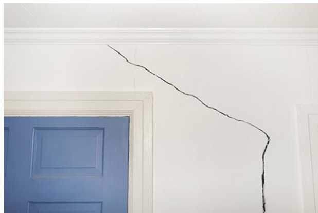
Figure 16 Structural cracking
