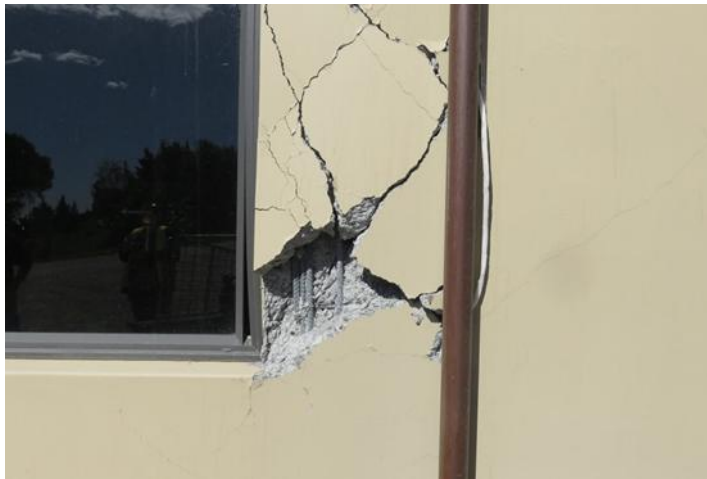
Figure 12 Cracked concrete panel
