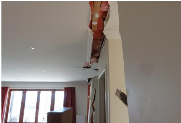
Figure 15 Structural cracking
