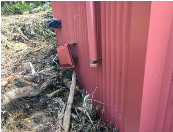
Figure 9 Impact damage to metal cladding
