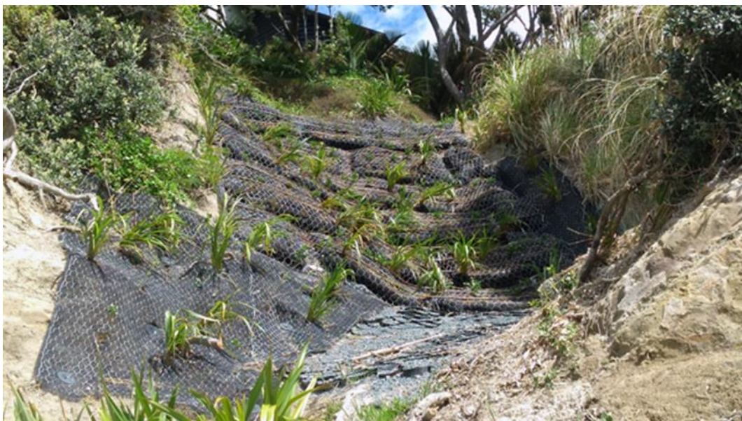
Figure 57 Pinned mesh retaining wall
