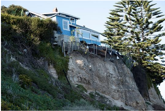
Figure 2 Natural landslip resulting in undermining of dwelling foundation
