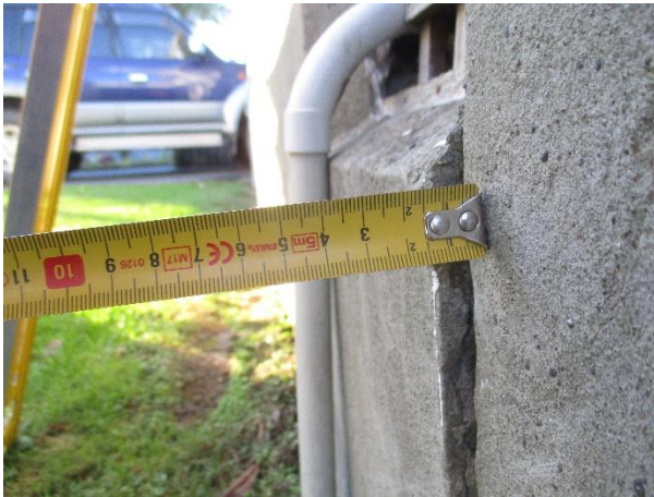
Figure 44 Out-of-plane displacement
