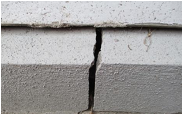
Figure 22 Cracked foundation
