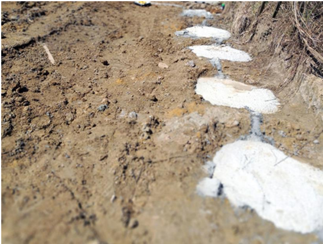
Figure 55 Reinforced concrete palisade wall – complete
