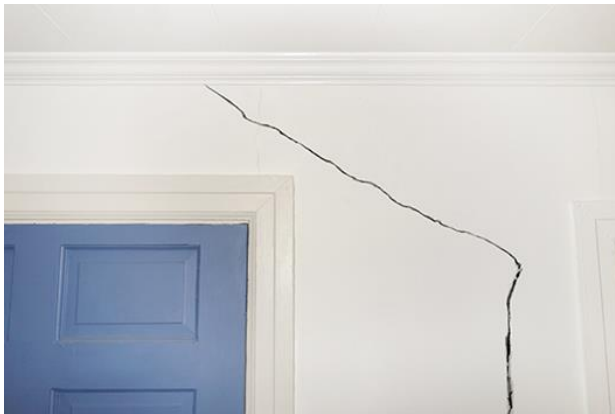
Figure 16 Structural cracking
