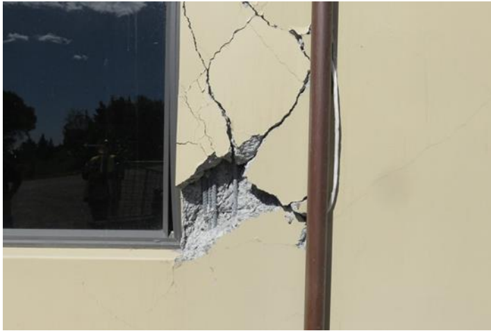
Figure 12 Cracked concrete panel
