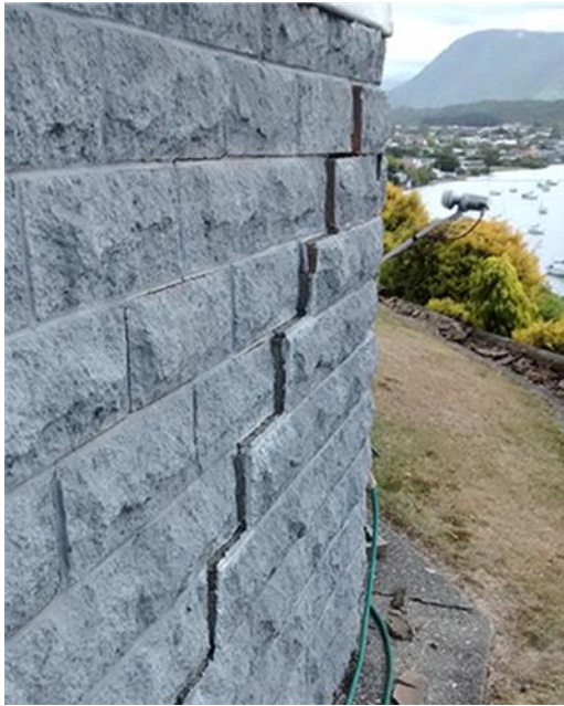
Figure 13 Step cracking to brick cladding with detachment
