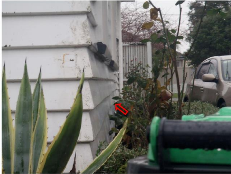
Figure 7: Timber weatherboards are visibly out of alignment
