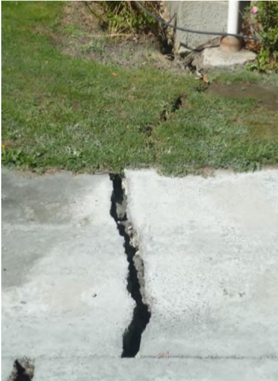
Figure 34 Cracking (oscillation movement of dwelling) due to earthquake
