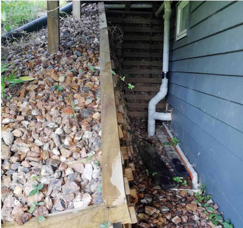
Figure 50 Timber crib retaining wall
