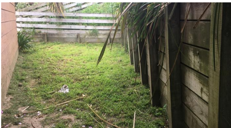
Figure 41 Timber retaining wall that has rotated due to land movement during a heavy rain event
