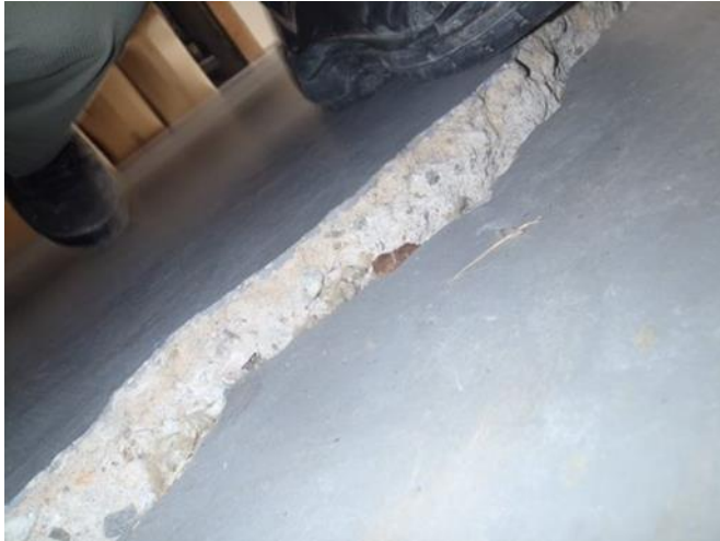
Figure 24 Cracking with vertical displacement
