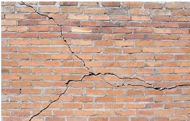
Figure 14 Severely cracked brick wall
