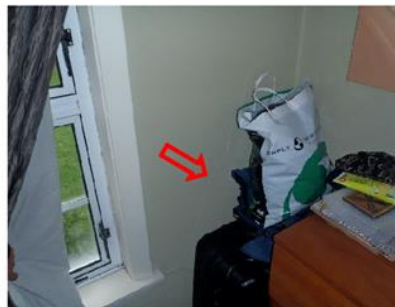
Figure 8: Diagonal wall lining crack in Bedroom 3
