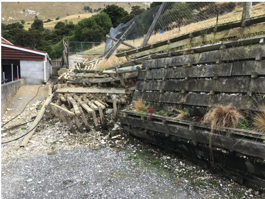
Figure 42 Timber crib retaining wall that has collapsed due to earthquake
