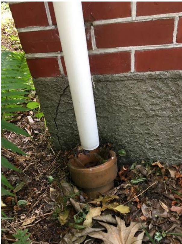
Figure 23 Cracked render finish
