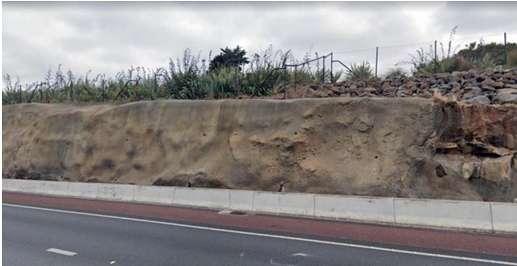
Figure 56 Sprayed concrete retaining wall
