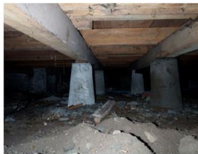
Figure 1: Precast concrete piles
