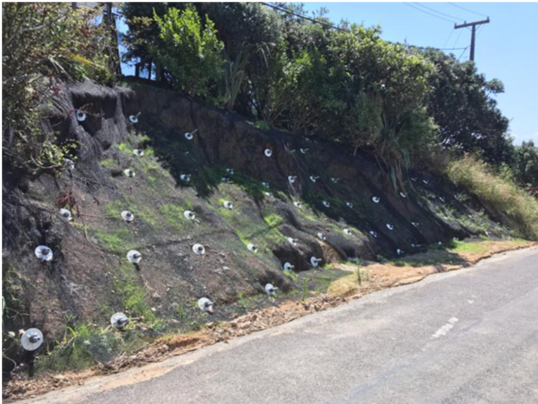
Figure 58 Soil nail retaining wall
