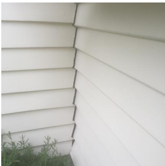
Figure 7 Weatherboard movement and cracking
