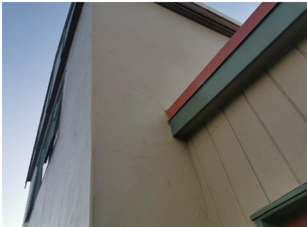
Figure 11 Cracked stucco panel
