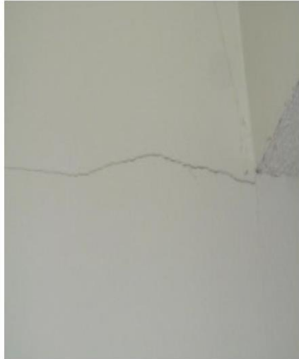
Bedroom 2 – 1.2 LM crack to painted plastered wall. Discoloured & aged. Not event-related.
