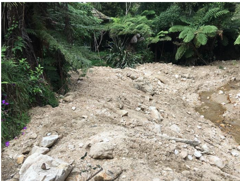
Figure 43 Stacked stone retaining wall washed away by flood waters
