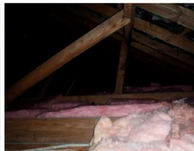
Figure 2: Timber rafters and struts
