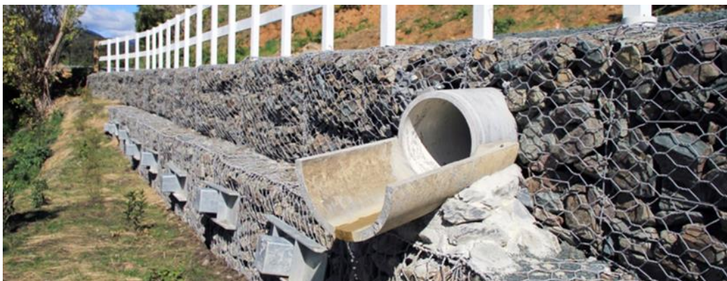
Figure 52 Gabion basket retaining wall
