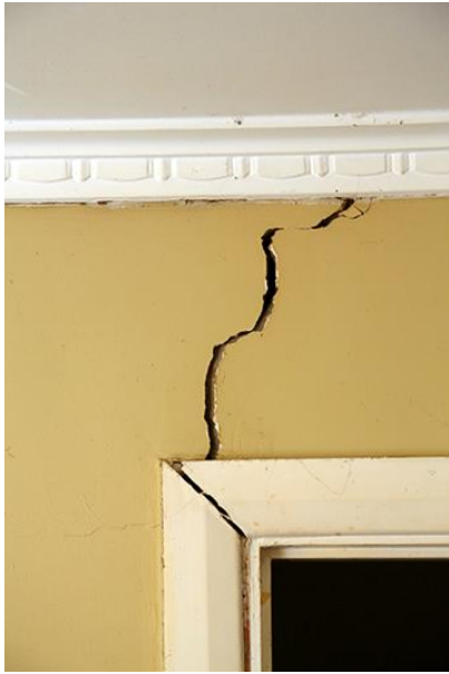
Figure 17 Structural cracking
