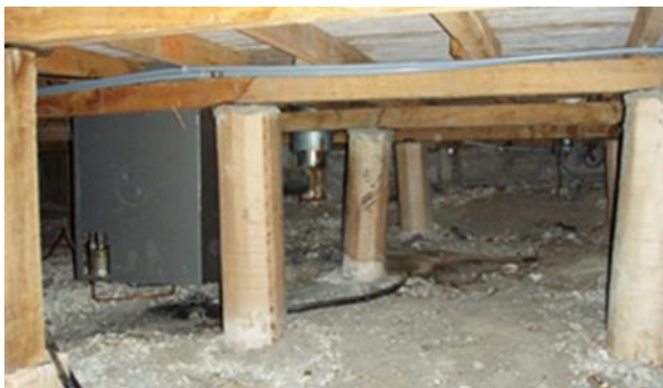
Figure 21 Pile detachment and rotation
