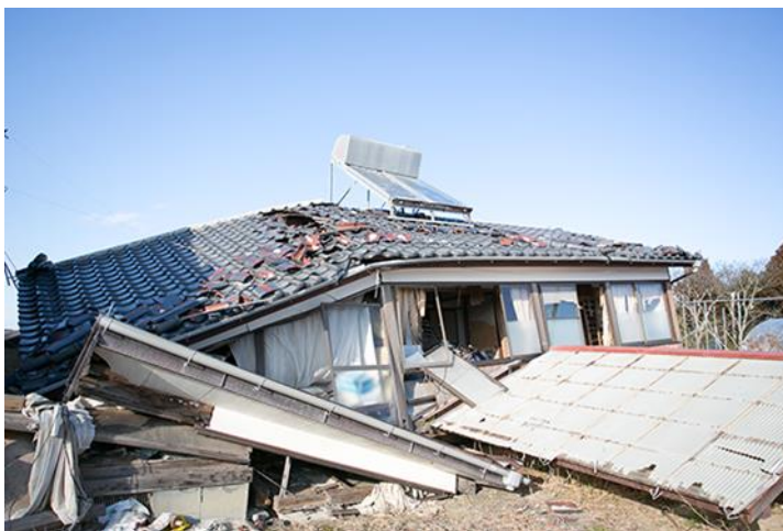
Figure 3 Total loss of dwelling due to tsunami impact
