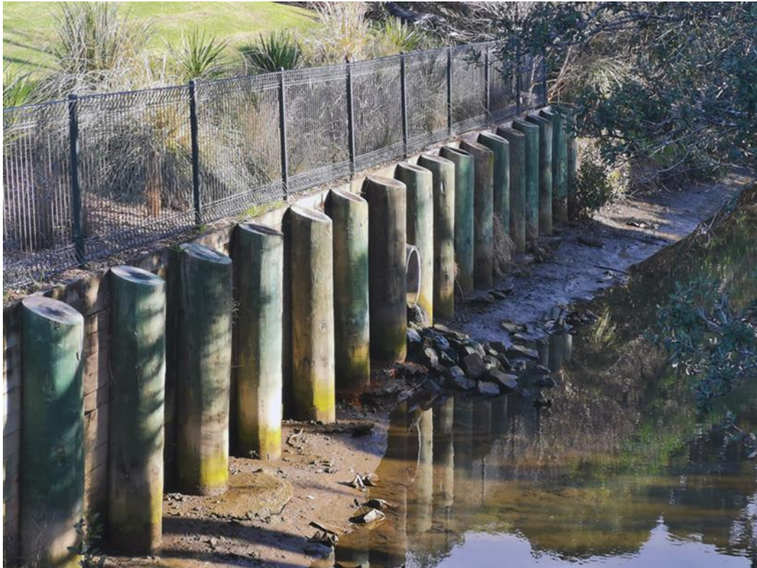
Figure 48 Timber pole retaining wall
