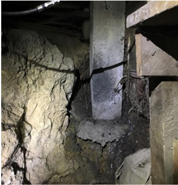
Figure 1 Pile settlement due to loss of support
