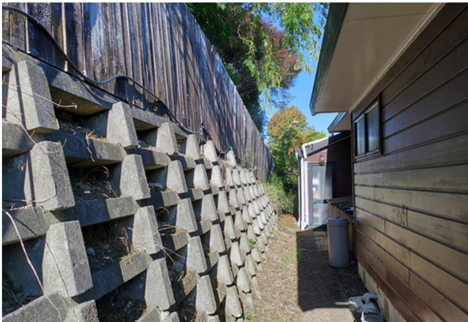
Figure 49 Concrete crib retaining wall
