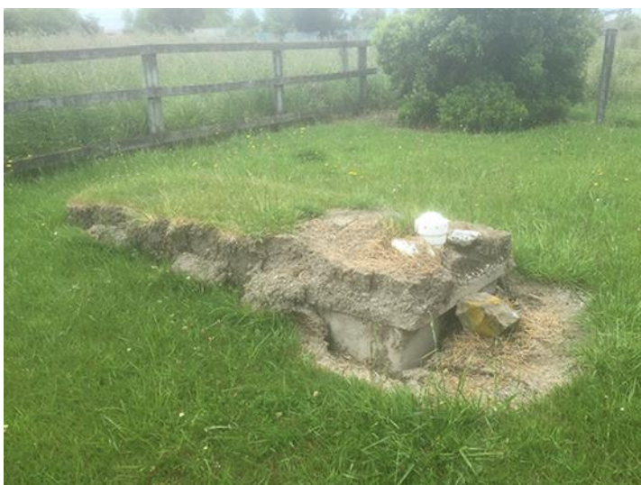
Figure 29 Displacement of septic tank
