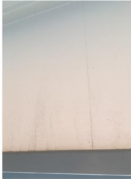
Bedroom 2 – 0.5 LM crack to painted plasterboard wall. EQ-related.
