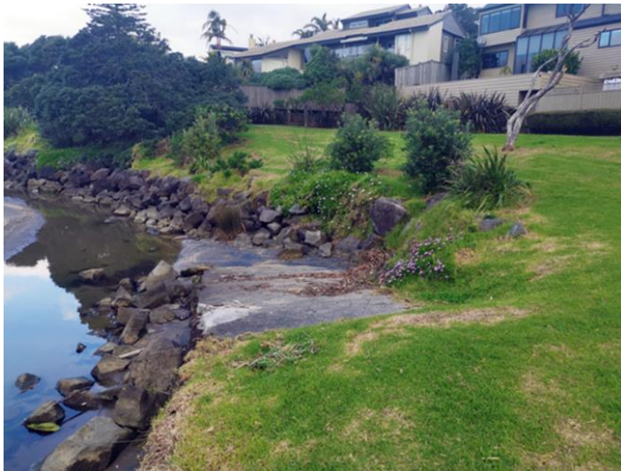
Figure 70 Riprap scour protection
