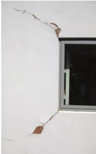
Figure 10 Cracked EIFS panel (BRANZ)
