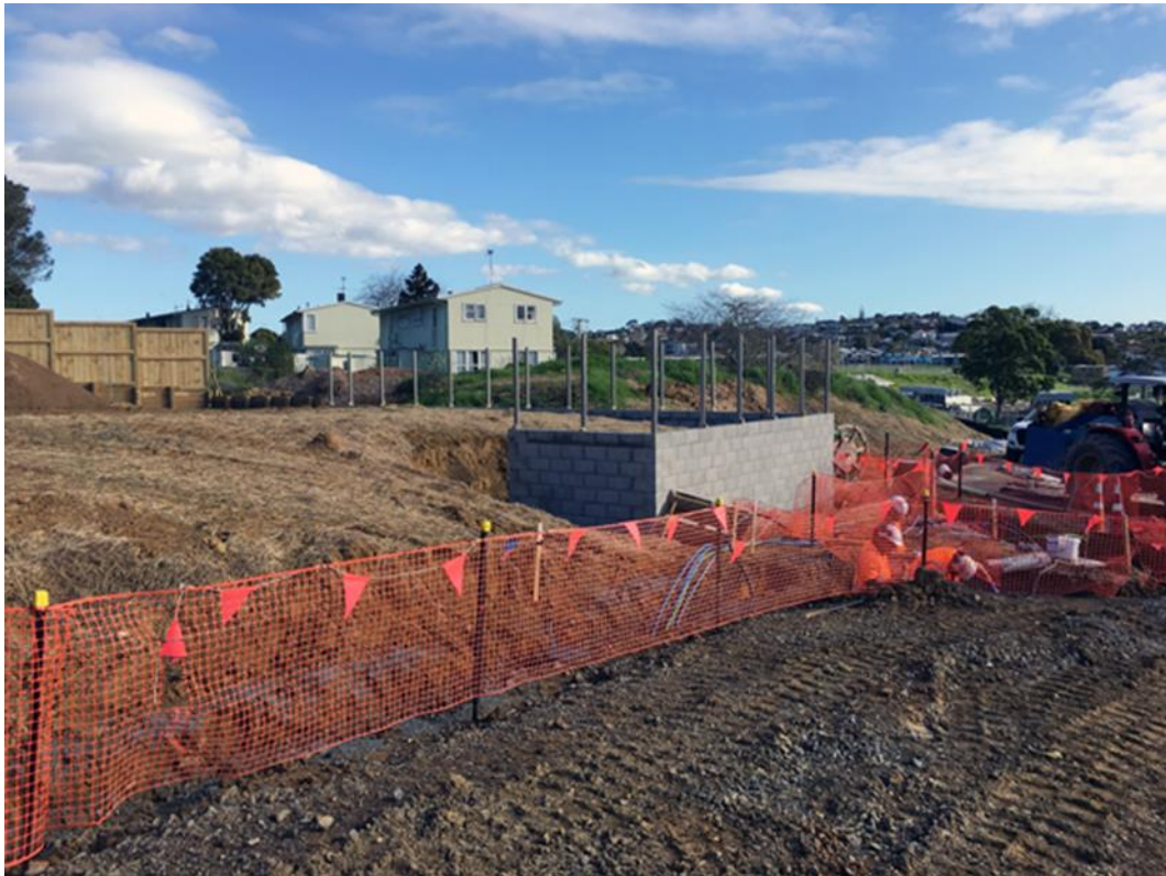
Figure 53 Concrete block retaining wall
