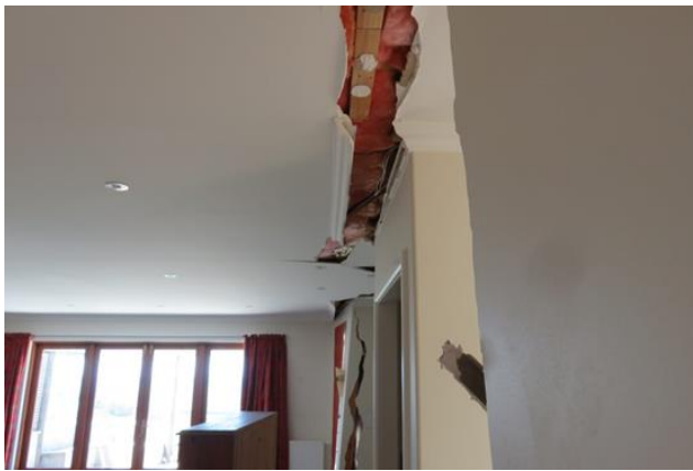
Figure 15 Structural cracking
