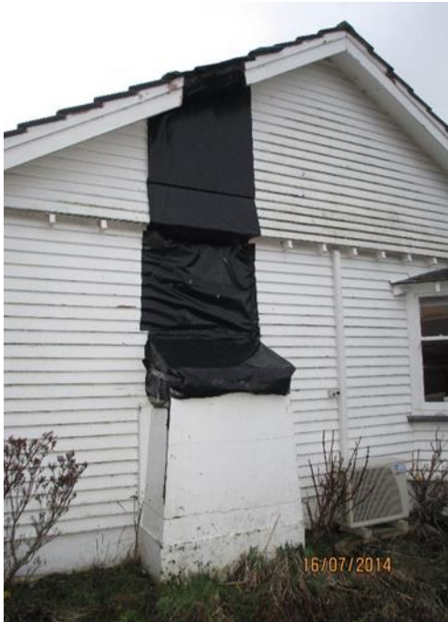
Figure 26 Total collapse of chimney with temporary waterproofing measures
