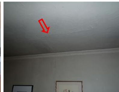
Figure 9: Ceiling crack in living area
