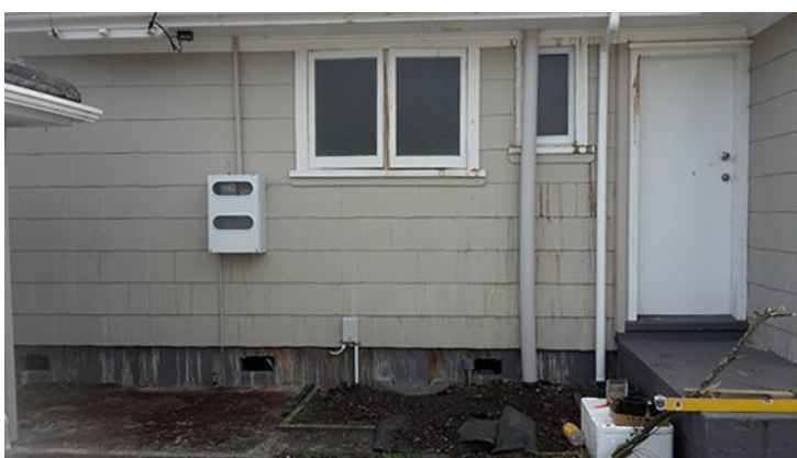
Figure 4 Heat damage to cladding from hydrothermal activity
