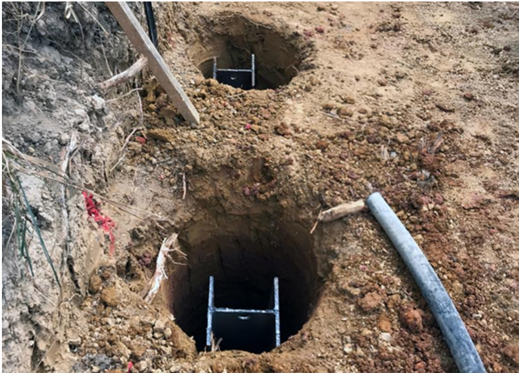
Figure 54 Reinforced concrete palisade wall holes
