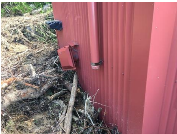
Figure 9 Impact damage to metal cladding
