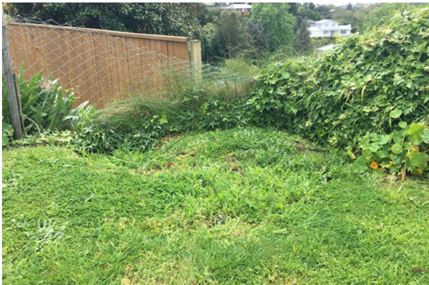
Figure 37 Localised settlement due to rotated retaining wall (obscured)
