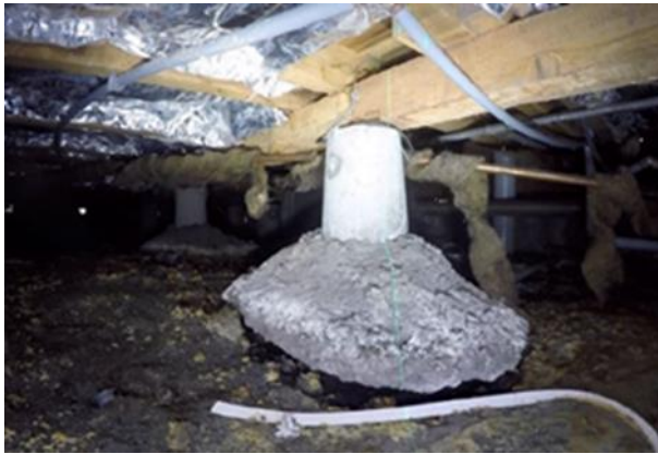
Figure 20 Loss of support resulting in settlement
