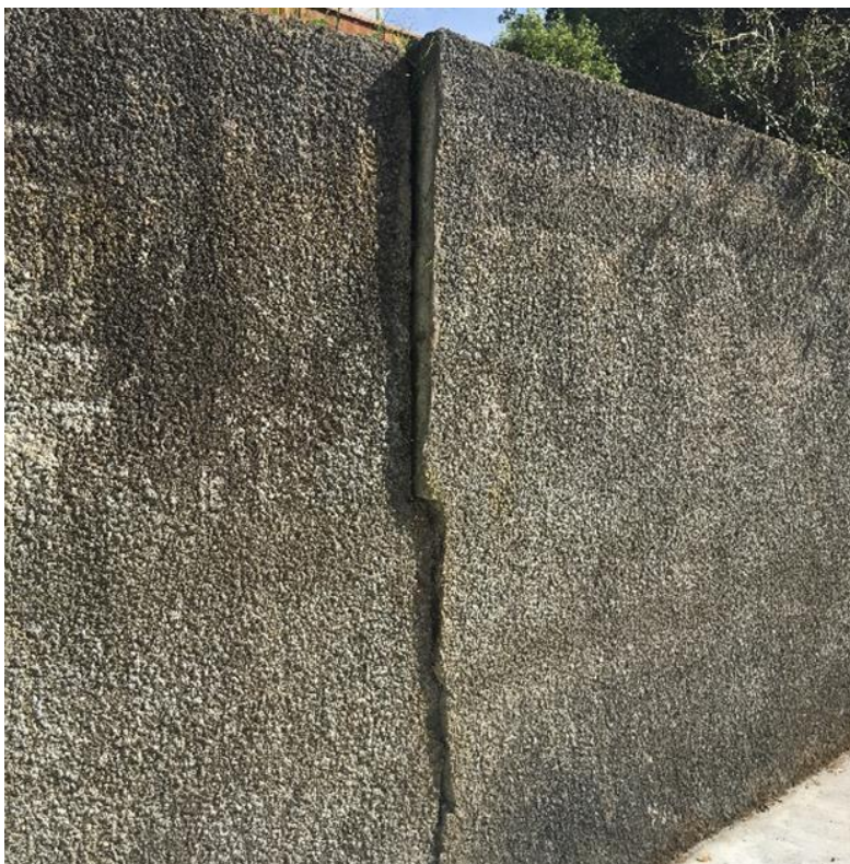
Figure 40 Retaining wall that has cracked due to earthquake
