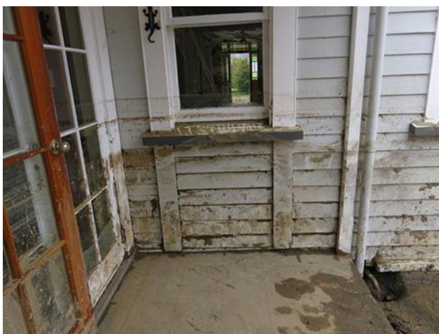
Figure 8 Moisture damage to weatherboards
