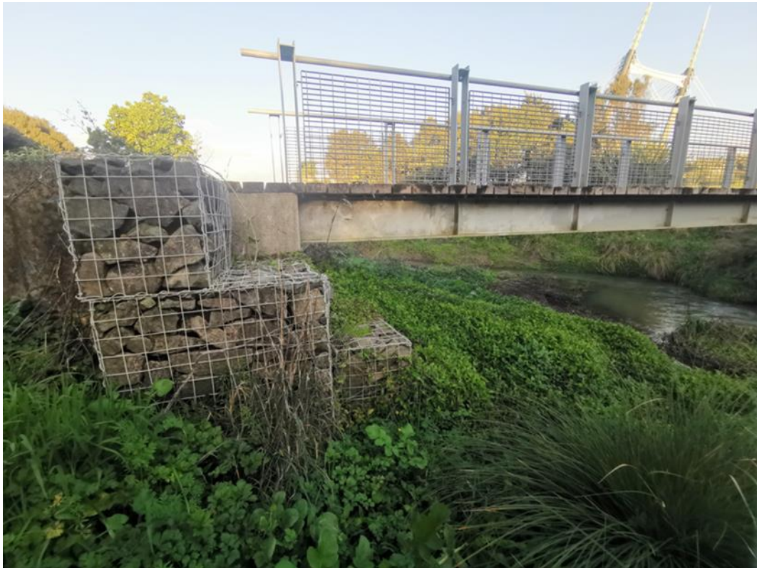
Figure 51 Gabion basket scour protection
