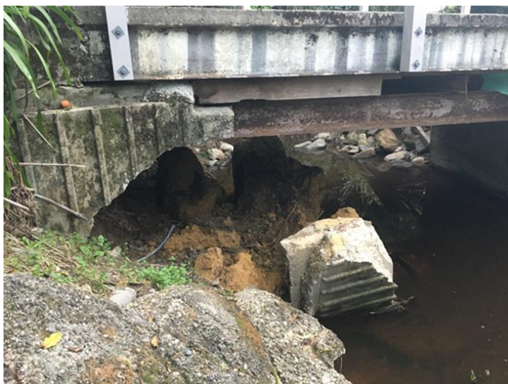
Figure 39 Impact damage to a bridge abutment from flood debris
