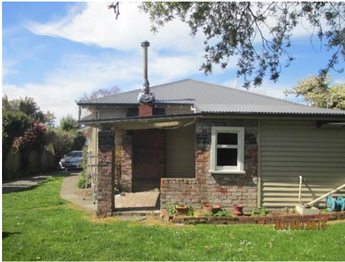
Figure 27 Disconnected flue with temporary waterproofing measures
