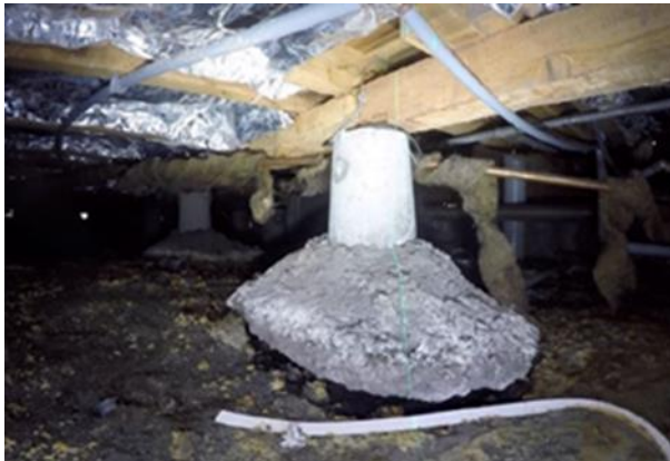
Figure 20 Loss of support resulting in settlement
