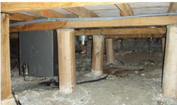
Figure 21 Pile detachment and rotation
