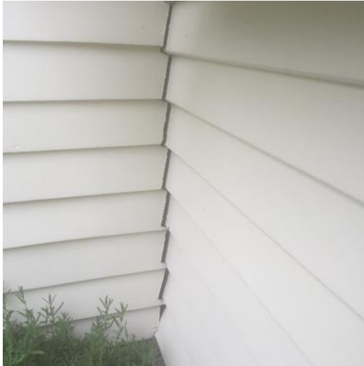
Figure 7 Weatherboard movement and cracking
