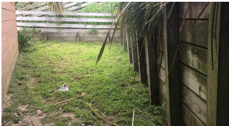
Figure 40 Timber retaining wall that has rotated due to land movement during a heavy rain event
