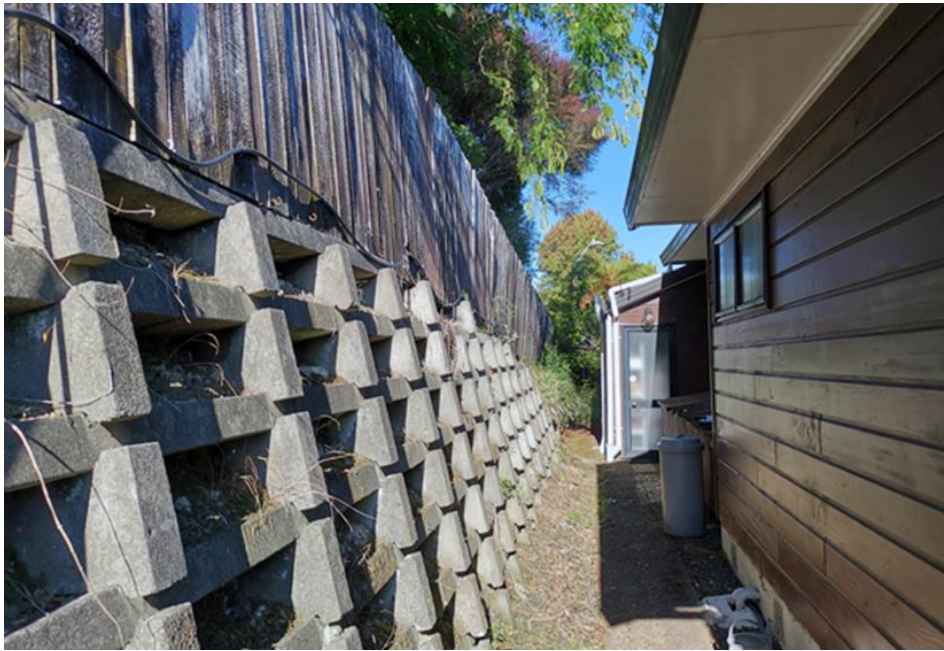
Figure 48 Concrete crib retaining wall
