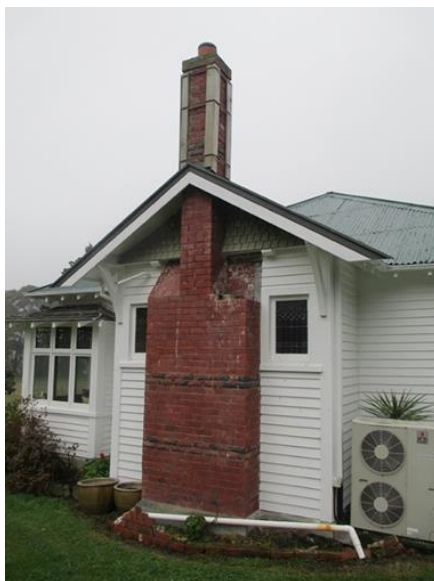
Figure 25 Chimney cracked at roofline with temporary supporting repairs
