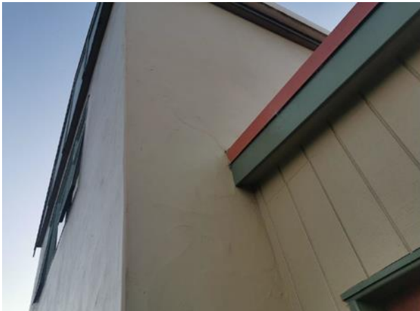
Figure 11 Cracked stucco panel
