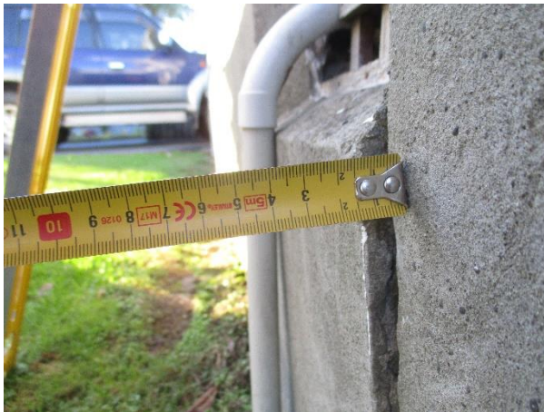
Figure 43 Out-of-plane displacement
