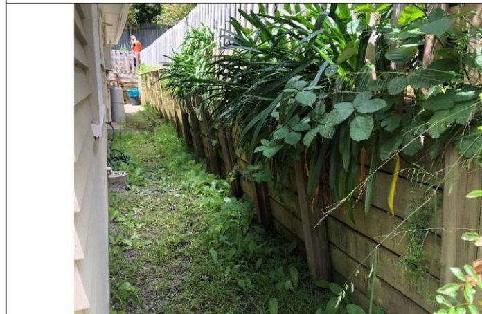
Photograph 2: View of rotation of RTW1 (taken 11 December 2024 facing east).
