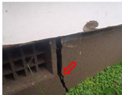
Figure 5: Fresh crack with sharp edges below North-facing window of Bedroom 3
