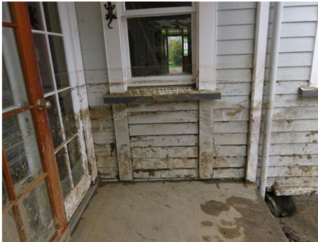
Figure 8 Moisture damage to weatherboards
