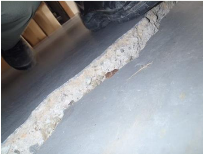
Figure 24 Cracking with vertical displacement
