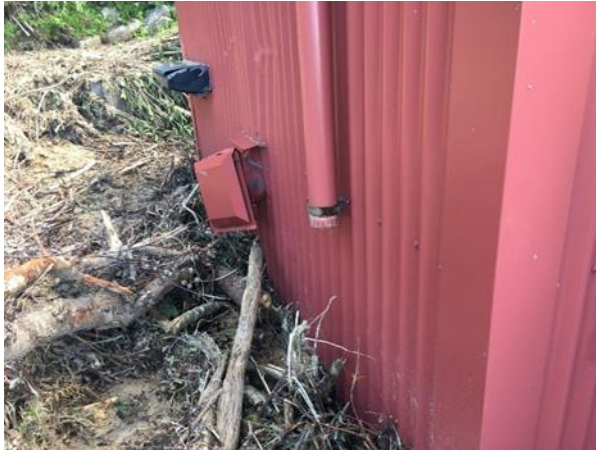
Figure 9 Impact damage to metal cladding
