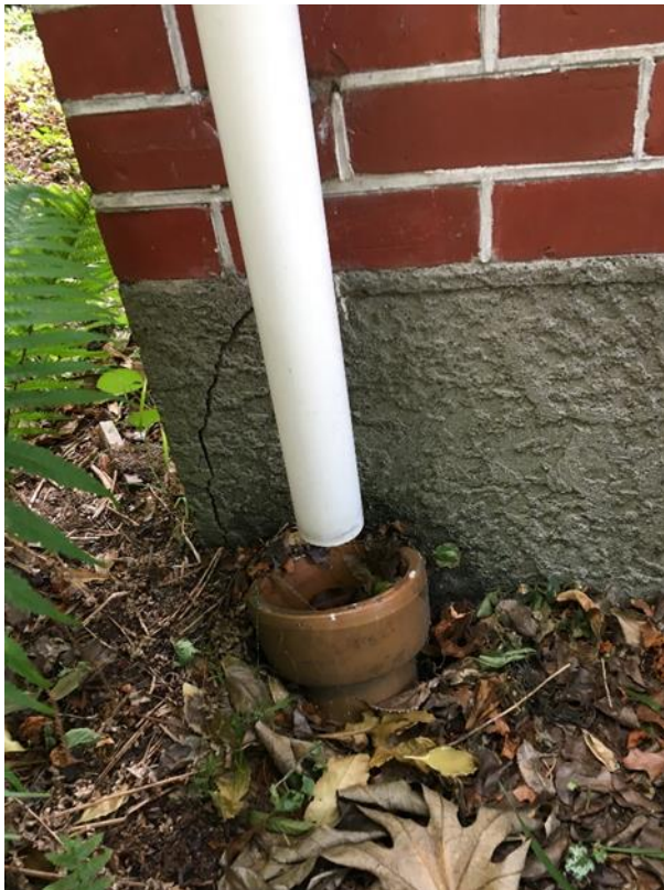
Figure 23 Cracked render finish
