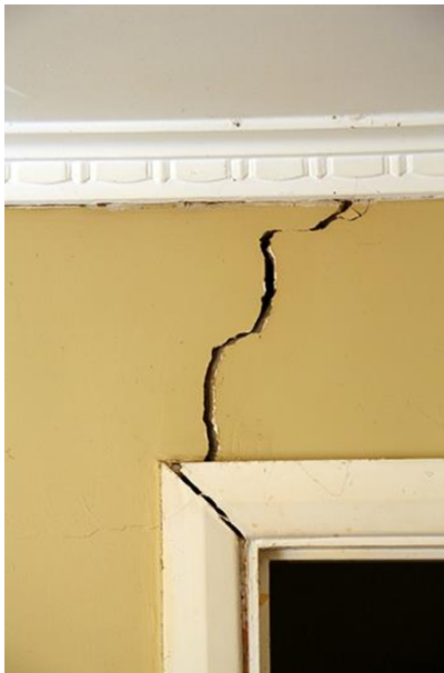
Figure 17 Structural cracking
