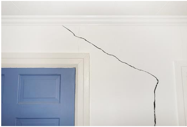
Figure 16 Structural cracking
