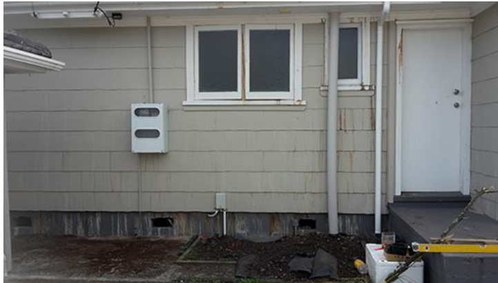
Figure 4 Heat damage to cladding from hydrothermal activity
