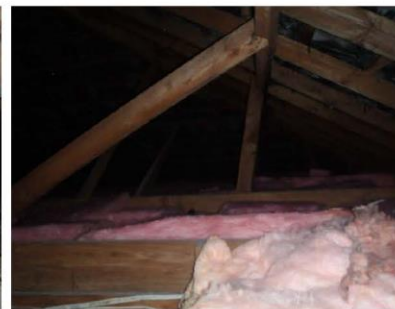
Figure 2: Timber rafters and struts
