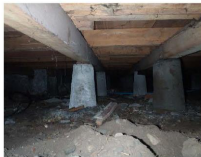
Figure 1: Precast concrete piles
