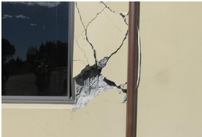
Figure 12 Cracked concrete panel
