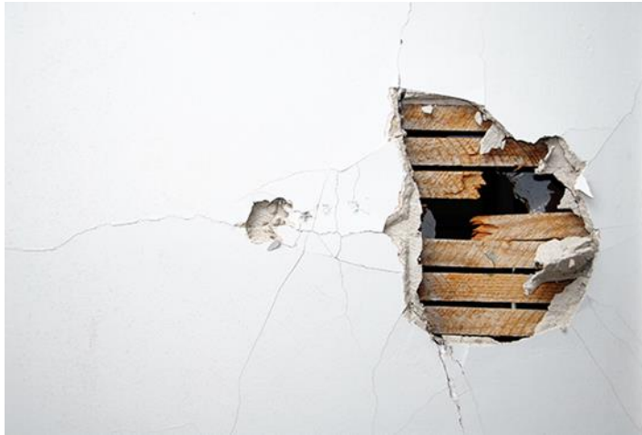
Figure 19 Cracking and detachment damage to a lath and plaster wall
