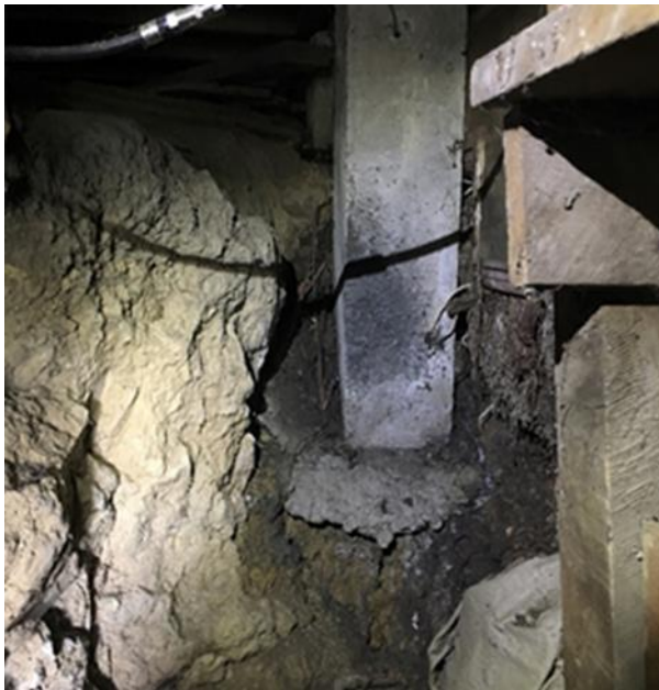
Figure 1 Pile settlement due to loss of support
