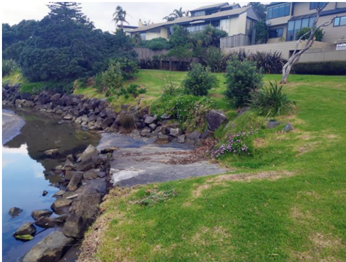
Figure 69 Riprap scour protection
