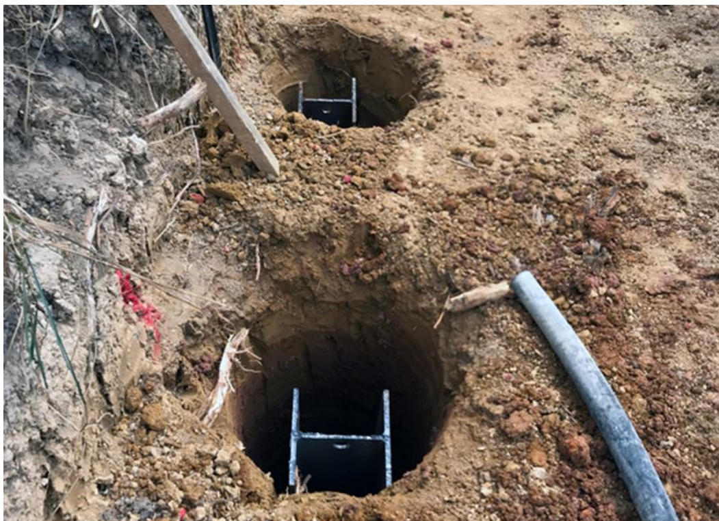
Figure 53 Reinforced concrete palisade wall holes
