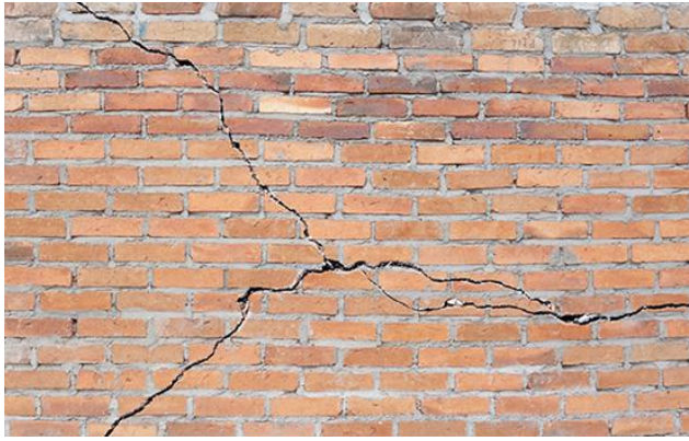
Figure 14 Severely cracked brick wall
