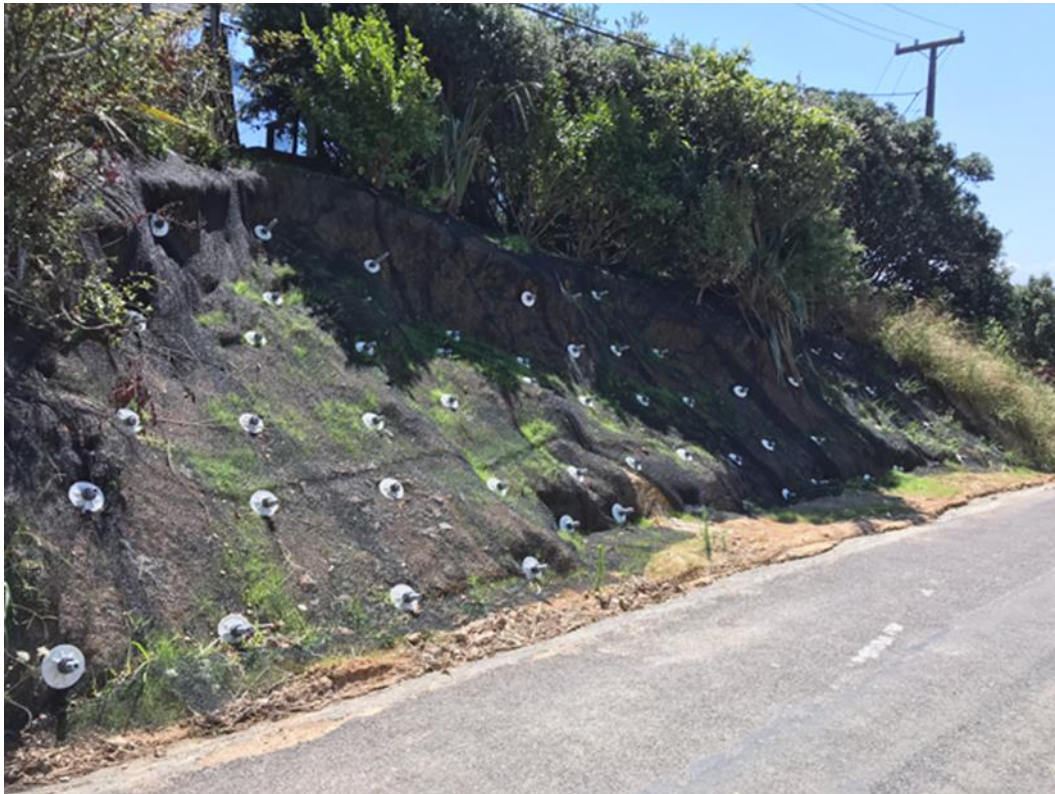
Figure 55 Soil nail retaining wall
