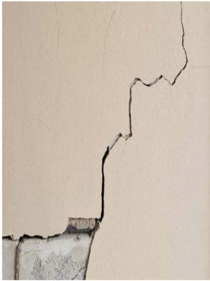
Living room – 1.5 LM structural crack in painted plasterboard intertenancy wall. EQ-related.
