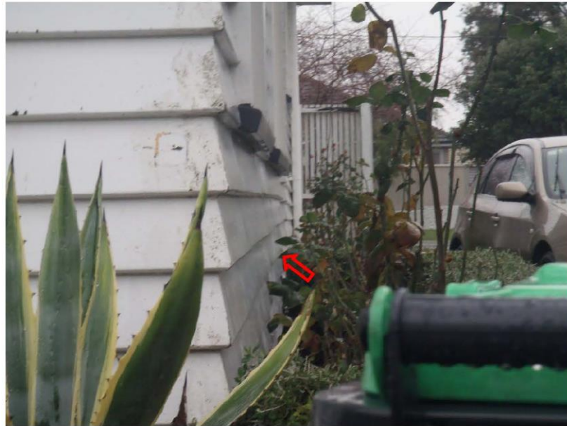
Figure 7: Timber weatherboards are visibly out of alignment
