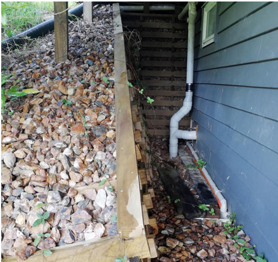
Figure 49 Timber crib retaining wall
