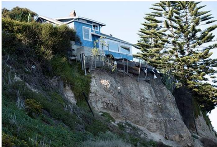
Figure 2 Landslide resulting in undermining of dwelling foundation
