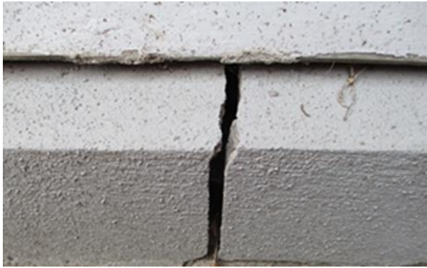
Figure 22 Cracked foundation
