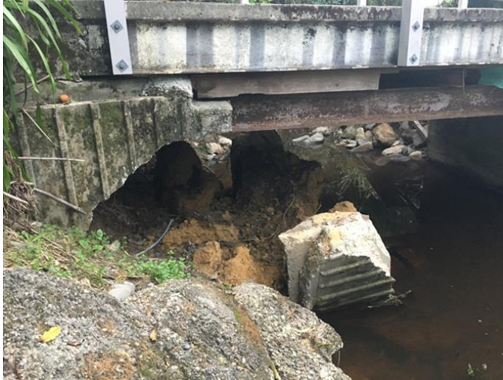
Figure 38 Impact damage to a bridge abutment from flood debris
