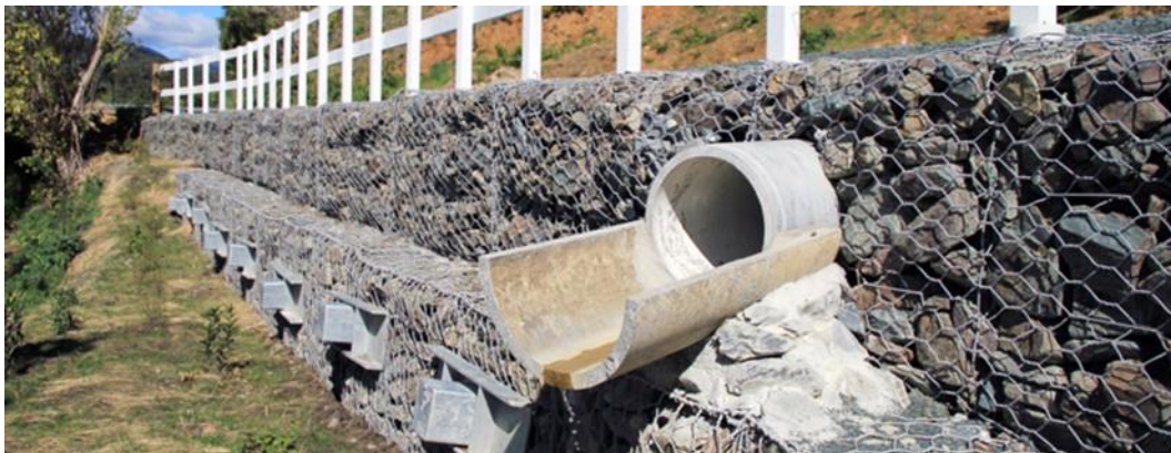
Figure 51 Gabion basket retaining wall
