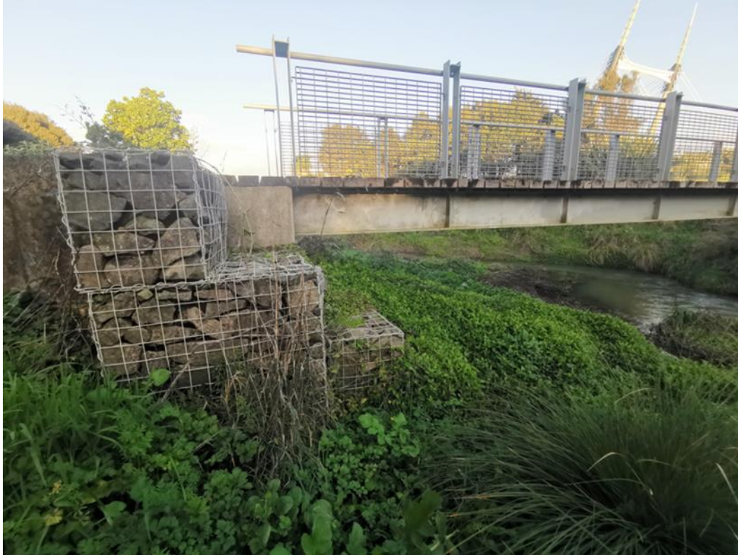
Figure 50 Gabion basket scour protection
