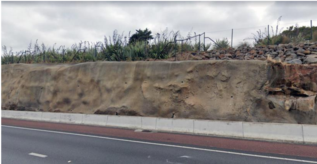
Figure 57 Sprayed concrete retaining wall
