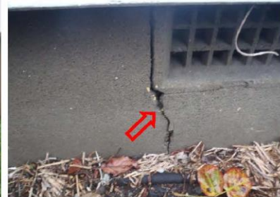
Figure 6: Old crack with paint embedment below East-facing window of dining area
