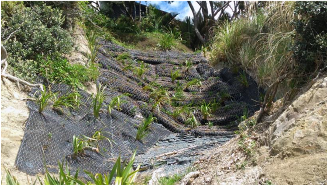
Figure 56 Pinned mesh retaining wall
