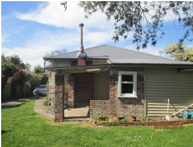
Figure 27 Disconnected flue with temporary waterproofing measures
