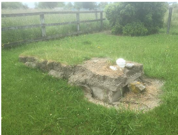
Figure 29 Displacement of septic tank
