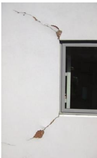
Figure 10 Cracked EIFS panel (BRANZ)
