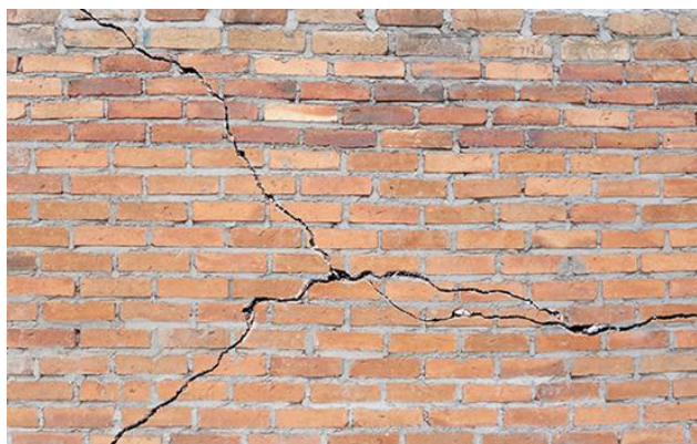
Figure 14 Severely cracked brick wall
