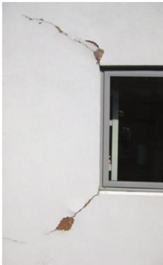
Figure 10 Cracked EIFS panel (BRANZ)
