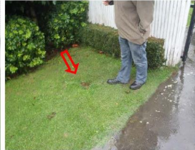
Figure 4: Depression in ground where fissure extends
