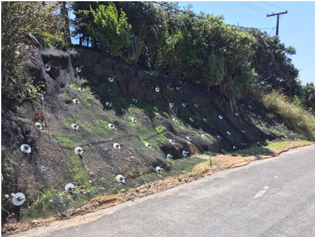
Figure 55 Soil nail retaining wall
