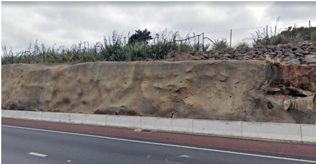
Figure 57 Sprayed concrete retaining wall
