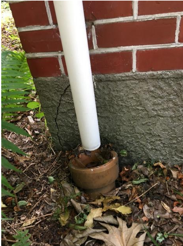
Figure 23 Cracked render finish
