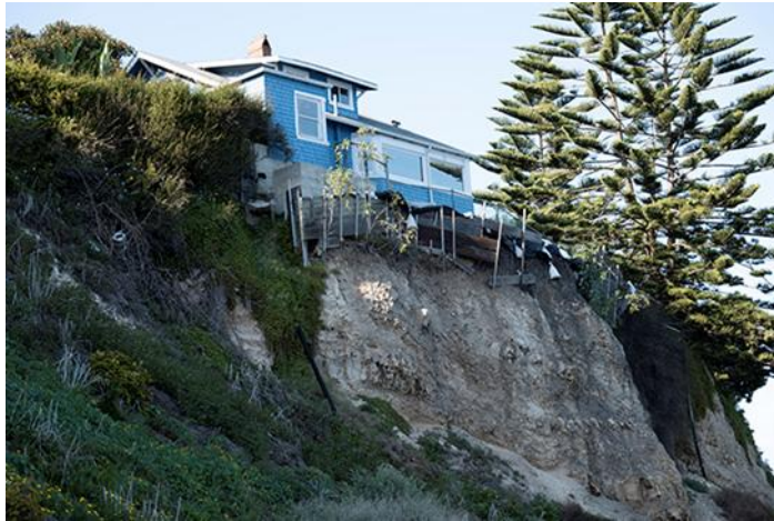
Figure 2 Landslide resulting in undermining of dwelling foundation
