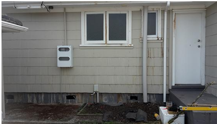
Figure 4 Heat damage to cladding from hydrothermal activity
