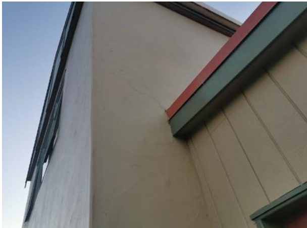
Figure 11 Cracked stucco panel
