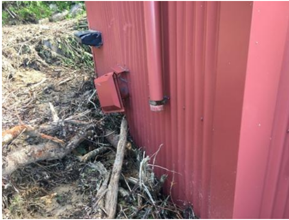
Figure 9 Impact damage to metal cladding
