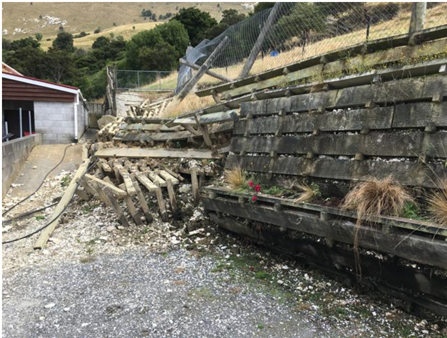
Figure 41 Timber crib retaining wall that has collapsed due to earthquake
