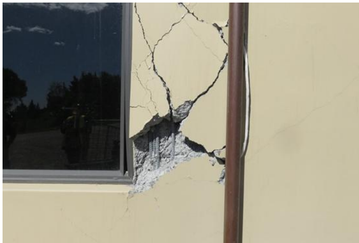
Figure 12 Cracked concrete panel
