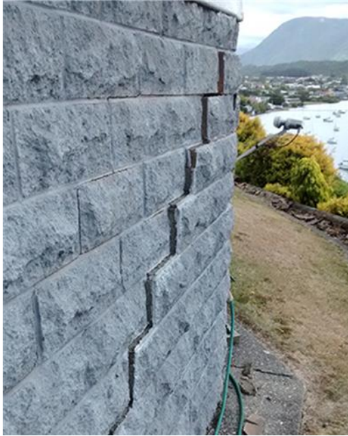
Figure 13 Step cracking to brick cladding with detachment
