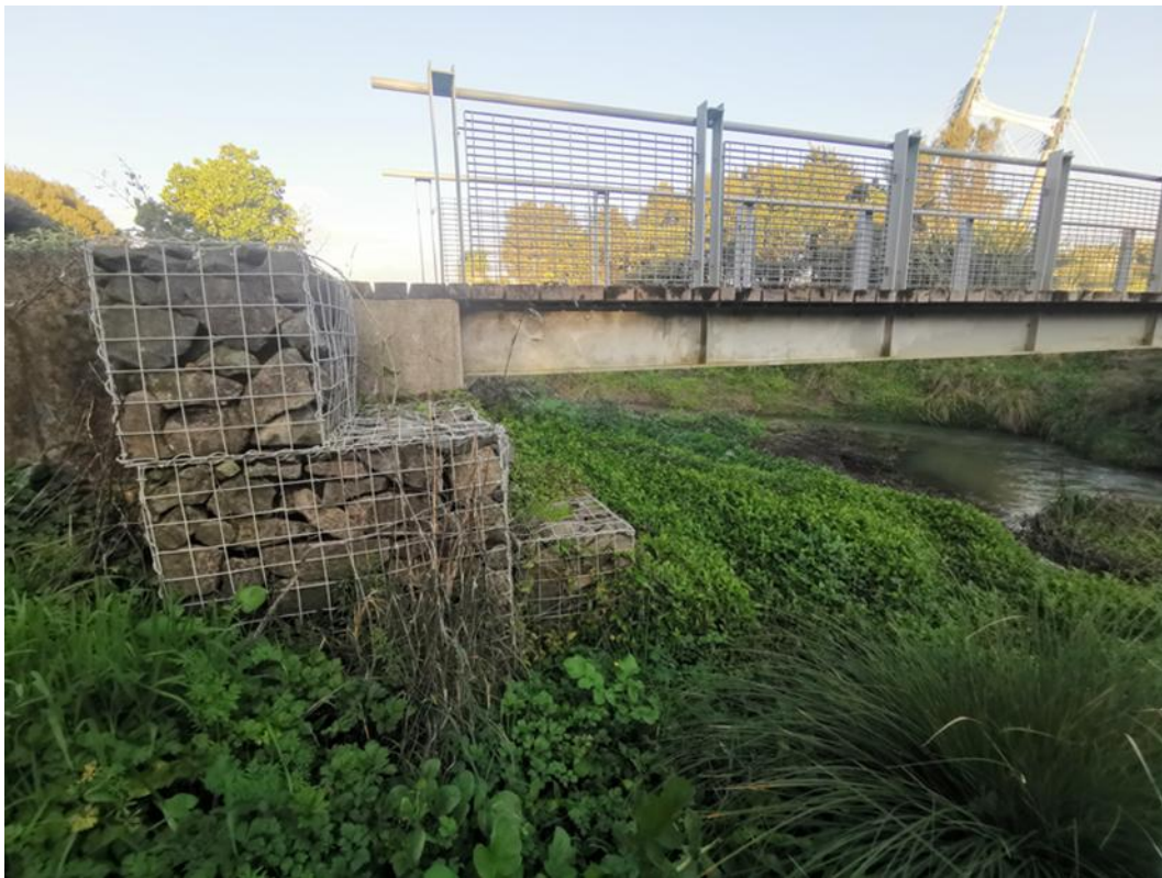
Figure 50 Gabion basket scour protection
