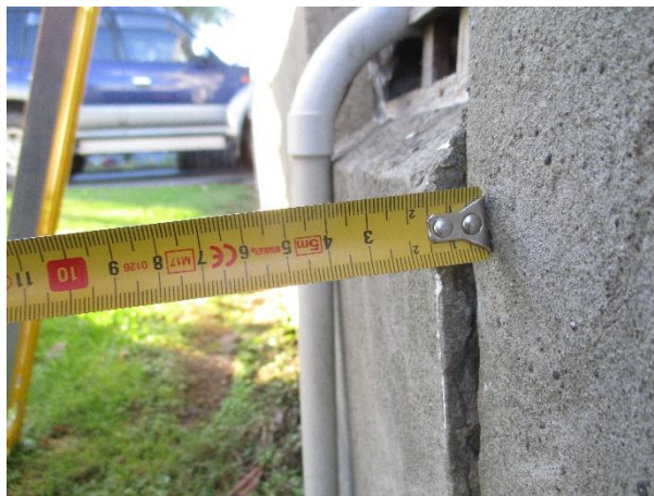
Figure 43 Out-of-plane displacement
