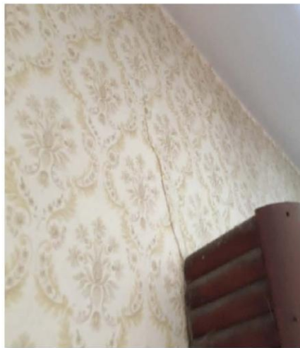
Living room - 2.0 LM structural tear / crack to wallpapered plasterboard intertenancy wall. EQ-related.
