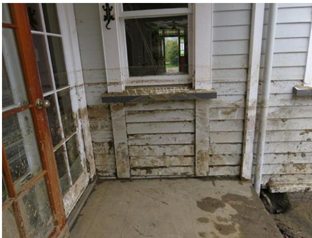
Figure 8 Moisture damage to weatherboards
