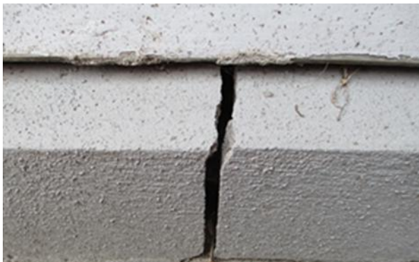
Figure 22 Cracked foundation
