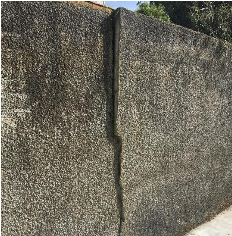
Figure 39 Retaining wall that has cracked due to earthquake
