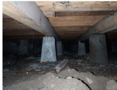
Figure 1: Precast concrete piles
