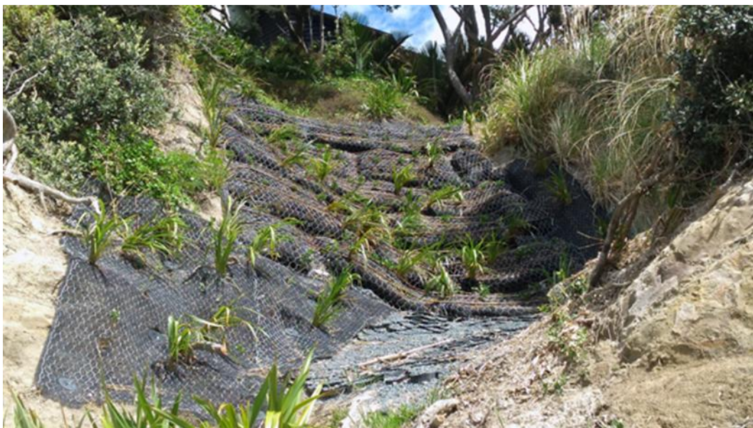
Figure 56 Pinned mesh retaining wall
