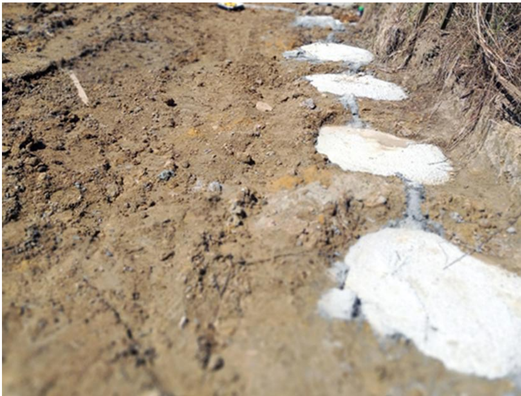
Figure 54 Reinforced concrete palisade wall – complete
