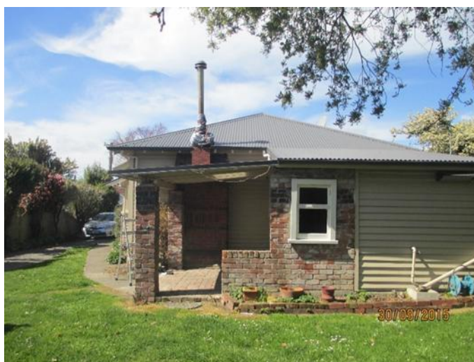
Figure 27 Disconnected flue with temporary waterproofing measures
