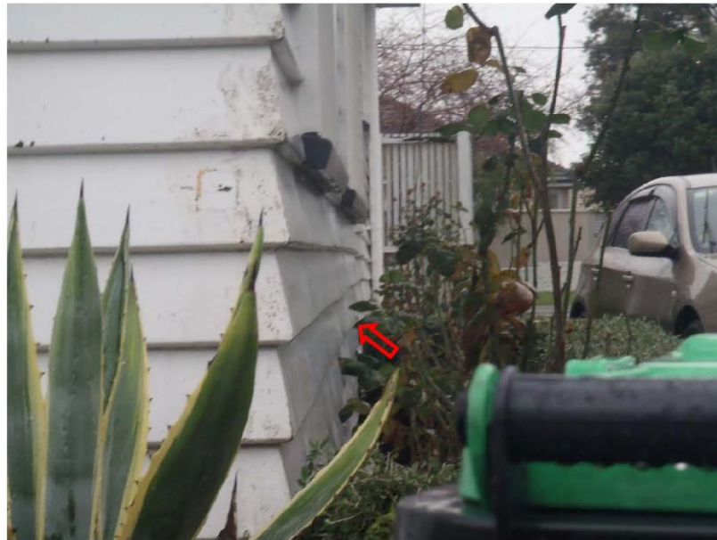
Figure 7: Timber weatherboards are visibly out of alignment
