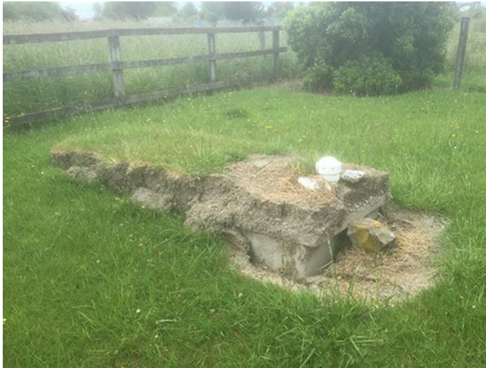
Figure 29 Displacement of septic tank
