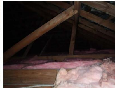
Figure 2: Timber rafters and struts
