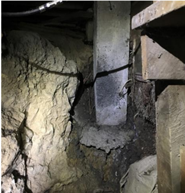
Figure 1 Pile settlement due to loss of support
