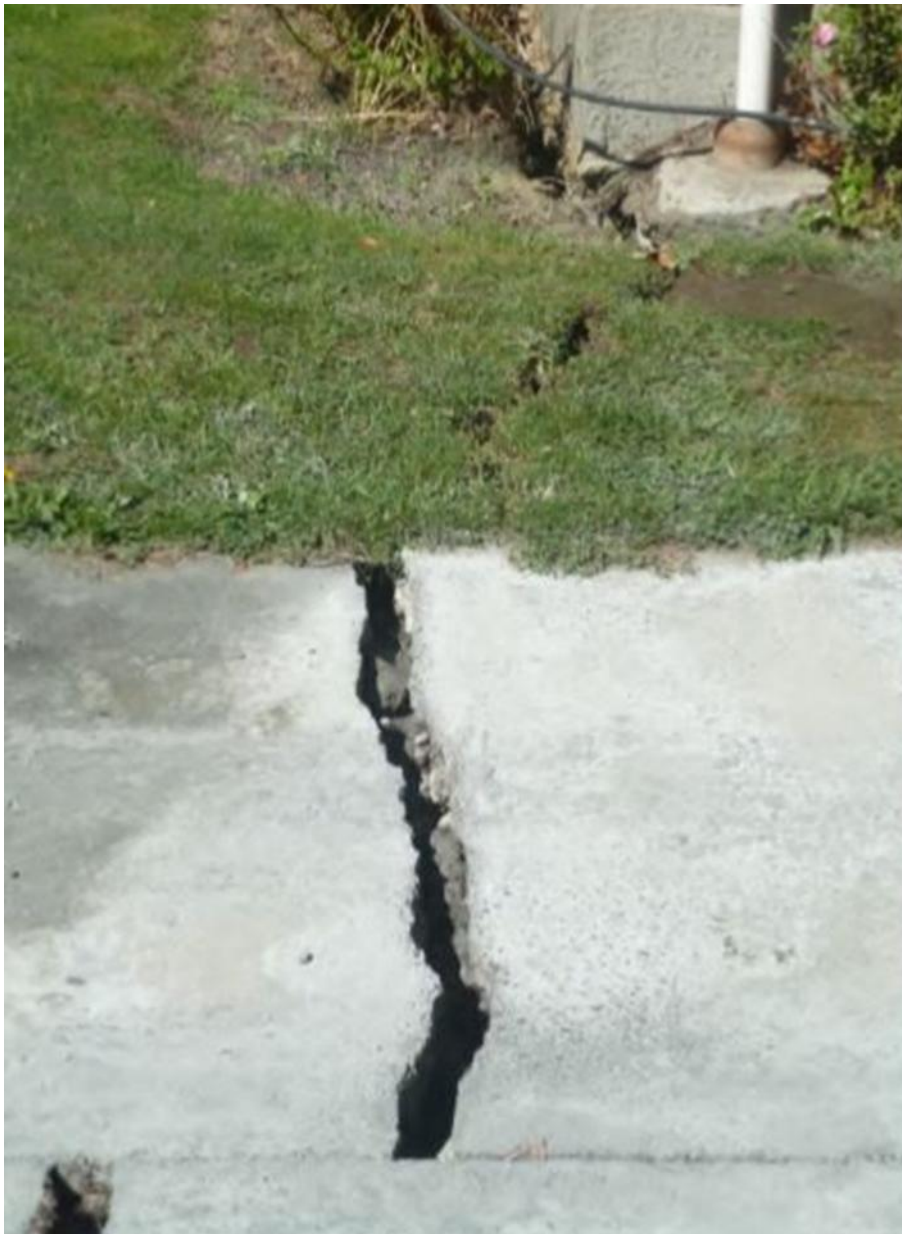
Figure 33 Cracking (oscillation movement of dwelling) due to earthquake
