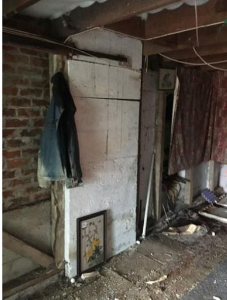
Figure 28 Pre-cast chimney
