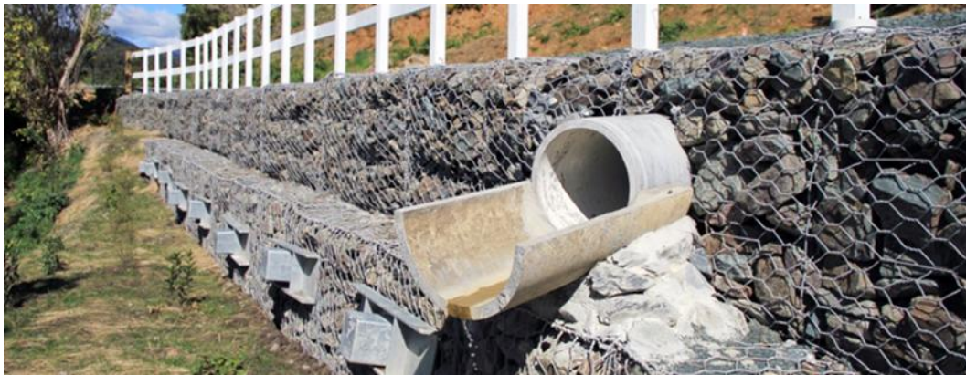
Figure 51 Gabion basket retaining wall
