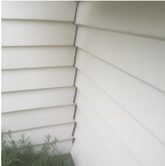
Figure 7 Weatherboard movement and cracking
