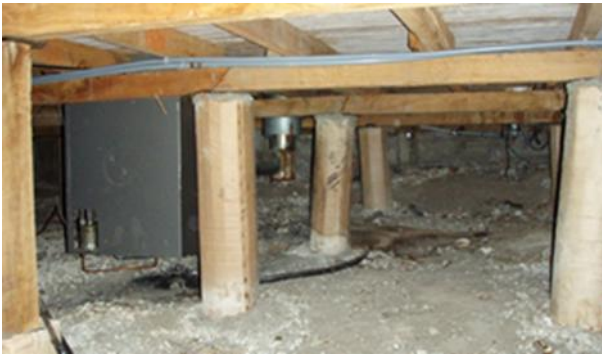
Figure 21 Pile detachment and rotation
