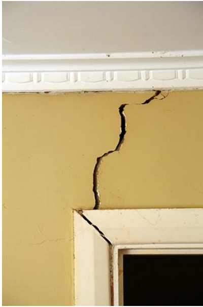
Figure 17 Structural cracking
