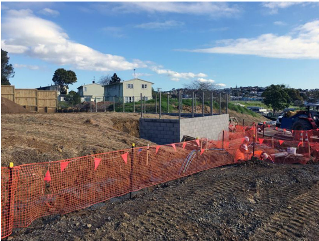
Figure 52 Concrete block retaining wall
