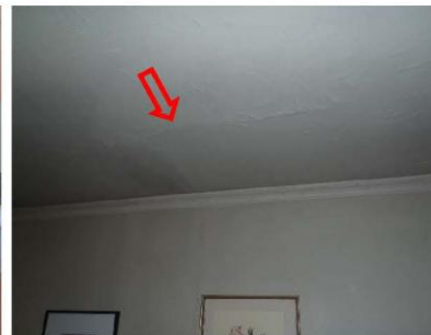
Figure 9: Ceiling crack in living area
