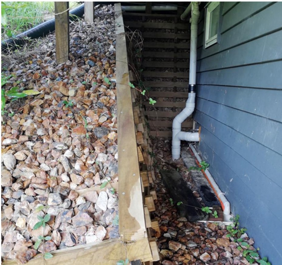
Figure 49 Timber crib retaining wall
