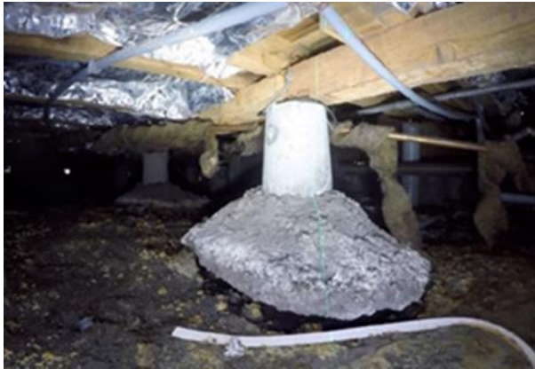
Figure 20 Loss of support resulting in settlement
