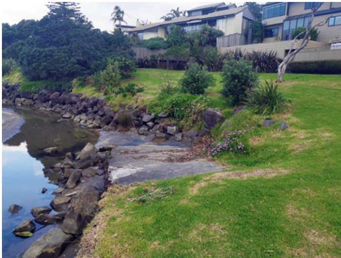
Figure 69 Riprap scour protection
