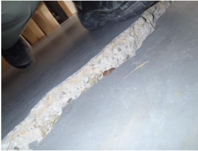
Figure 24 Cracking with vertical displacement
