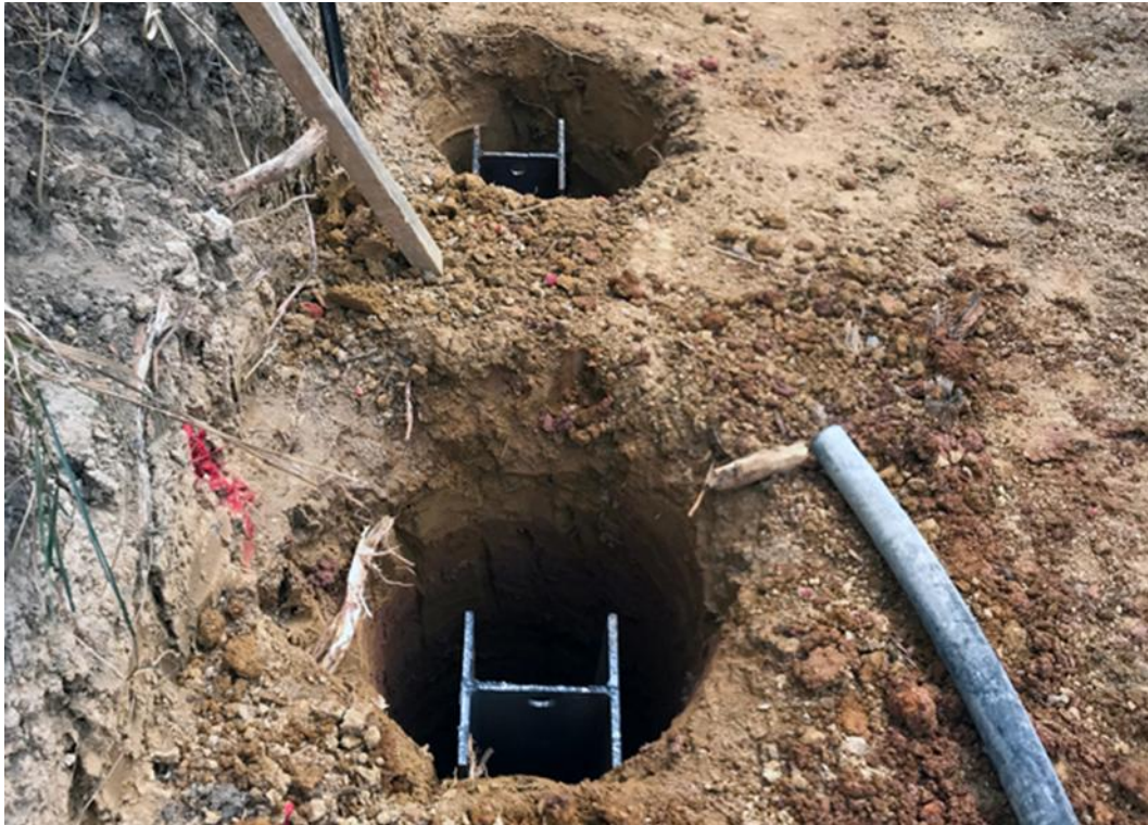
Figure 53 Reinforced concrete palisade wall holes
