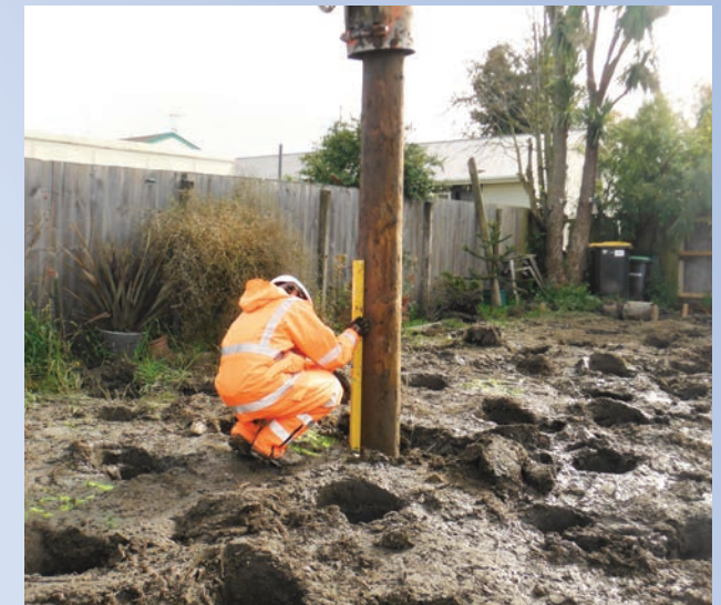
Construction of driven timber poles
