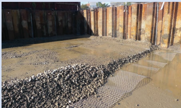
Reinforced Gravel Raft – geogrid and gravel installation
