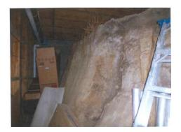
[99] In his view, the landslip was a combination of a rotational and translational landslip that resulted in a saturated debris flow down the slope below. It was triggered
