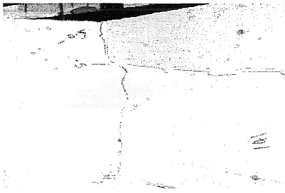
(i) North side cracks pattern
