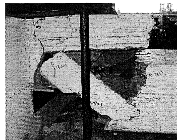
(iii) Floor unit at failure
