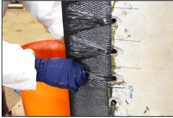
(g) Installing FRP spike anchors
