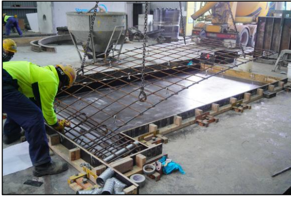
(a) Reinforcement into formwork
