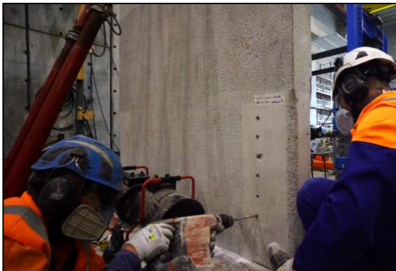
(c) Drilling holes to install FRP spike anchors
