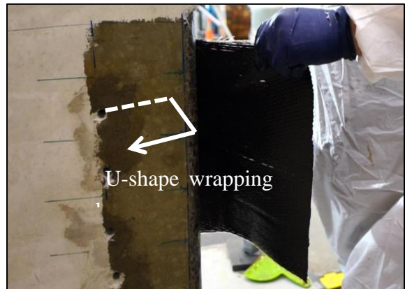
(f) Wrapping the U-shape FRP laminate
