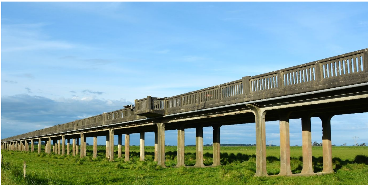
Figure 1: The Whirokino Trestle Bridge in Foxton, NZ prior to demolition.
