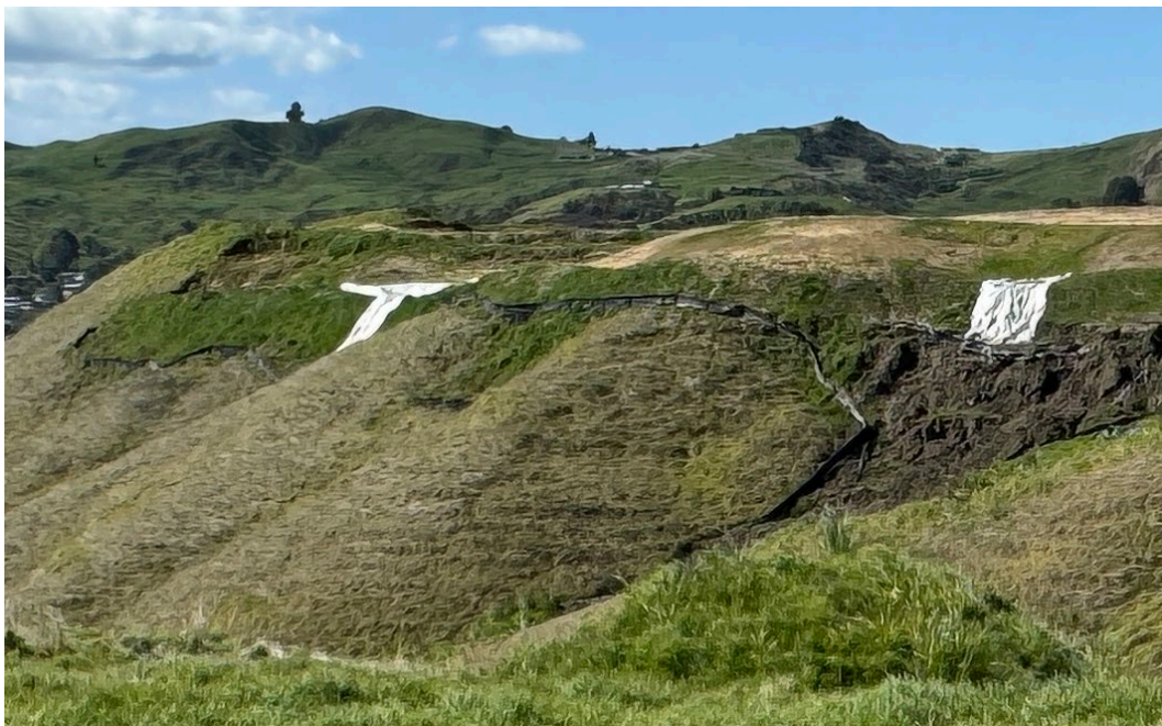
Figure 14: Edge of Pleistocene Mangatuna Fm plateau with Miocene Tolaga Gp below. These plateau remnants are highly unstable, as the Pleistocene soils become saturated and slump over the underlying impermeable mudstones.
