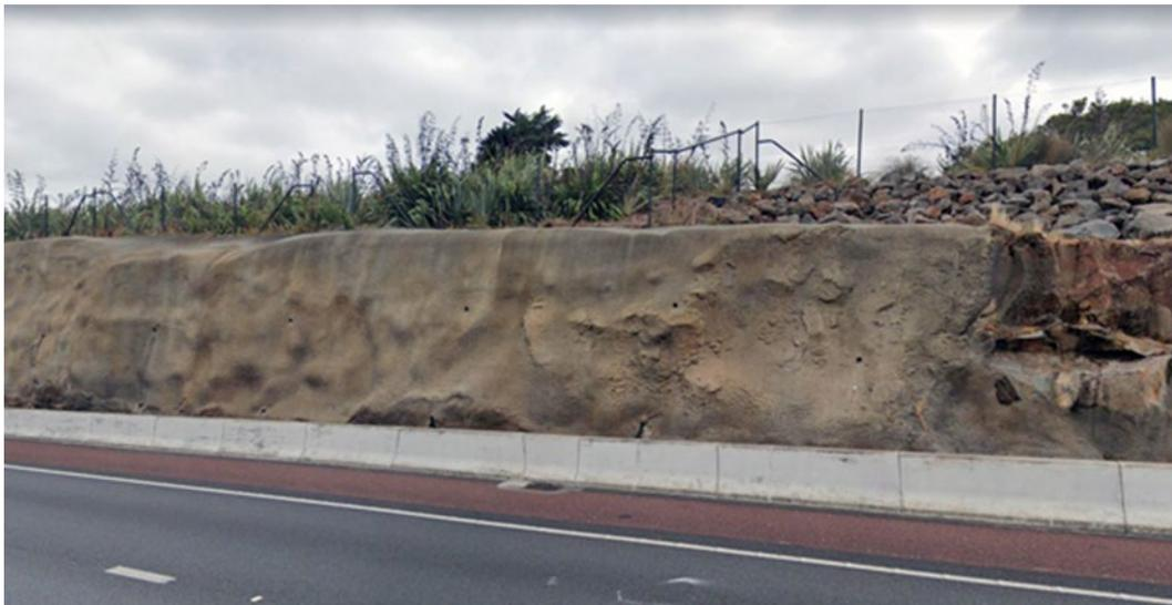
Figure 56 Sprayed concrete retaining wall
