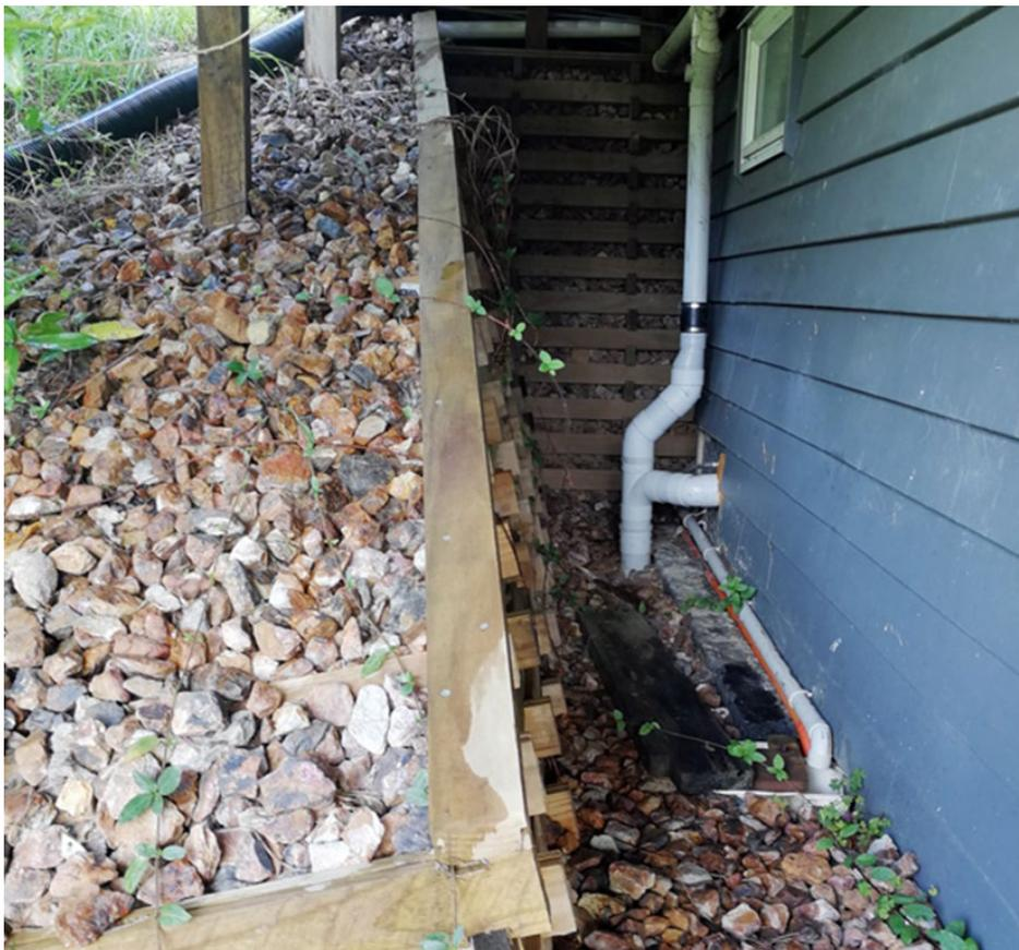
Figure 50 Timber crib retaining wall
