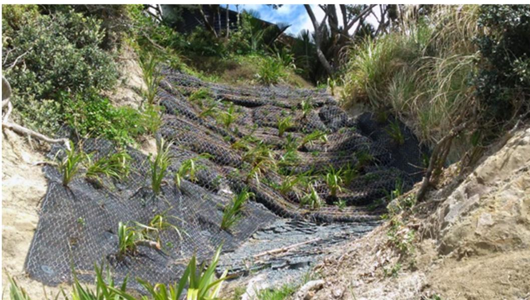
Figure 57 Pinned mesh retaining wall
