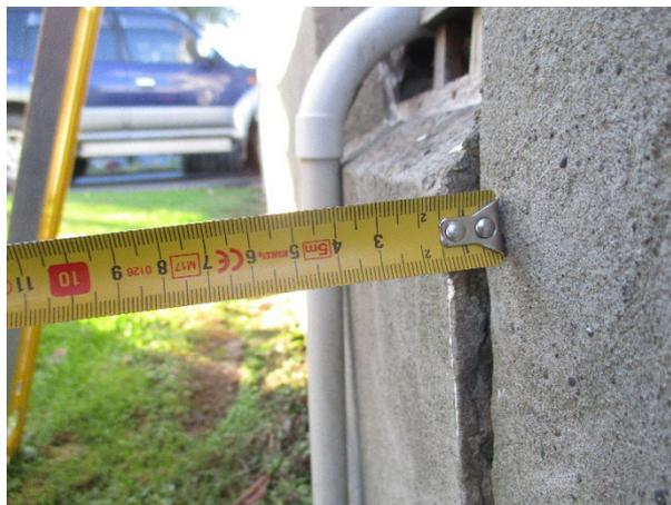
Figure 44 Out-of-plane displacement
