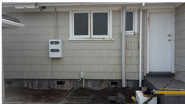
Figure 4 Heat damage to cladding from hydrothermal activity
