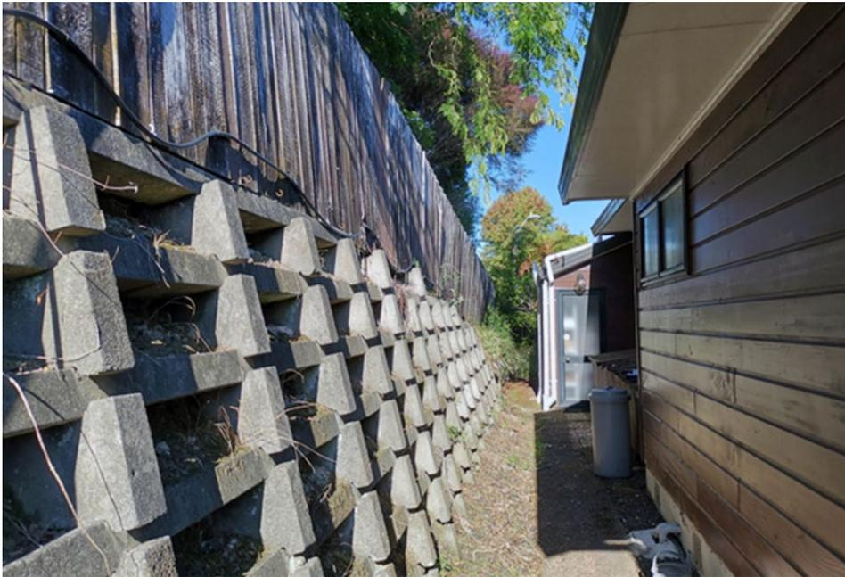
Figure 49 Concrete crib retaining wall
