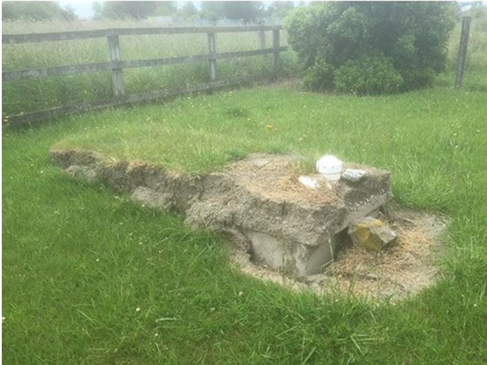
Figure 29 Displacement of septic tank
