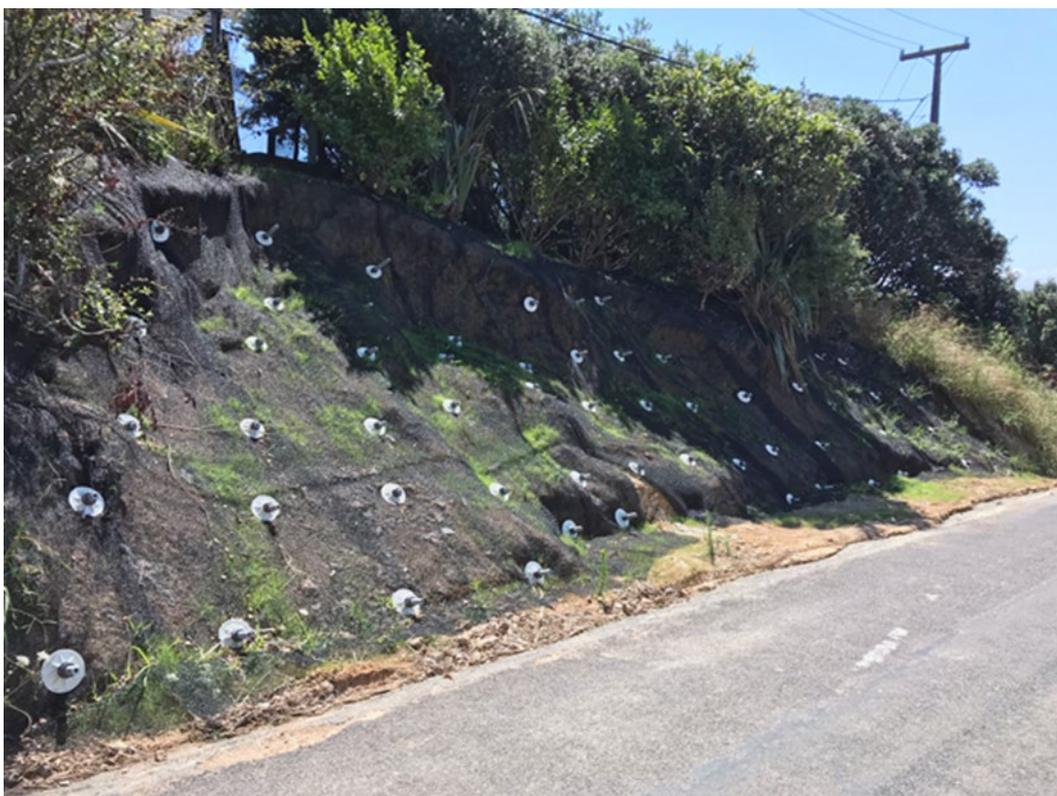
Figure 58 Soil nail retaining wall
