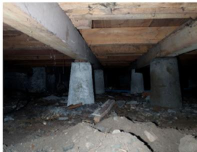
Figure 1: Precast concrete piles
