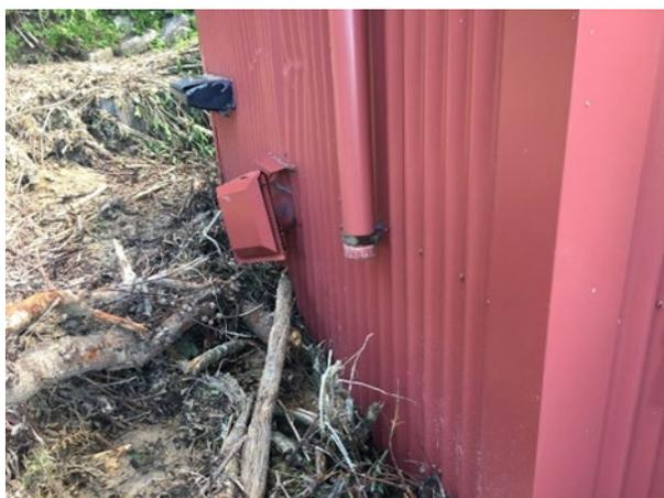
Figure 9 Impact damage to metal cladding
