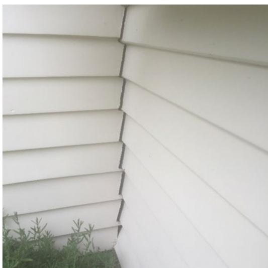
Figure 7 Weatherboard movement and cracking
