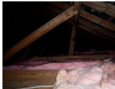
Figure 2: Timber rafters and struts
