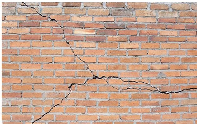
Figure 14 Severely cracked brick wall
