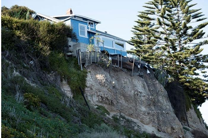
Figure 2 Natural landslide resulting in undermining of dwelling foundation
