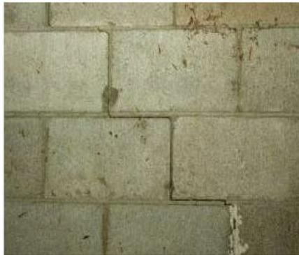
Living room – Adjoining intertenancy concrete block wall with Unit 2 – 1.0 LM step crack in wall mortar. EQ-related.
