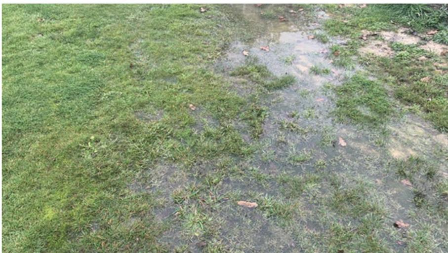
Figure 36 Localised ponding due to earthquake
