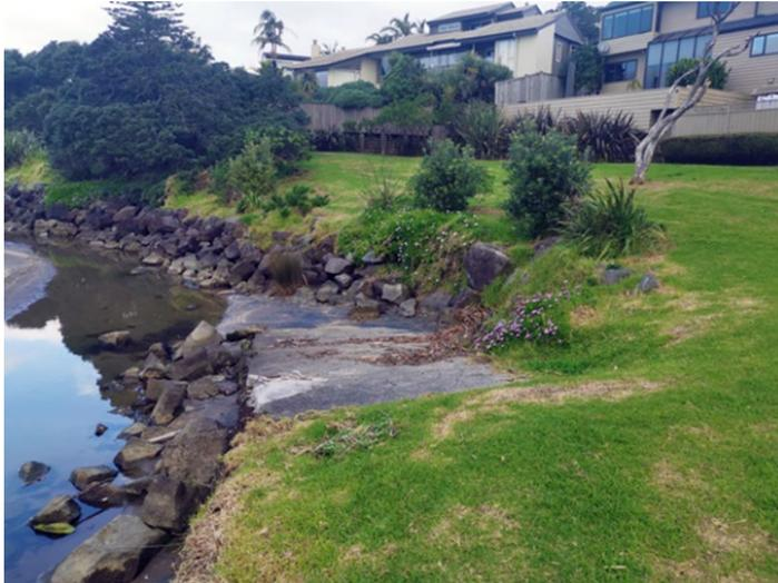
Figure 70 Riprap scour protection
