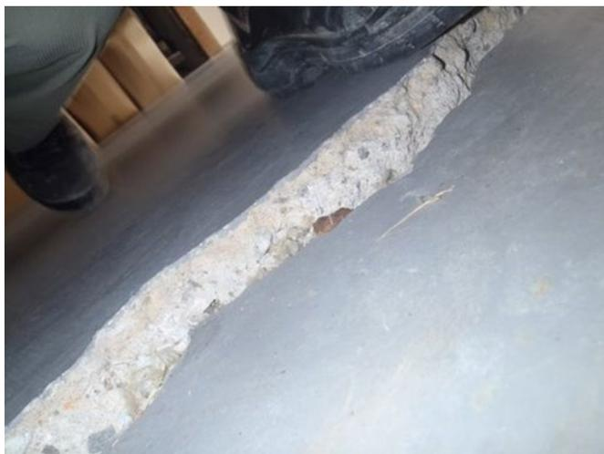
Figure 24 Cracking with vertical displacement
