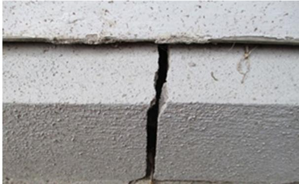
Figure 22 Cracked foundation
