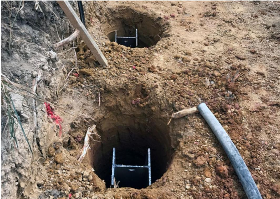
Figure 54 Reinforced concrete palisade wall holes
