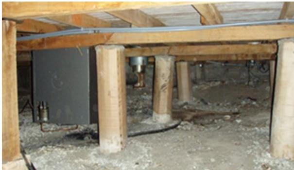
Figure 21 Pile detachment and rotation
