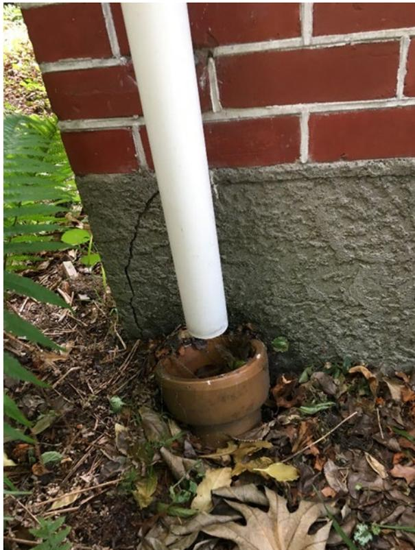
Figure 23 Cracked render finish
