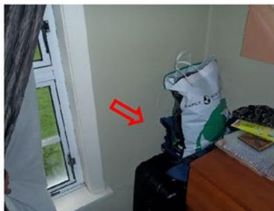
Figure 8: Diagonal wall lining crack in Bedroom 3
