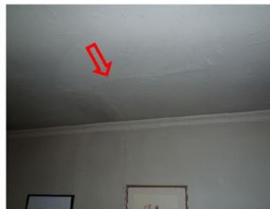
Figure 9: Ceiling crack in living area
