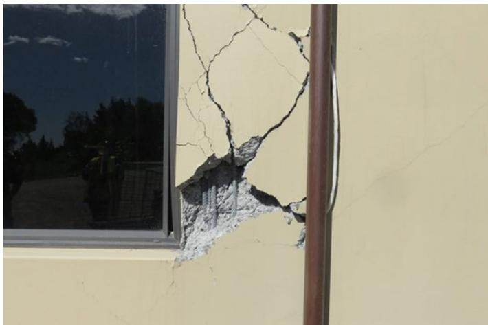
Figure 12 Cracked concrete panel
