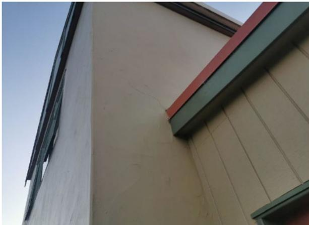
Figure 11 Cracked stucco panel
