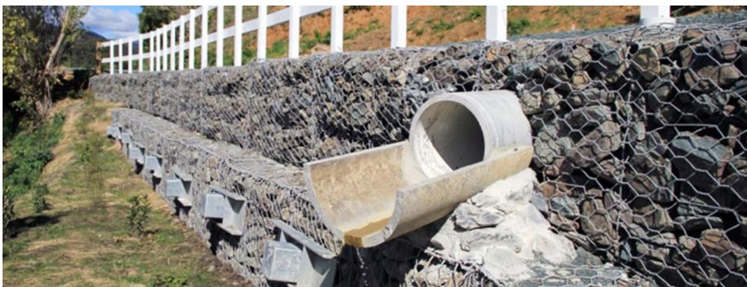
Figure 52 Gabion basket retaining wall
