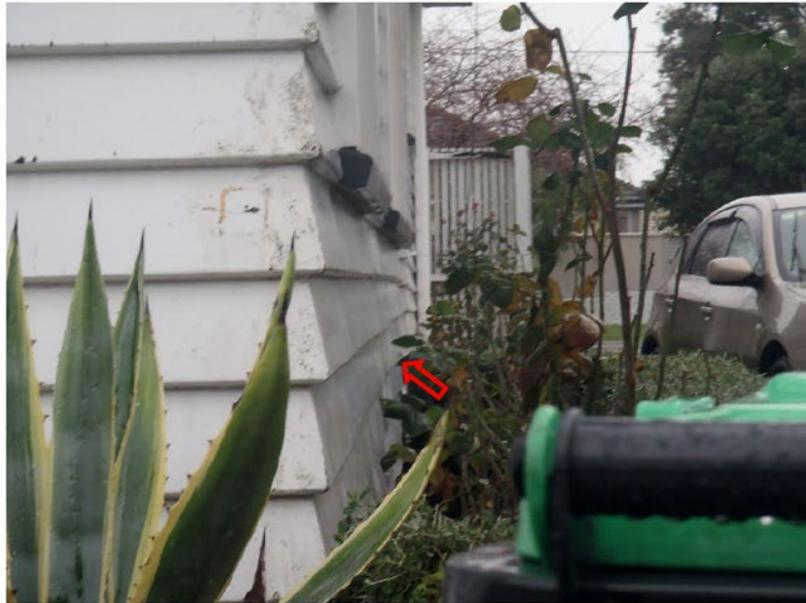
Figure 7: Timber weatherboards are visibly out of alignment
