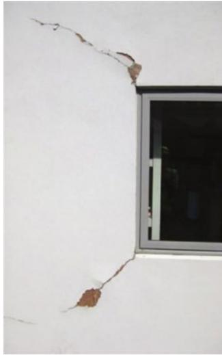
Figure 10 Cracked EIFS panel (BRANZ)
