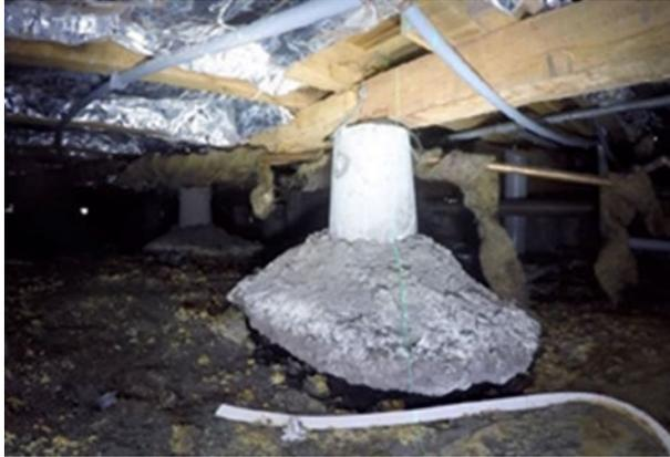
Figure 20 Loss of support resulting in settlement
