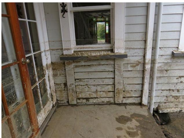
Figure 8 Moisture damage to weatherboards
