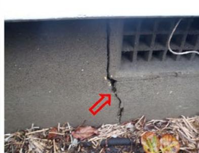
Figure 6: Old crack with paint embedment below East-facing window of dining area
