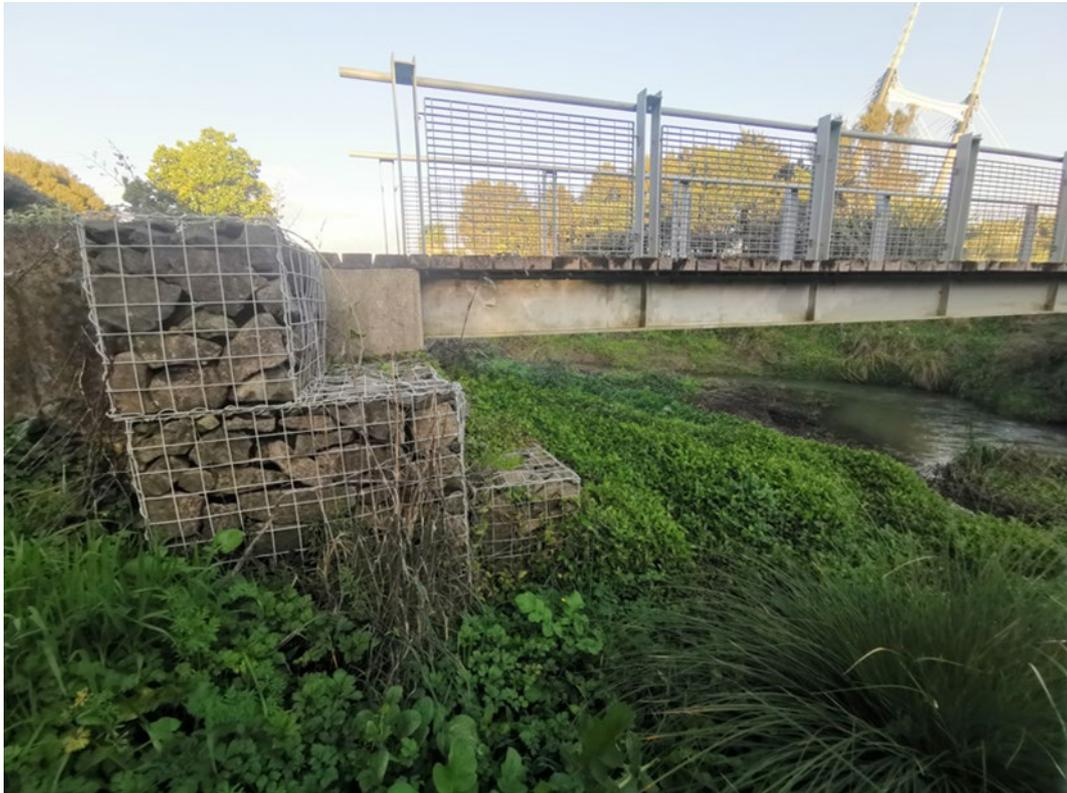
Figure 51 Gabion basket scour protection
