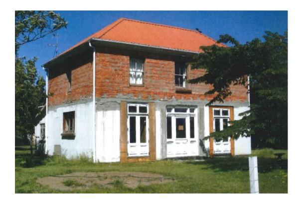
[3] The ground floor of the house was built in the 1860s. The ground floor walls of the house are made of unreinforced concrete. The first floor was added around 1897. Beams of hardwood were placed on top of the concrete walls. On top of those beams, the walls were double brick.
