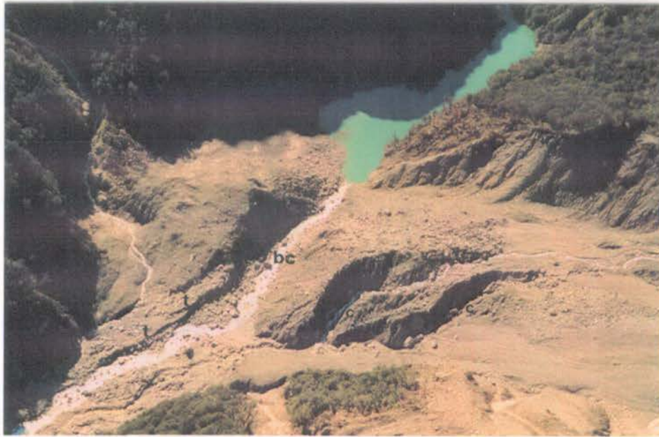
Fig. 5 Poerua landslide dam after failure, October 1999 (Hancox et al , 1999)
