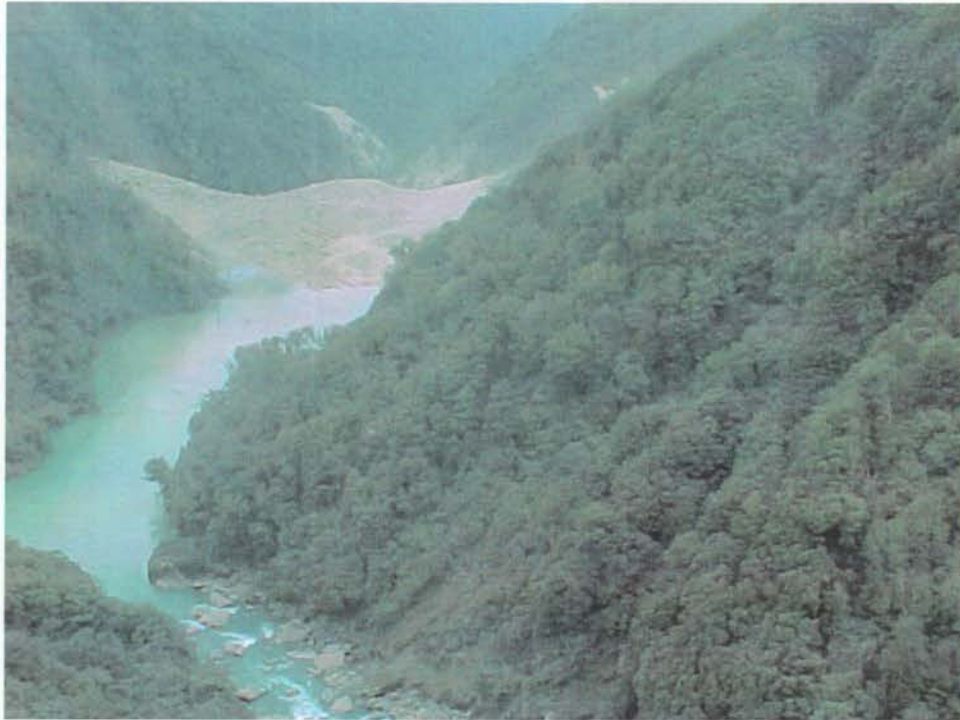
Fig. 3 Poerua landslide dam before overtopping; looking downstream. (R Daniel Westland District Council)
