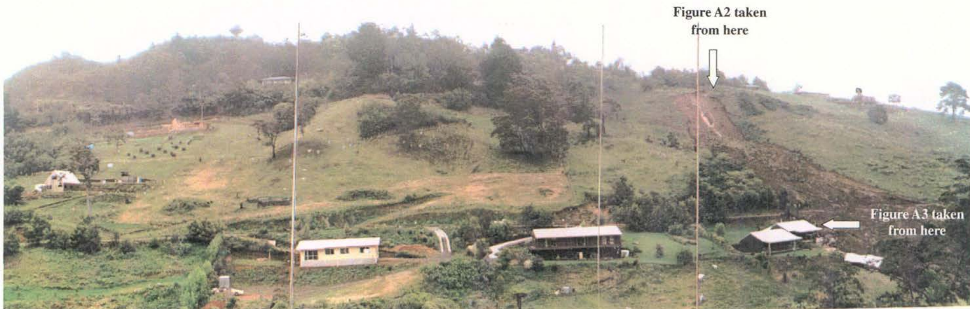
Figure A1: Landslide of 7th December 1983, damaged house on right of photo (view looking southwest)
