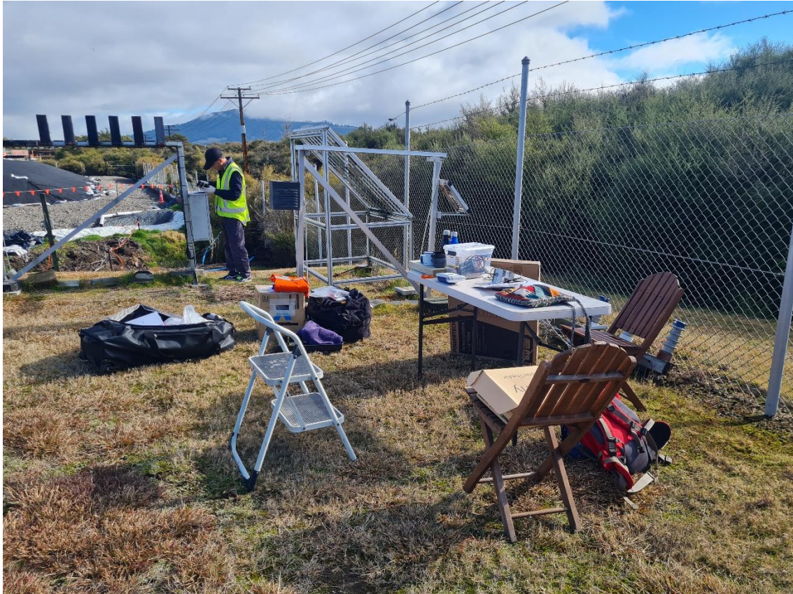
Figure 3 View of WWTP deployment site
