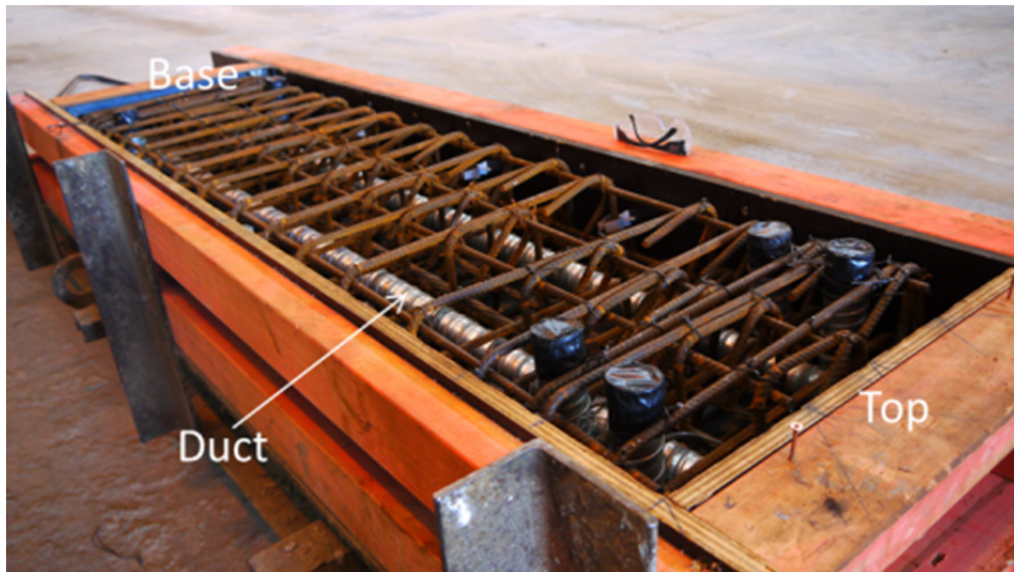
(a) Vertical ducts for PT bars
