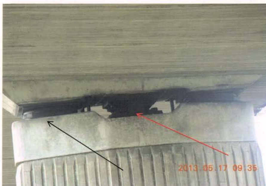
Figure 6.11. TETRON SE bearing (black arrow) and shear key (red arrow).
