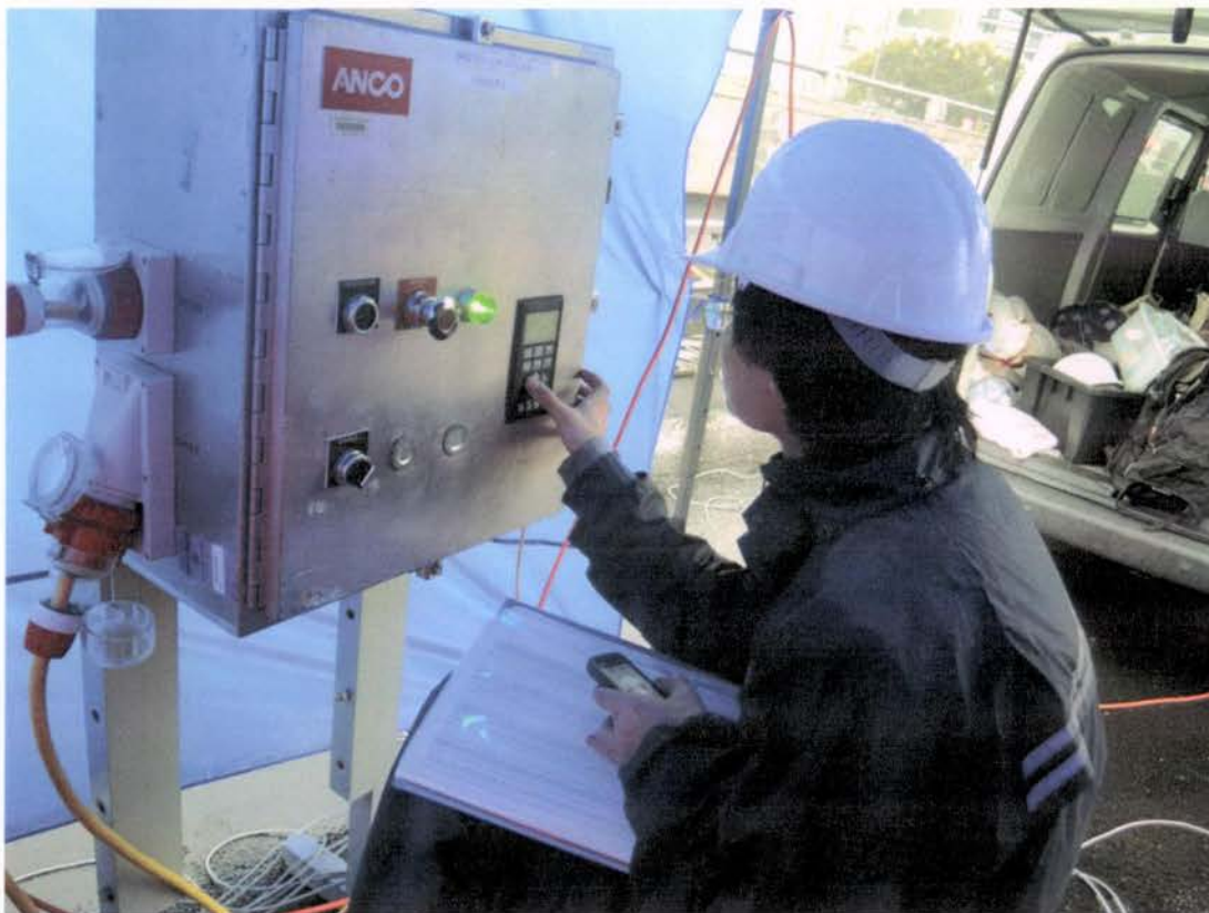
Figure 6.49. Danfoss VLT-5011 variable frequency drive control system.
