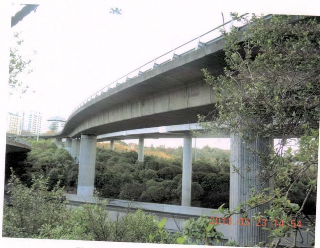
Figure 6.3. Side view of Nelson St off-ramp bridge.
