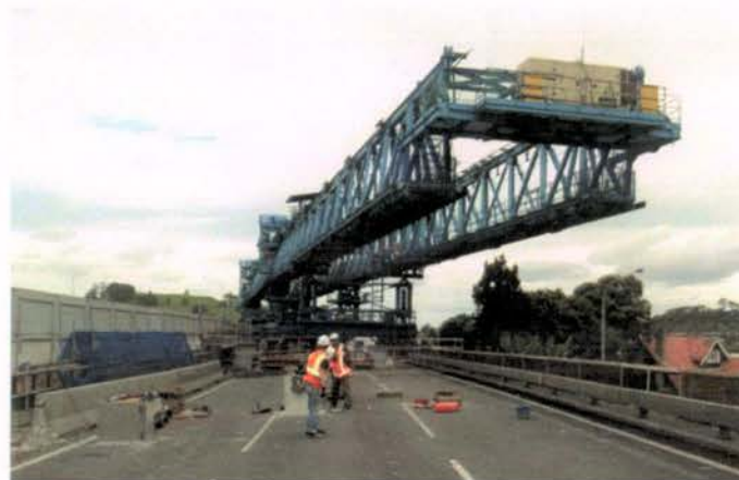
Figure 7.9. View of the deck with vertical shaker on the left and horizontal shaker in the centre, and blue demolition gantry in the foreground.
