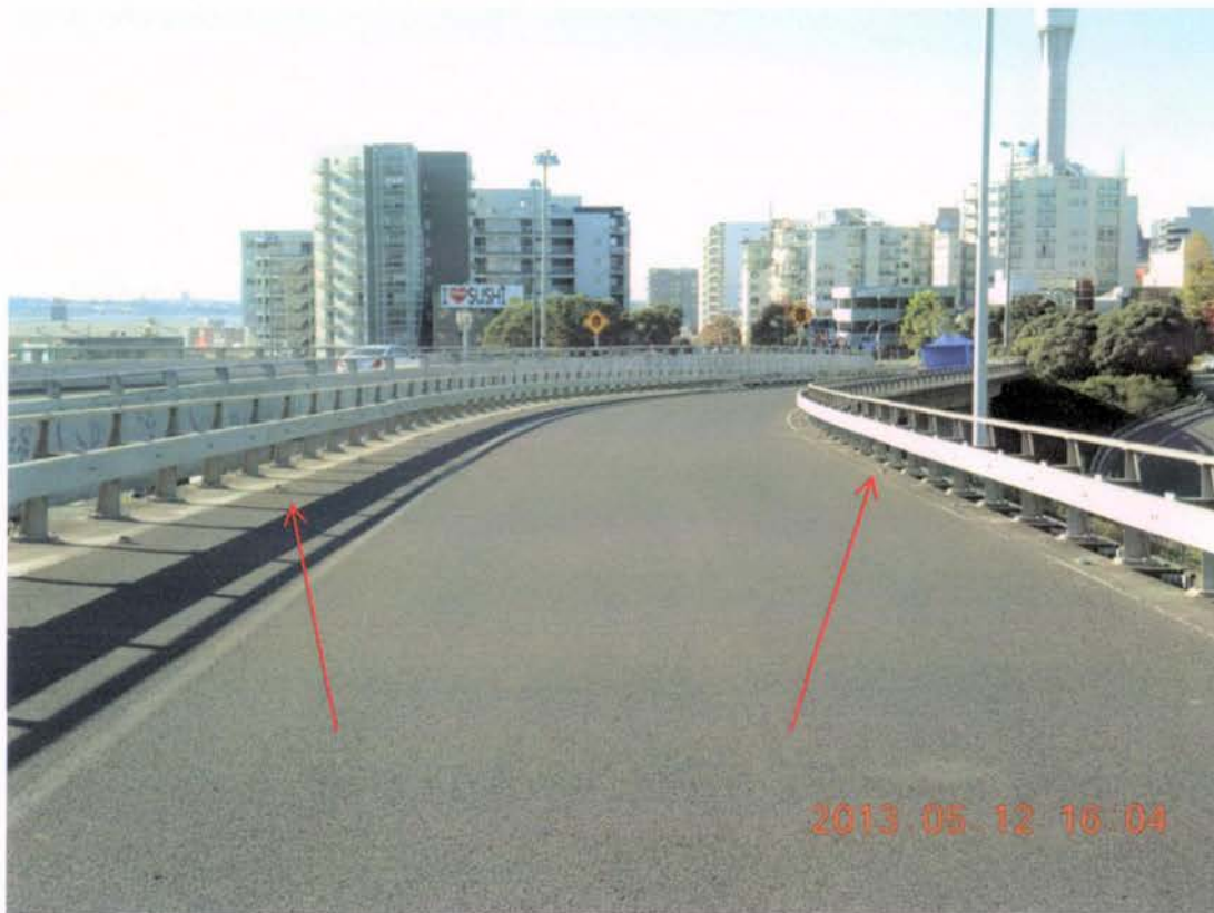
Figure 6.46. USB accelerometer arranged along both bridge curbs.
