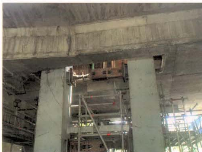
Figure 7.4. Steel towers for demolition gantry penetrating through the deck.
