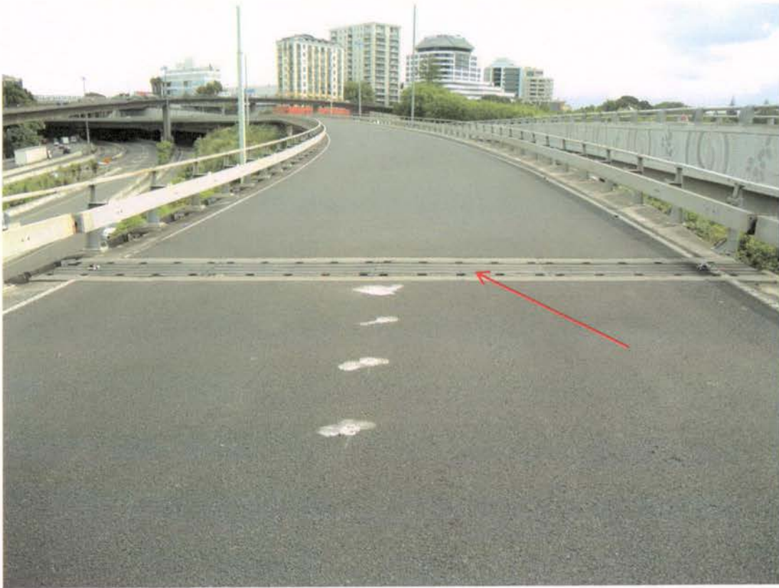
Figure 6.7. Hinge connection as seen on the bridge deck.
