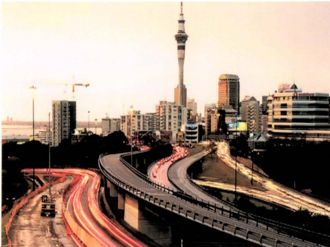
Figure 6.1. Aerial view of Nelson St off-ramp bridge.
