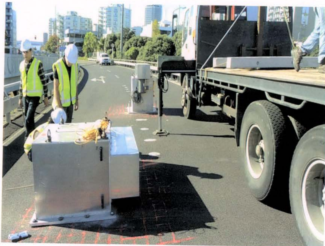
Figure 6.42. Two shakers anchored to the bridge deck.
