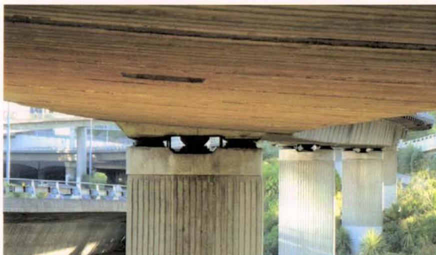
Figure 6.10. Bearing support on piers.
