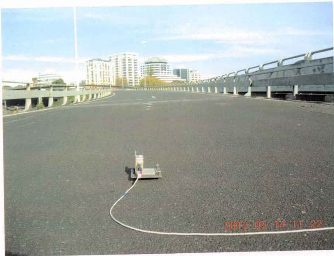
Figure 6.47. Wired accelerometers installed along centreline of the bridge deck.
