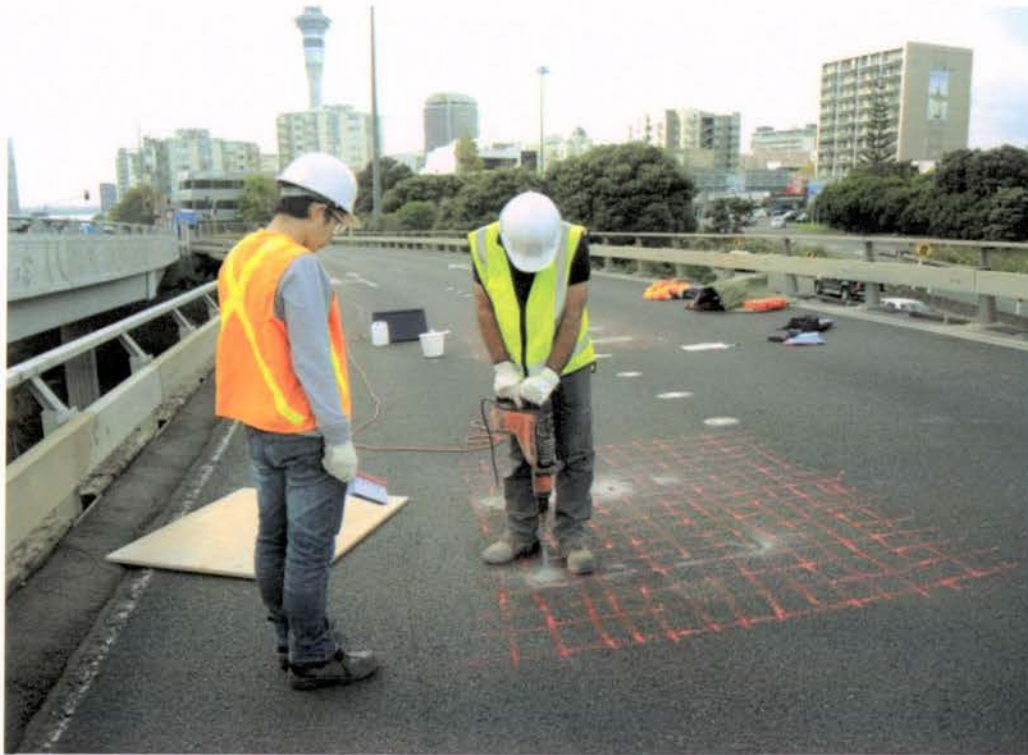
Figure 6.33. Drilling holes by using rotary hammer.
