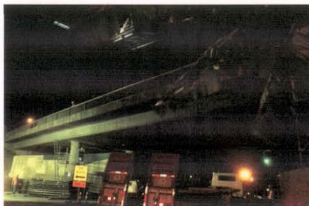
Figure 7.1. Side view of Gillies Avenue overbridge.
