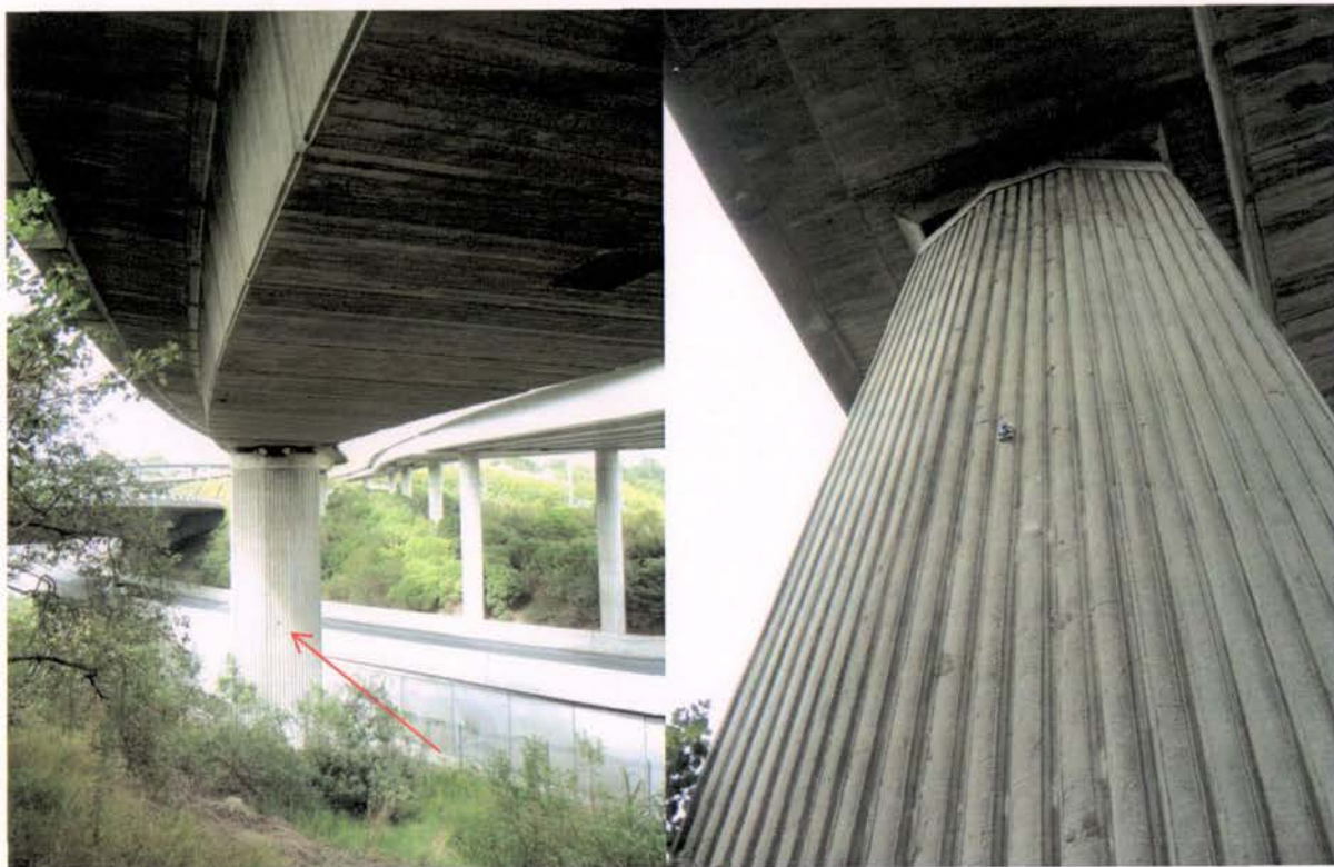
Figure 6.13. USB accelerometer installed on bridge pier.
