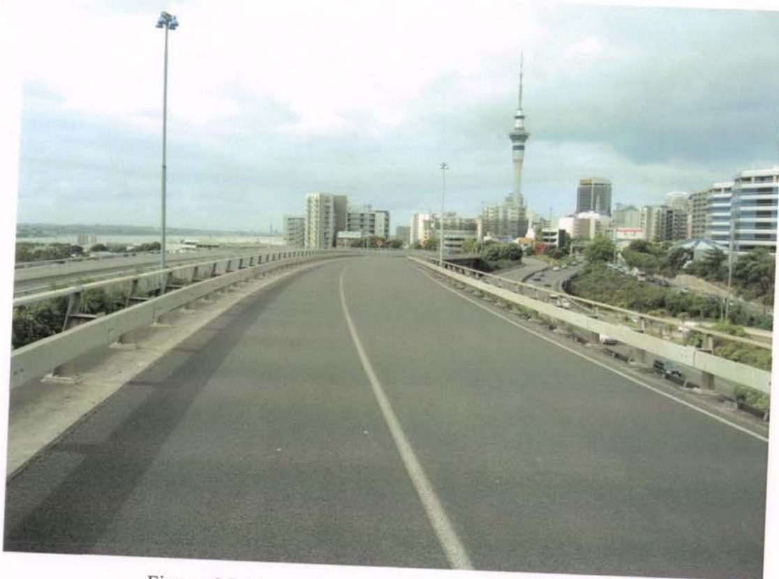
Figure 6.2. Front view of Nelson St off-ramp bridge.
