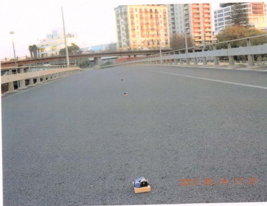
Figure 6.48. USB accelerometers installed along centreline of the bridge deck.
