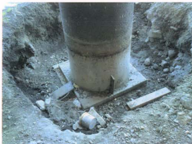
Figure 7.5. Partially excavated column foundation.
