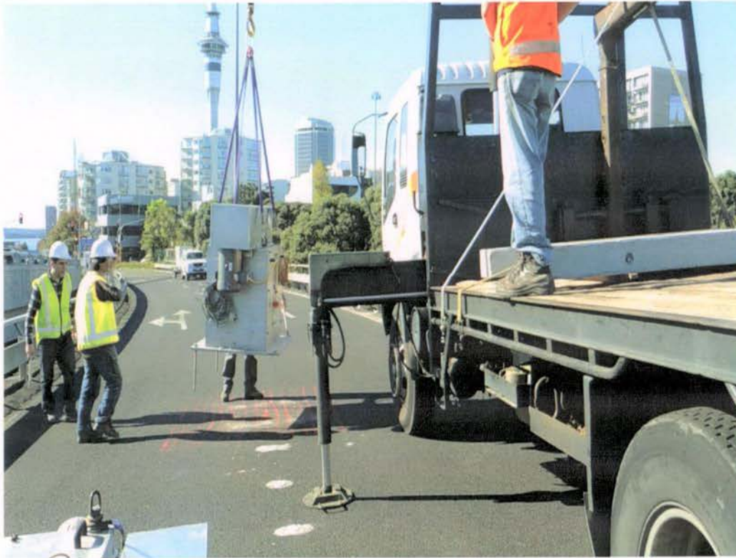
Figure 6.35. Placing shakers with the help of hiab truck.
