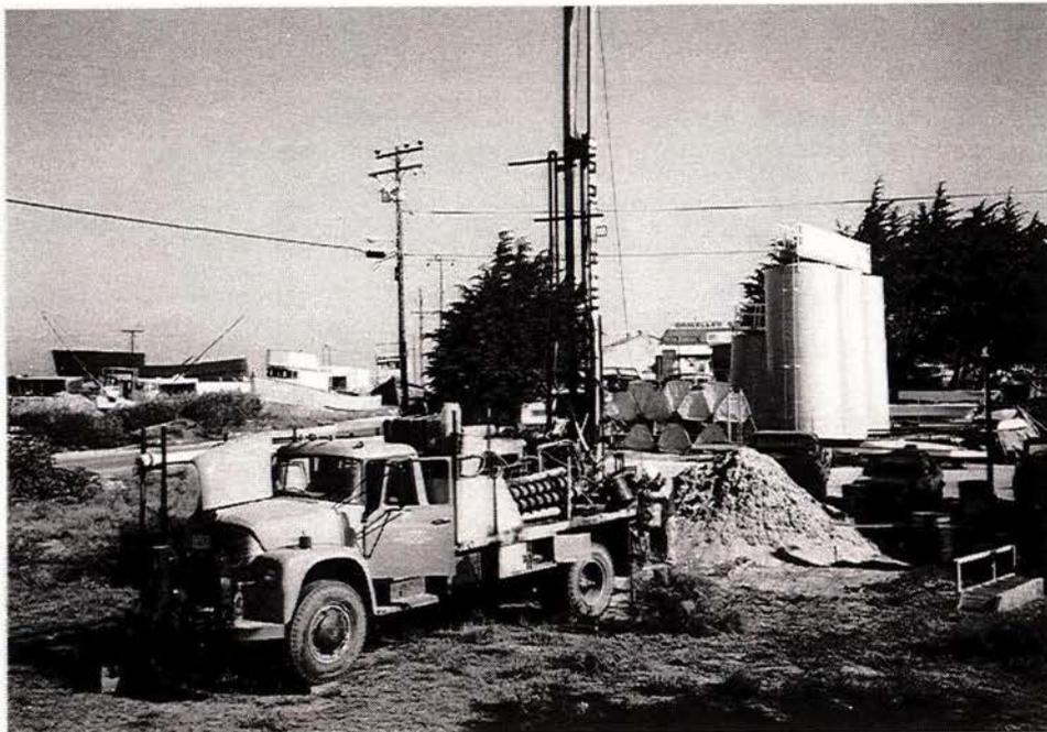
Figure 2.4 Moss Landing test site, viewed NW (SPT in progress). The oil tanks in the background underwent a foundation failure during the earthquake.
