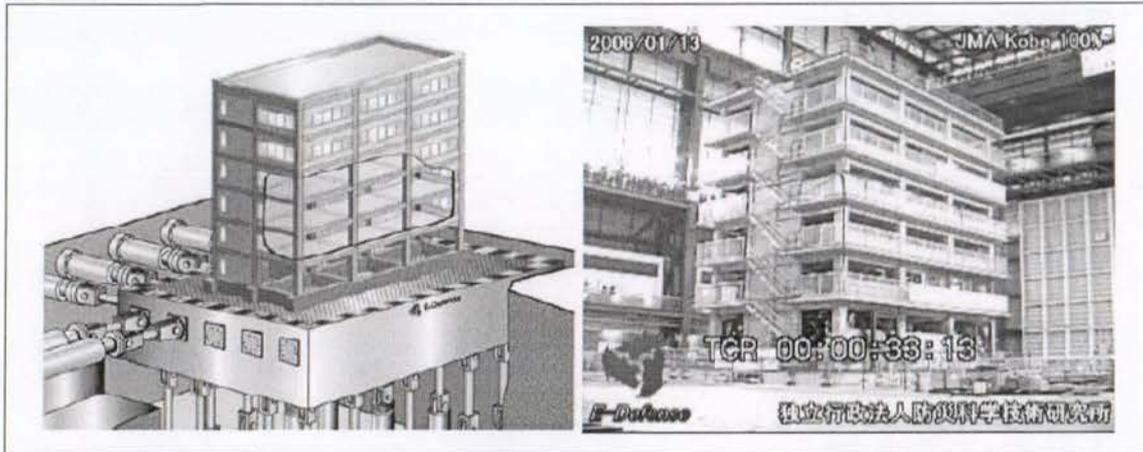
Figure 29. Overall view of the full scale RC structure used in E-Defense, (a) schematic view, (b) actual model (NIED (website) 2006)
