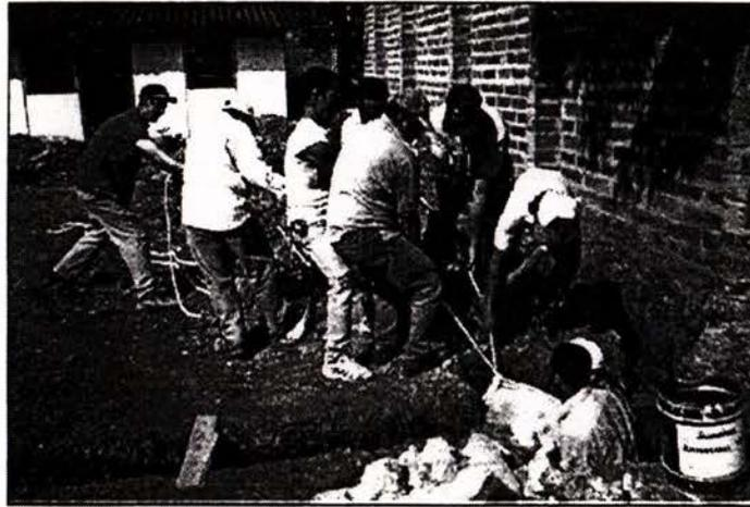
*Figure 2.6. A construction gang removes a large boulder from an excavation into rubbly debris-flow deposits (Q<sub>fm</sub>) near accelerograph station POL (P-18).*
