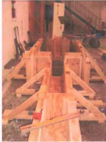
Figure 3.4-Formwork construction
