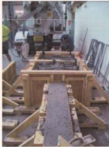
Figure 3.6-Pouring of concrete
