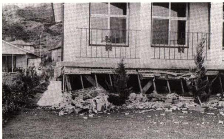
Figure 2-7 Jackstudded Sub-floor showing Cladding broken off and a slumping to one side (Source: Jennings and Housner 1971)
