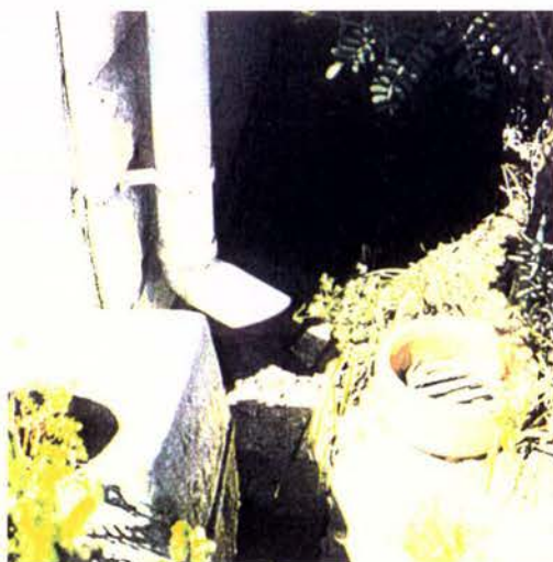
Figure 2-15 Slab on Ground showing relative sliding difference between the Dwelling and Ground; note the prior location of Services (Source: BRANZ 2003)
