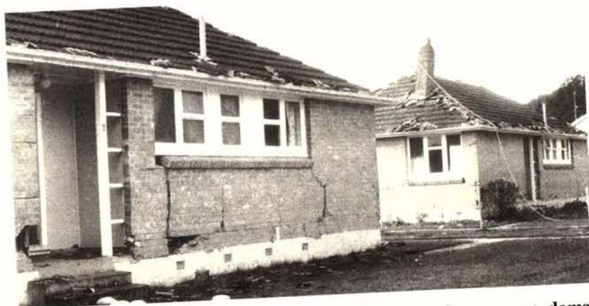
Figure 2-9 Superficial Damage to brick veneer on State Dwellings, however no damage to the Foundation Wall is evident (Source: Eiby 1980)
