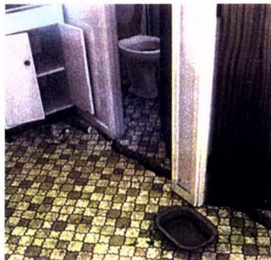
Figure 2-15 Slab on Ground showing relative sliding difference between the Dwelling and Ground; note the prior location of Services (Source: BRANZ 2003)
