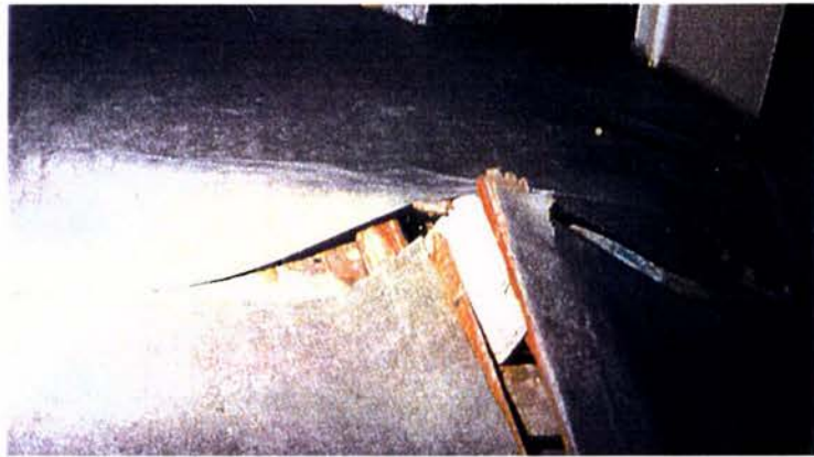
Figure 2-4 Example of Piles punching through the Floor due to Sub-floor Framing slipping off Piles (Source: BRANZ 2003)
