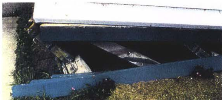
Figure 2-2 Corner of Foundation showing Piles swayed to one side (Source: BRANZ 2003)
