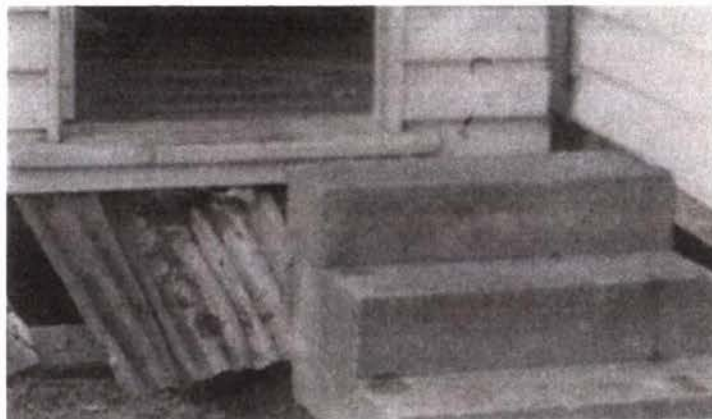
Figure 2-5 Full Piled Foundation slipped off Foundations, with Concrete steps remaining in place (Source: Cooney 1979)
