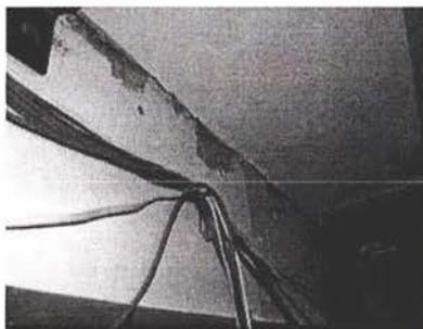
(b) Entire seat has been lost at the completion of the Phase I ( $-2.0\%$ )
