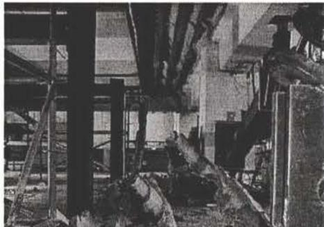
(a) Failure of the first hollowcore unit
