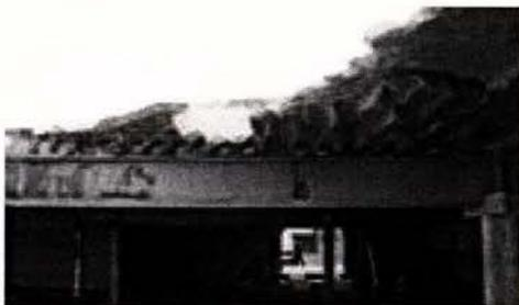
Figure 1 Photograph of precast hollow core floor collapse after the 1994 Northridge earthquake
