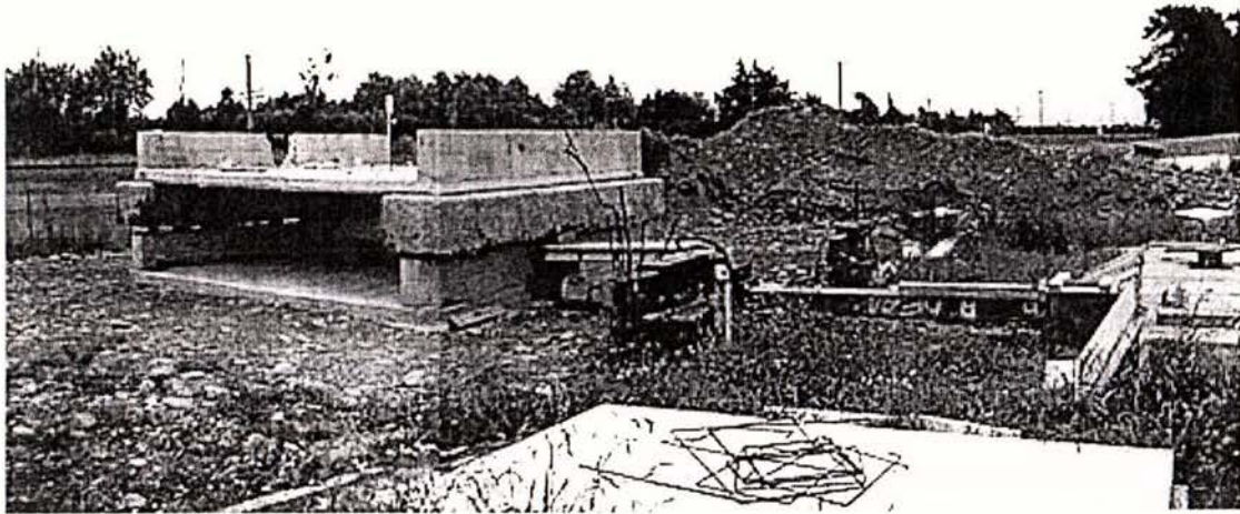
Figure 3.16. View of Test 3 with carcass of Test 1 placed on top.
