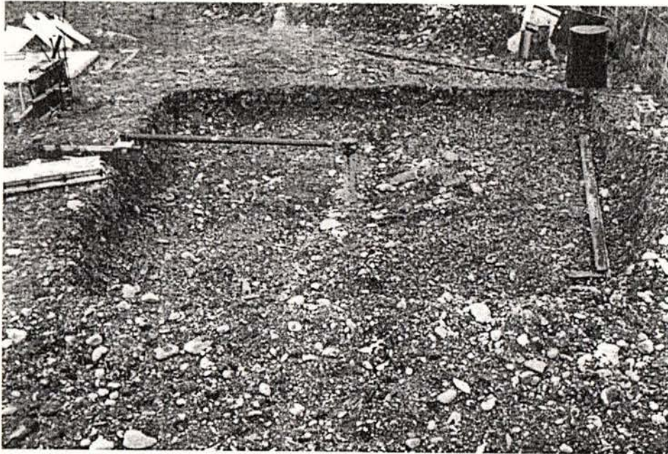
Figure 6.1. Steel pipe pile in place prior to construction of shallow foundation.
