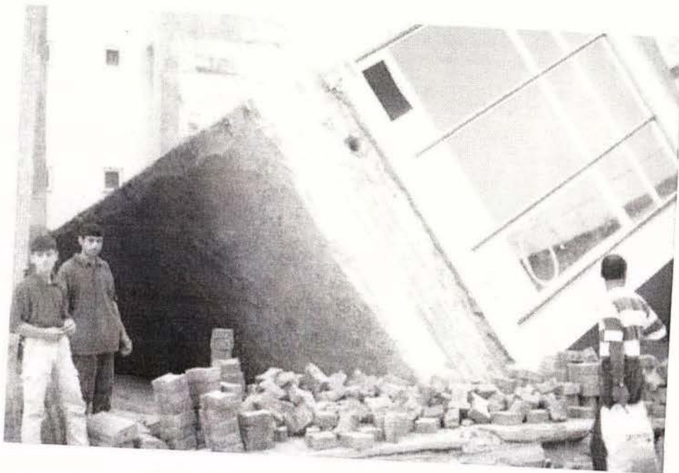
Figure 1. Overturned building in Adapazzari.
