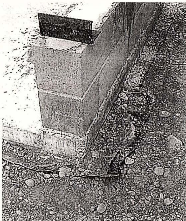
Figure 3.8. View of masonry wall built on top of slab and beam.
