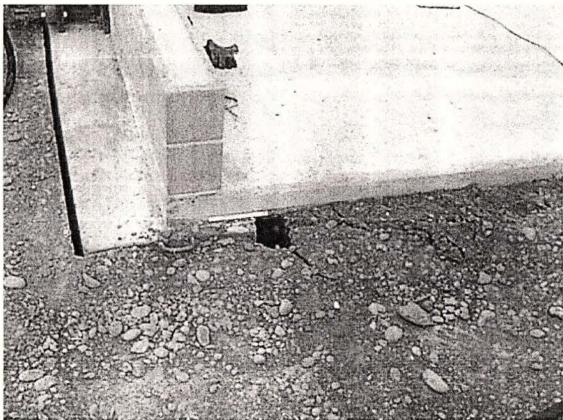
Figure 6.10. Gapping and passive wedge after completion of testing.
