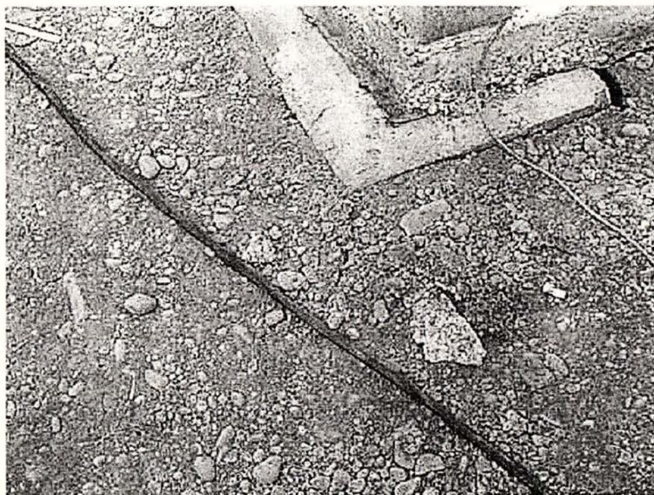
Figure 4.9. Soil cracking and heave in front of the test structure after load step 3.
