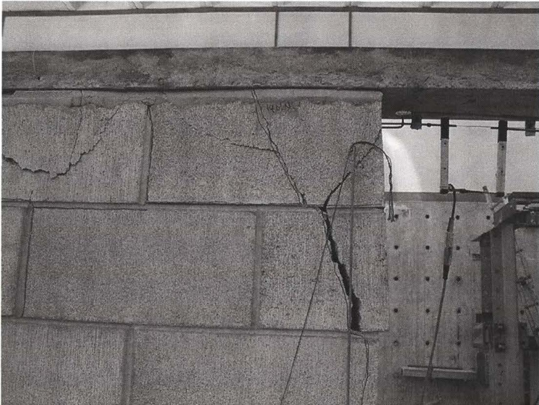
Figure A.7 Structural damage at bond beam causing significant steel channel-masonry wall slippage.
