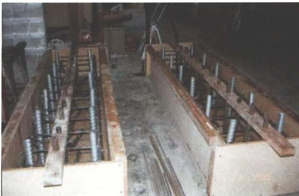
Photo 1 Footing reinforcement cages positioned in boxing.
