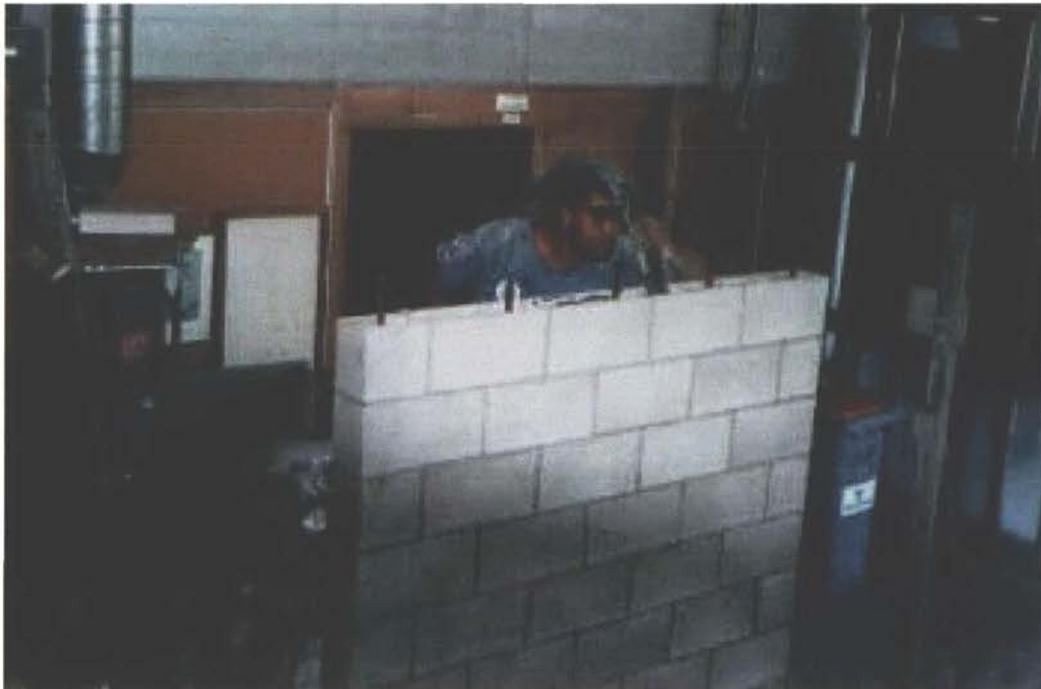
Photo 4 Masonry wall grouting.
