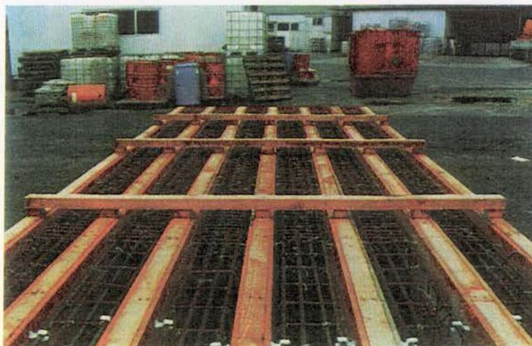
Figure 4-13 Reinforcement Cages Positioned in Boxing
