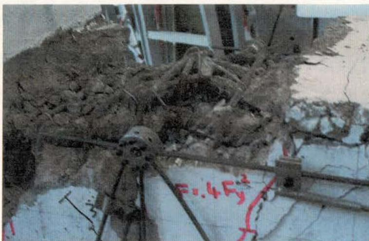
Figure C-9 Rupture of Longitudinal Bar
