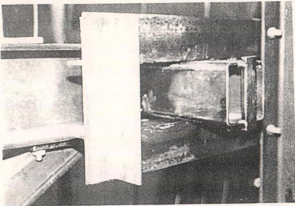
(c) Connection of support beam to column 2
