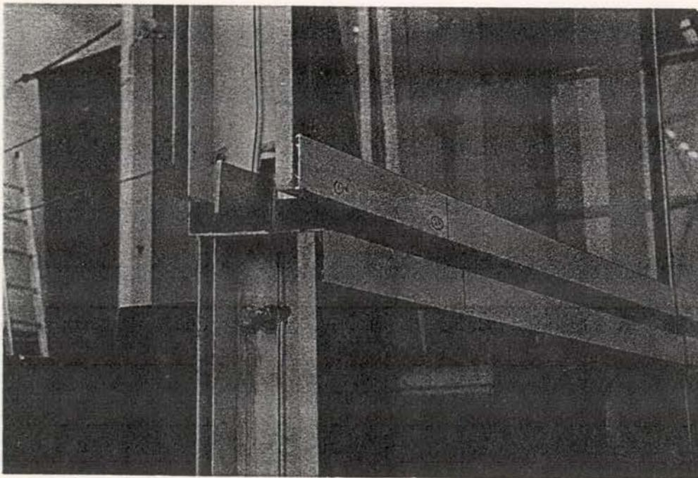
Figure A4 Method for preventing panel misalignment
