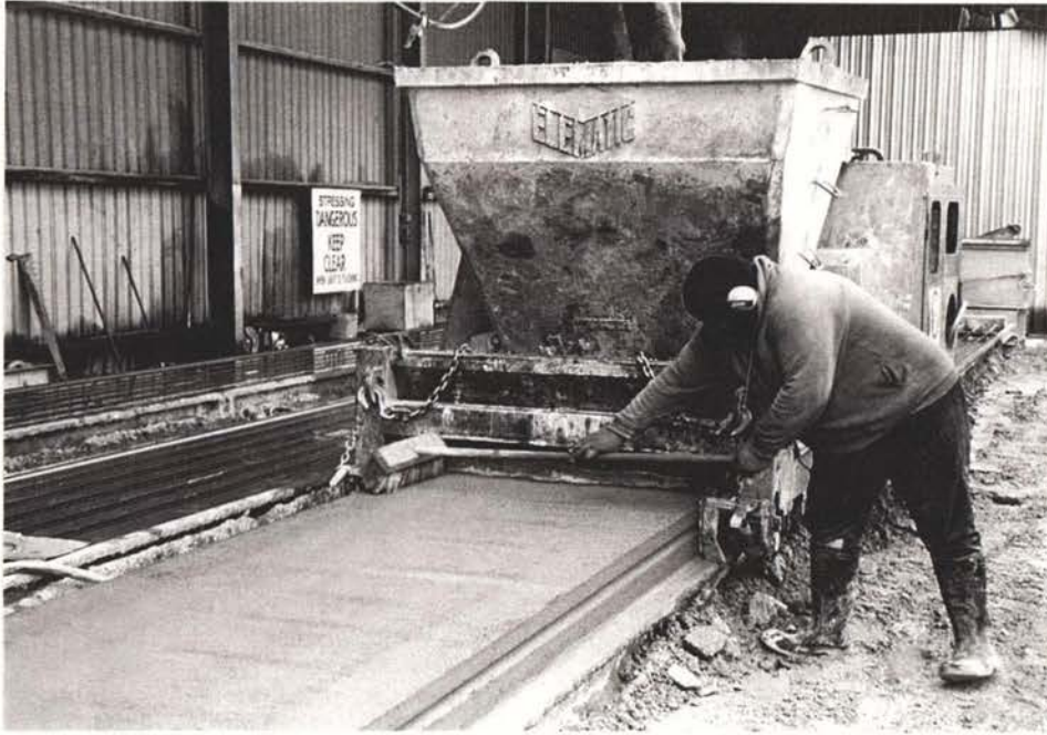
Fig. 1.14 Brooming of an extruded hollow core surface
