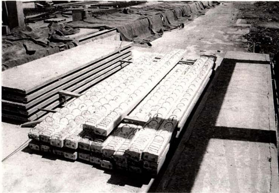
Fig. 1.5 Manufacture of pretensioned joist units (Interspan)
