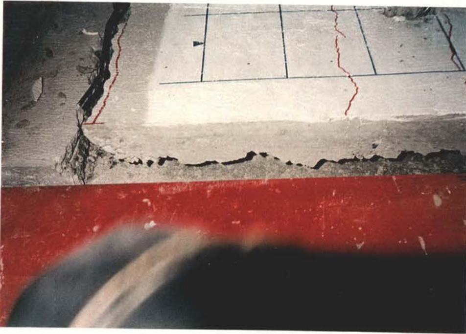
Fig. 3.24 Topping separation caused by downward dislocation of the hollow core unit
