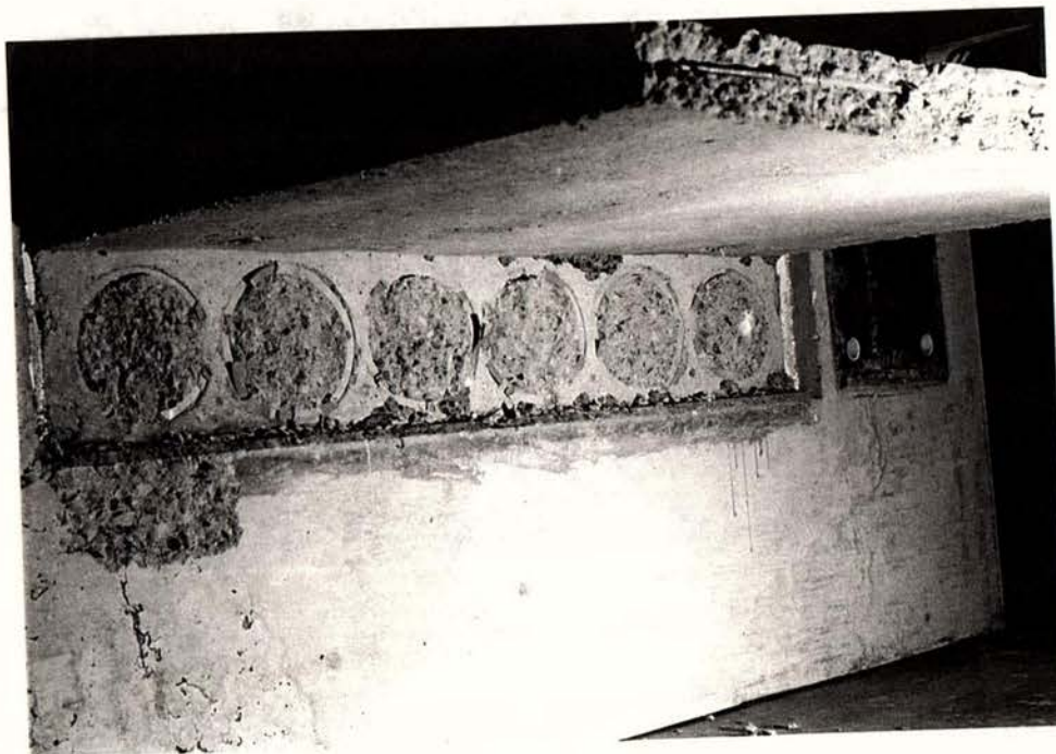
Fig. 3.68 View of support block after removal of hollow core section. Note smooth soffit of cantilevered topping slab
