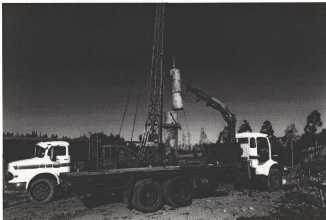
Figure 12. Preparing to drive the casing.
