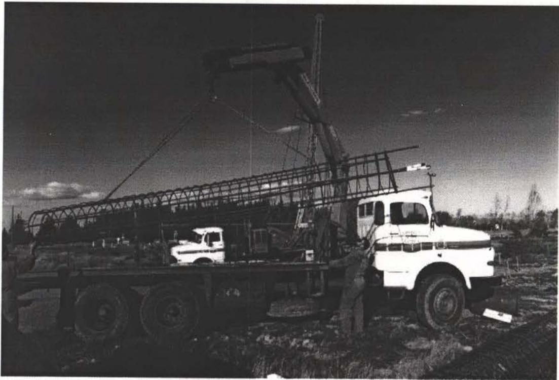
Figure 13. Unloading the reinforcing cage.
