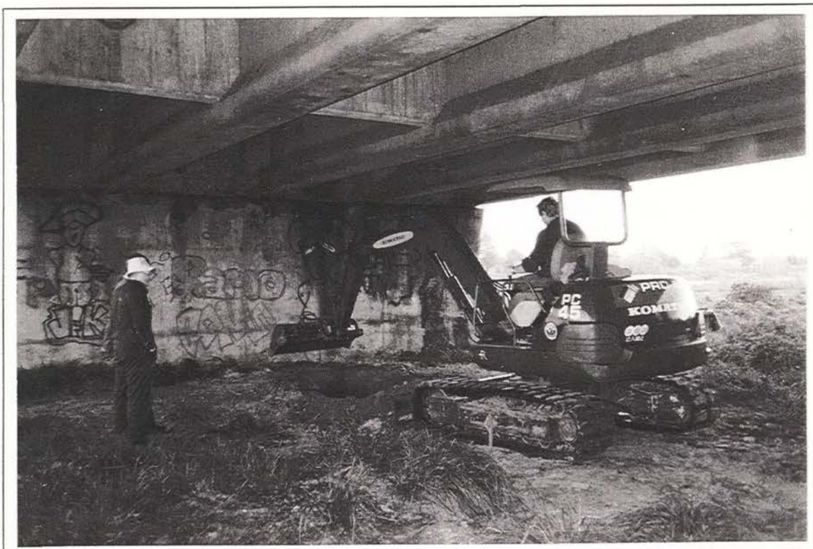
Figure 4.5 Start of excavation at Pier C
