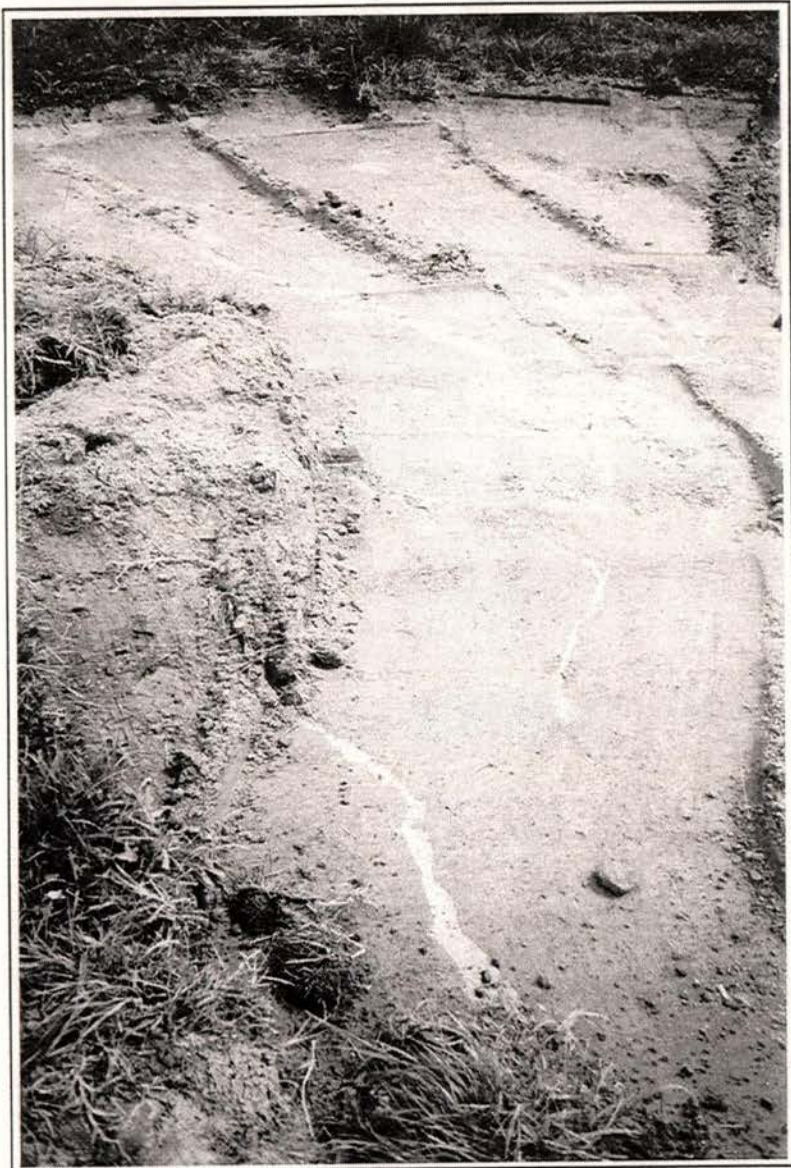
Figure 4.14 Sand Filled Lateral Spread Cracks South of Trench 1
