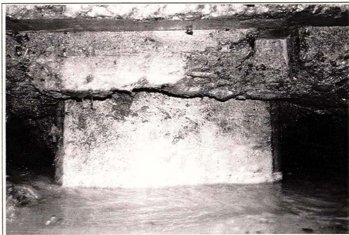
Figure 4.11 Riverside view of the top of pile 3
