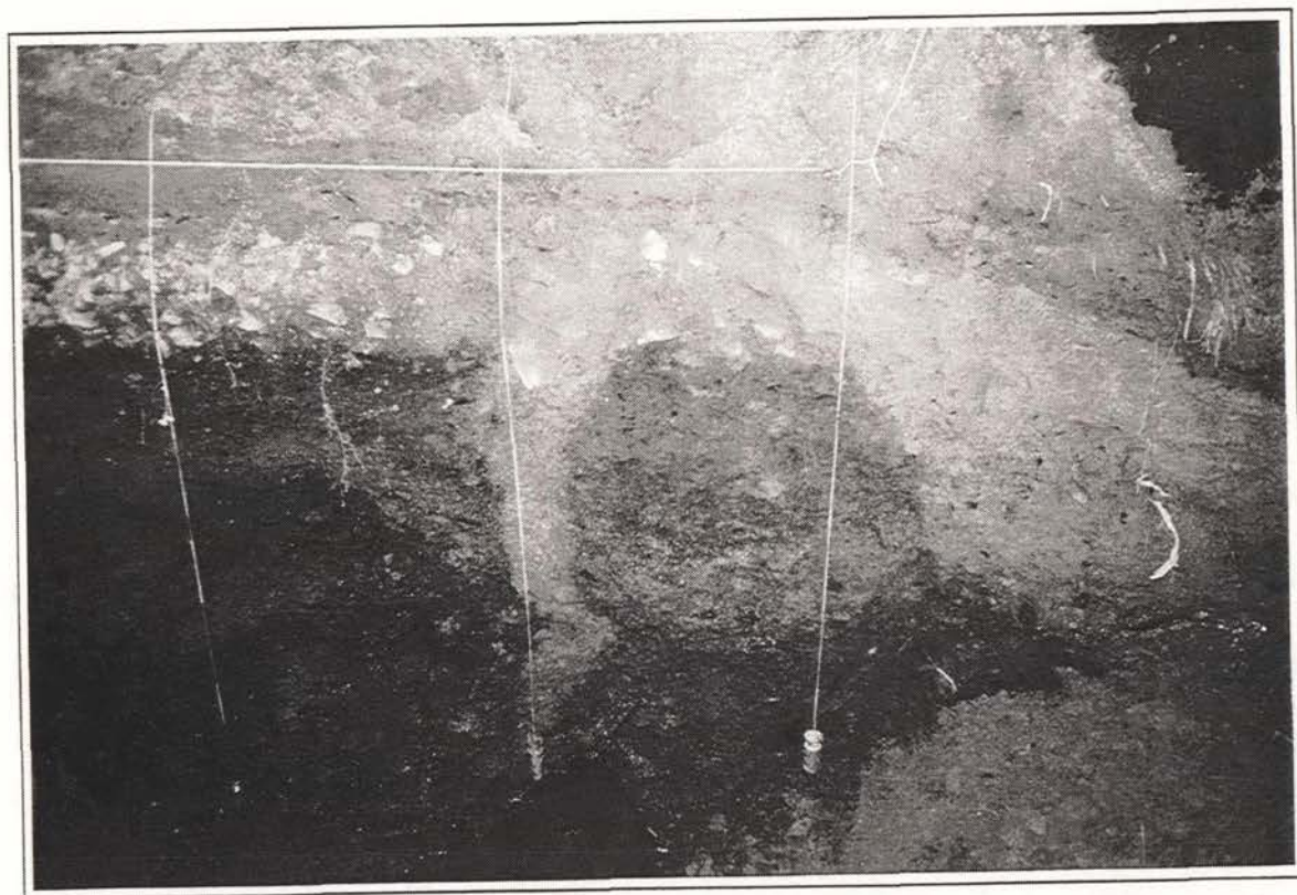
Figure 4.9 Lateral spread crack about 2.5 m from the river side of Pier C
