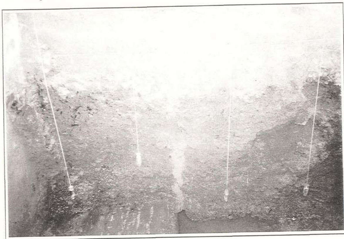
Figure 4.8 Lateral spread crack near the river side of Pier C
