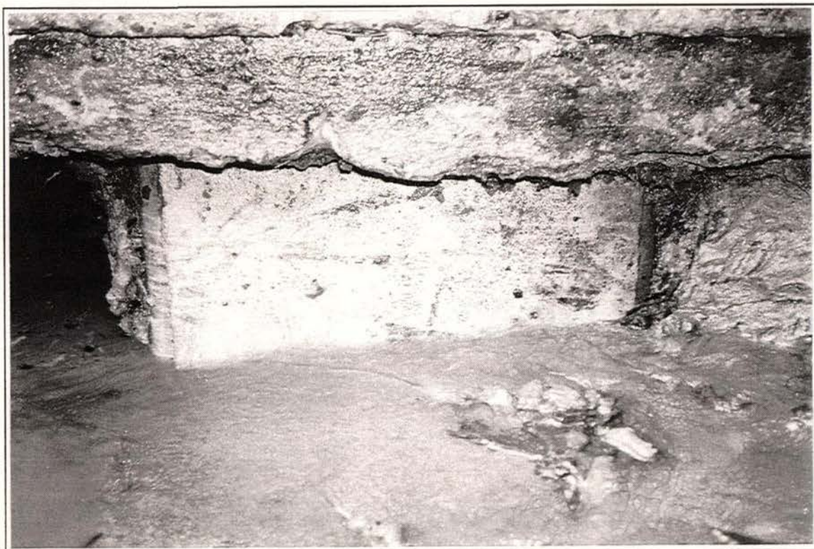
Figure 4.12 Riverside view of the top of pile 4
