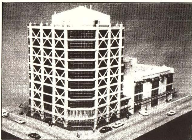
Figure 4.7 Base isolation has been used in the new Wellington District Police Headquarters and Central Police Station. The base isolation combines three components: long flexible piles standing within oversize casings; special spherical bearings at the pile tops; and lead extrusion dampers. Architects: Works Corporation
