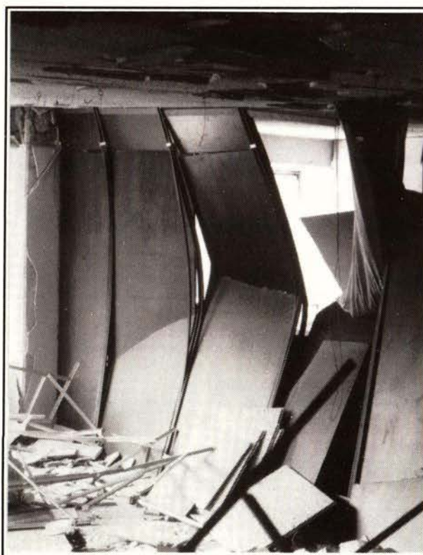
Figure 1.1 Damage to partitions and ceilings in DDF Water Supply Secretariat, Mexico City. September 1985.
