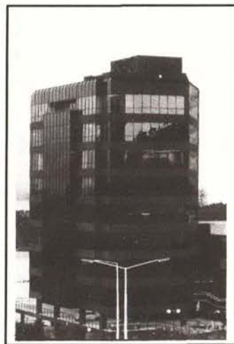
Figure 4.6 NEC House in Grafton Road, Auckland uses a combination reinforced concrete shear walls and beam/column frames. It is typical of many medium rise office build- ings erected in the 1980s. Seismic move- ment was allowed for in both the curtain wall and precast concrete spandrels. Architects: KRTA Ltd.
