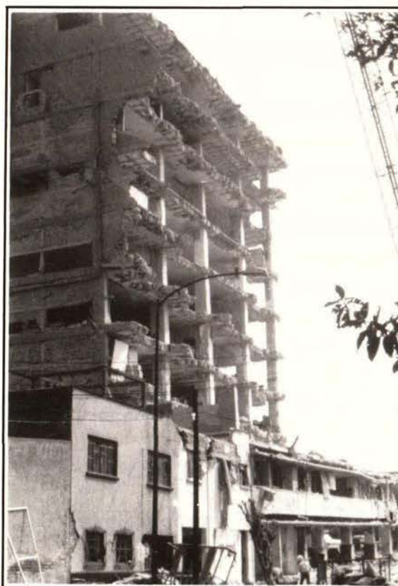
Figure 2.1 Secretariat of water supply, Mexico City, after collapse of the top 8 storeys of the first bay adjoining street facades.
