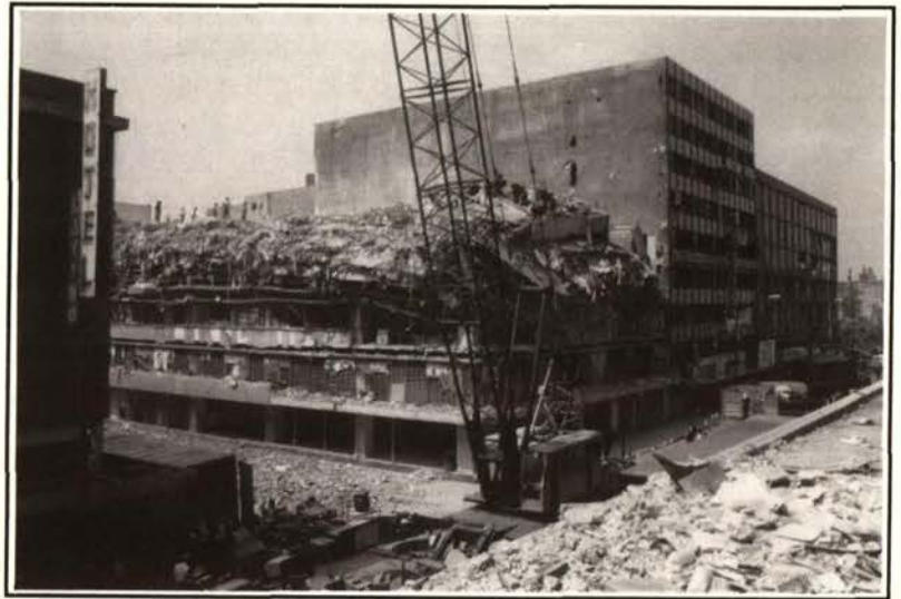
Figure 3.6 Pancake collapse of a manufacturing building in Mexico City because the columns did not match the requirement for ductile behaviour.
