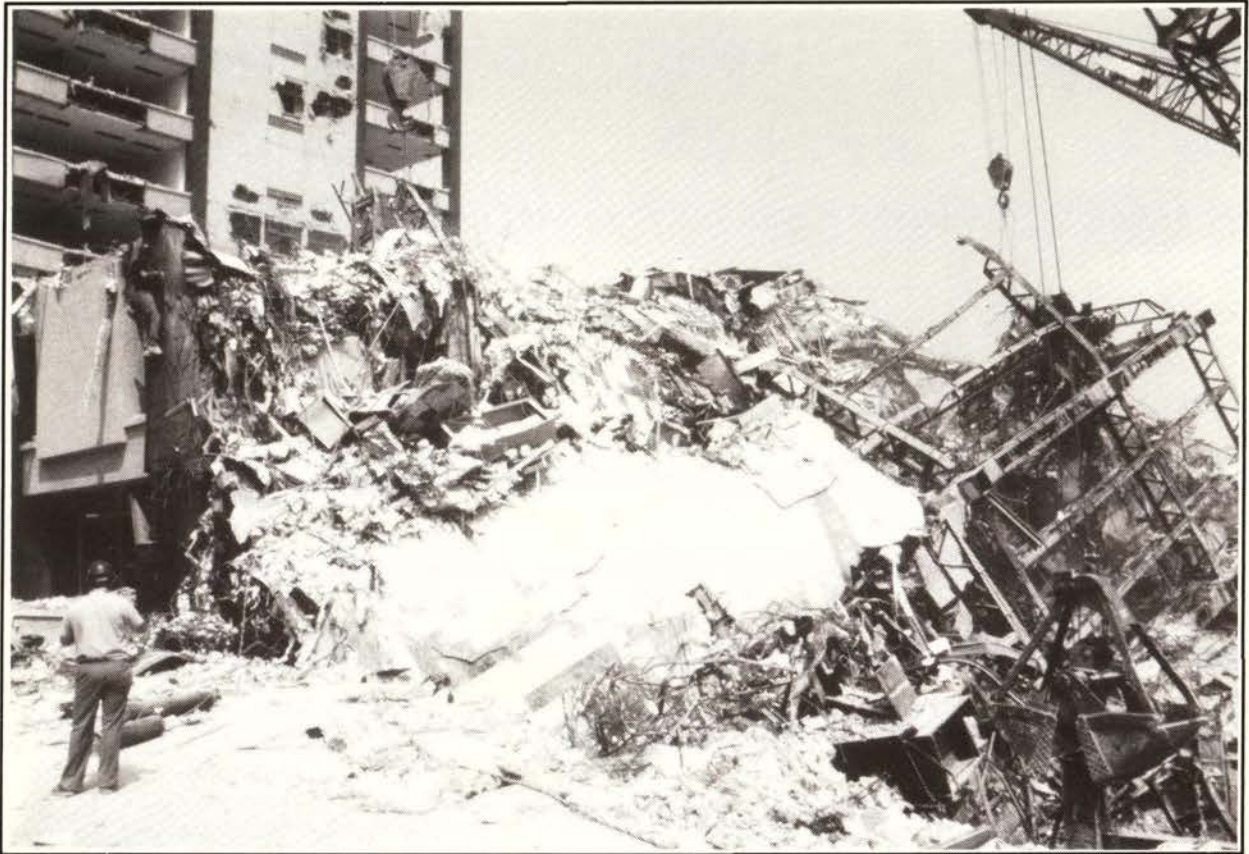
Figure 1.7 Total collapse of two steel-framed high-rise buildings (14 and 22 storeys) in the Mexico City earthquake Sept 1985.
