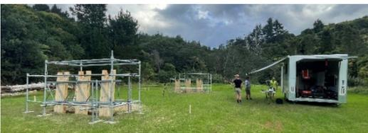
*Figure 2. Stage 01 showing the two sets of poupou hung from scaffolding and awaiting the concrete to be poured into the footings. Note: the field trailer to the right. Image: Anthony Hōete.*
