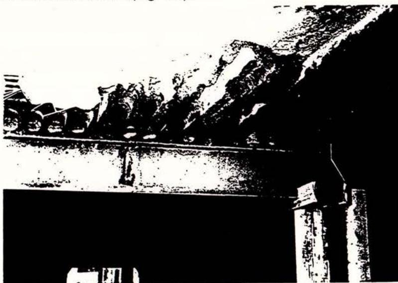
**Fig 1.1: Hollow Core floor failure exhibiting fracture of web elements
