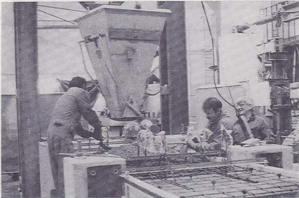
Fig. 3.9e Pouring of Cast-in-Place Topping Concrete Specimen 1
