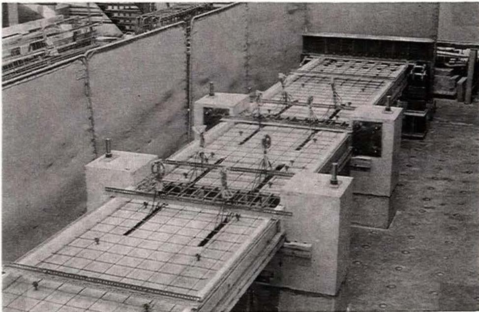
Fig. 3.9d Wire Mesh Placed Above the Units
