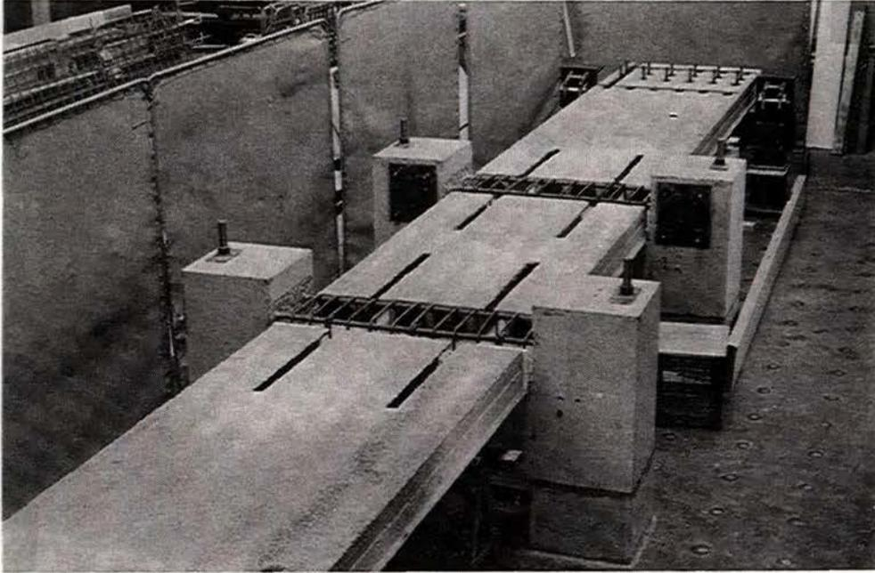
Fig. 3.9c Dy-core Units with Top Flange of the Voids Broken Back to Anchor Tie Bars
