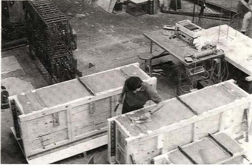
Fig. 3.9a Pouring of Supports
