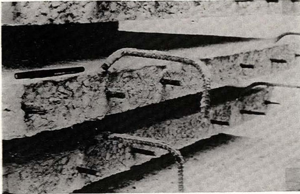
Fig. 1.2 Hanger Bars for Precast Concrete Floor Units According to the New Zealand Guidelines [1]
