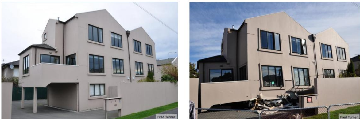
Figure 14. Soft storey collapse of ground floor observed in the canterbury earthquake sequence.
