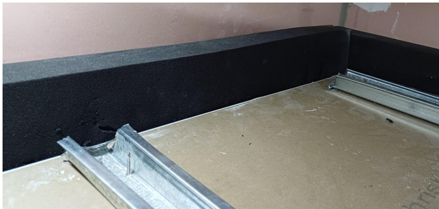
Figure 4.10. Photo of edge of fully floating ceiling with isolation foam
