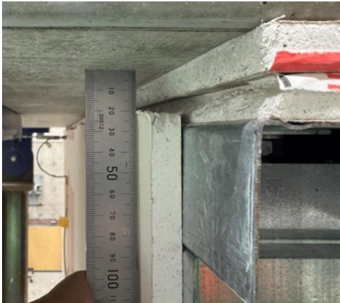
a) 20 mm - at Steel NW-Outside Wall
