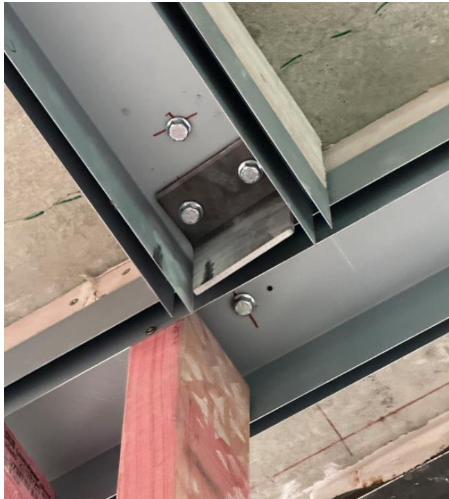
Figure 4.5. Steel angle at the wall T-junction
