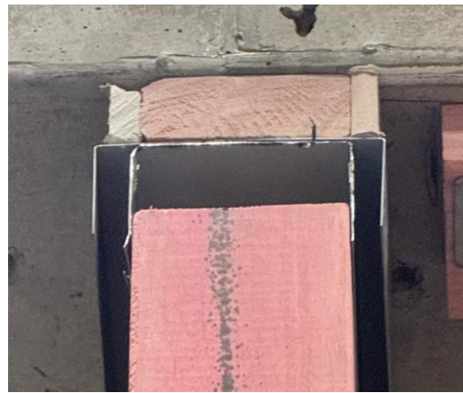
d) Photo at top of South out-of-plane wall
