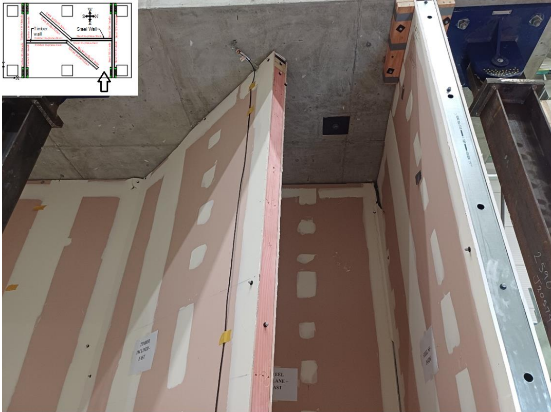
Figure 2.68. Walls from East direction after motion 18 - 3 % inter-storey drift
