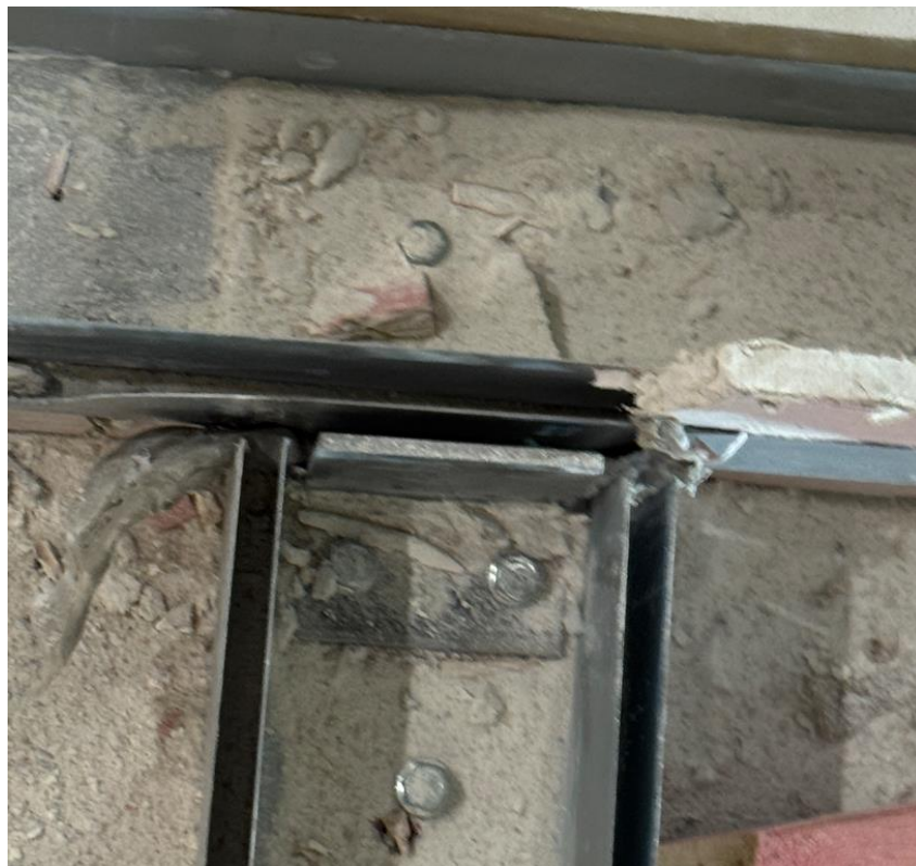
Figure 4.69. Photo of bottom steel angle at South wall junction taken during demolition
