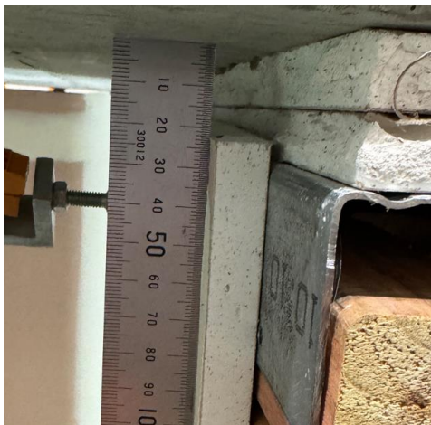
c) 22 mm - at Timber SW-Inside Wall
