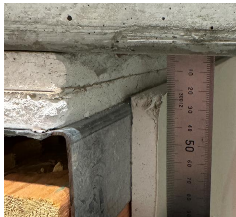
d) 22 mm - at Timber SW-Outside Wall
