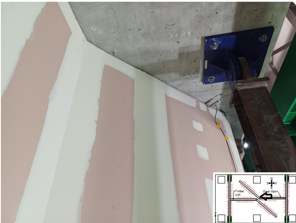
Figure 2.59. Steel wall West inclined junction after motion 18 - 3 % inter-storey drift
