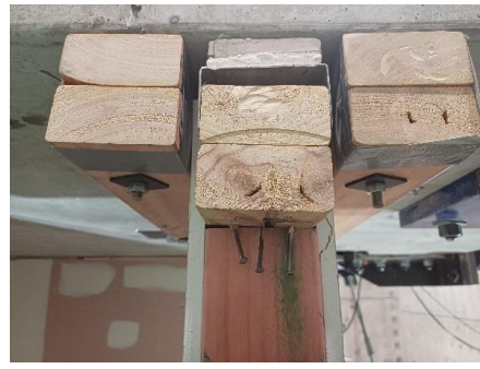
b) Timber South-West wall
