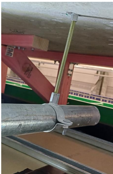
a) Pipe supported by M10 threaded hanger rod
