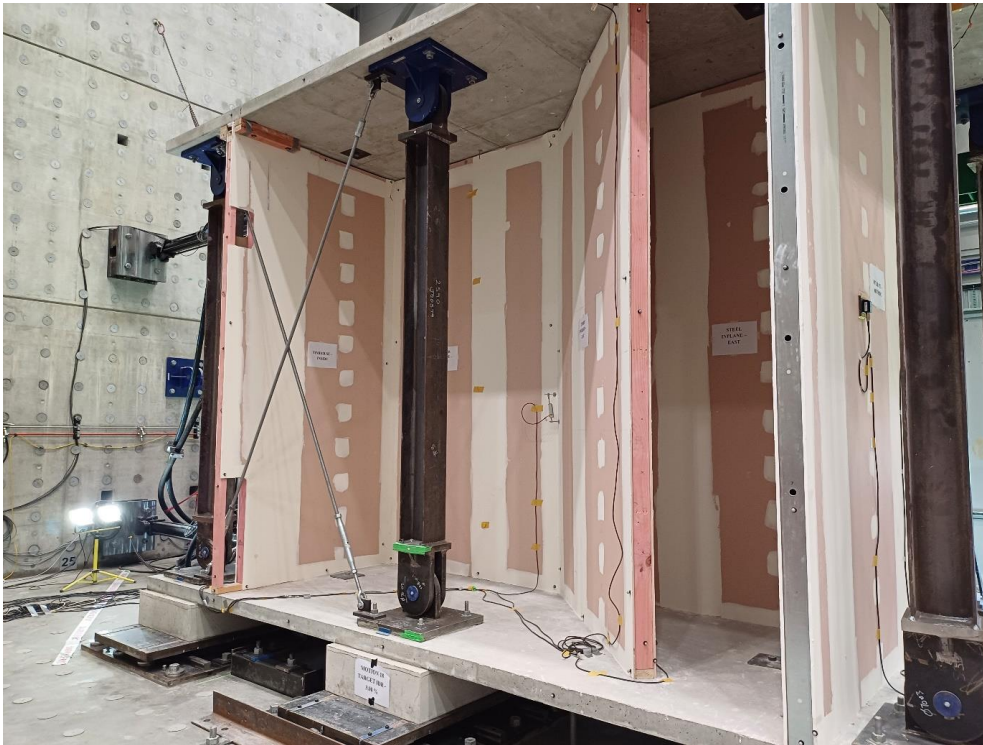
Figure 2.56. Wall specimen after motion 18 - 3 % inter-storey drift (North-East elevation)
