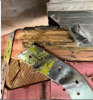
Timber wall SW/SE and Timber in-plane wall junctions and where there were nails securing the strap
