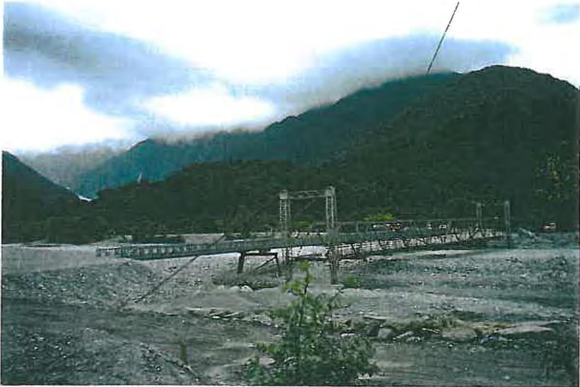
**Figure 8.8** - The Waiho River at Franz Josef which has had a history of flooding and aggradation. The old bridge has had to be cut and lifted to maintain the waterway while a new temporary bridge has been put in immediately upstream for SH 6. This type of aggradation is likely in many other rivers draining the Southern Alps following an Alpine Fault earthquake.
