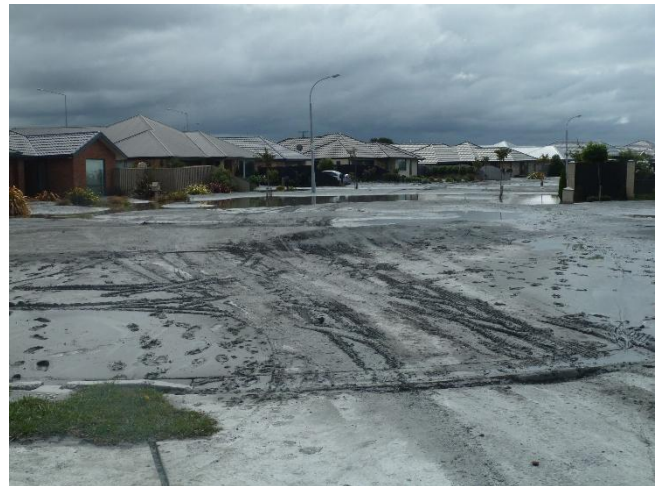
Liquefaction damage in Christchurch, 2011
