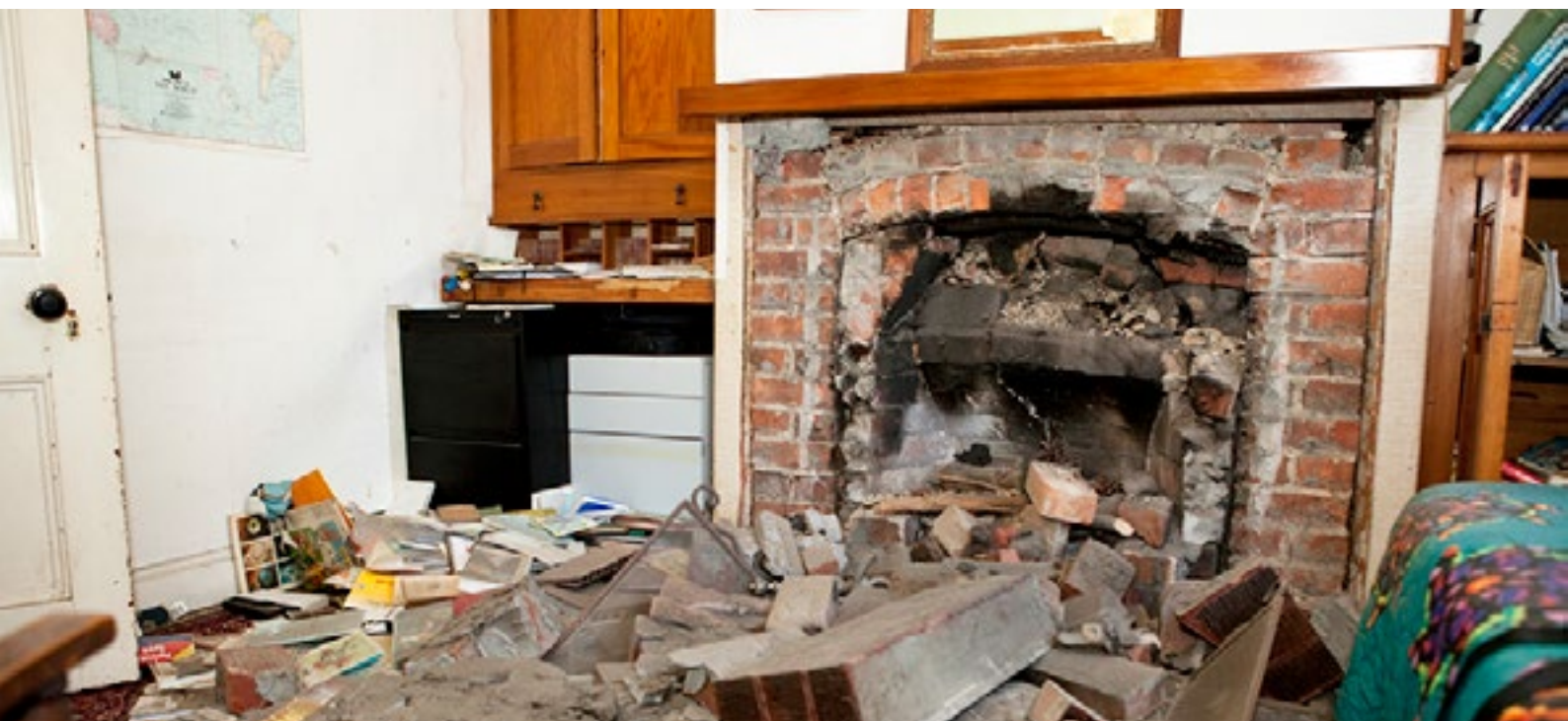
Chimney damage from the 2013 Seddon earthquake
